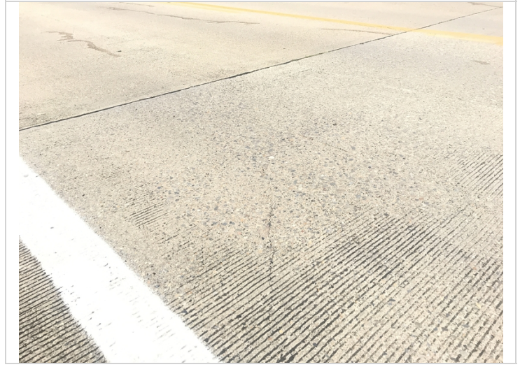
Cracking some sealed some not sealed
