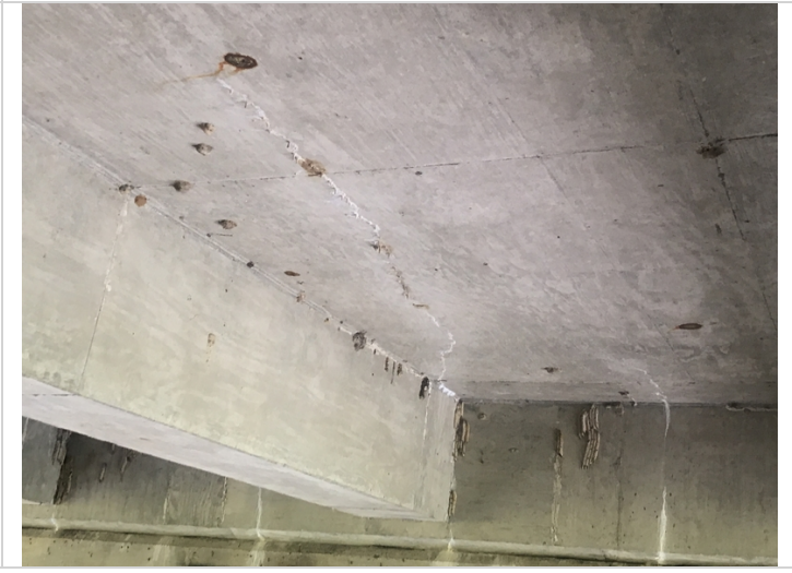
Span 4 photo of efflorescence
