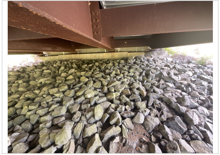
6/23 abutment photo of abutment 1 with riprap
