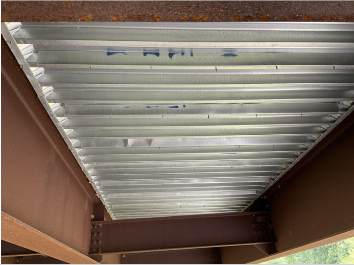
6/23 typical deck pans bottom side deck
