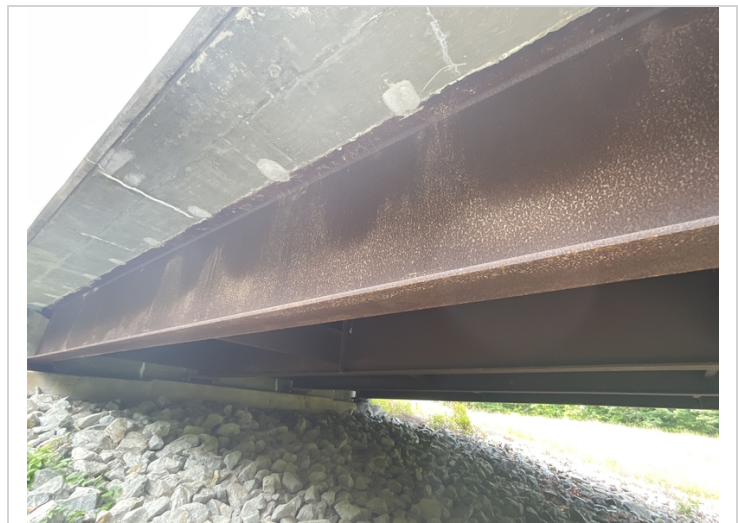
Span 1 beams 2,3&4 has a light color to weathering beams
