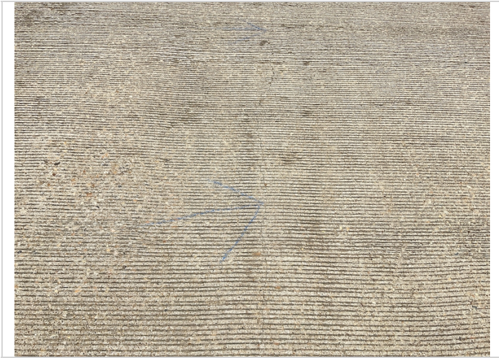
6/23 cracking in concrete deck
