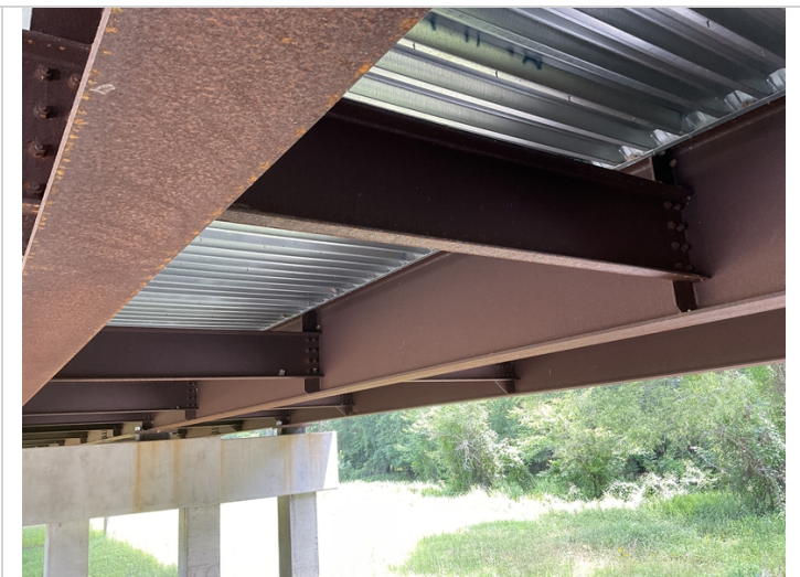
6/23 photo of weathering steel beams
