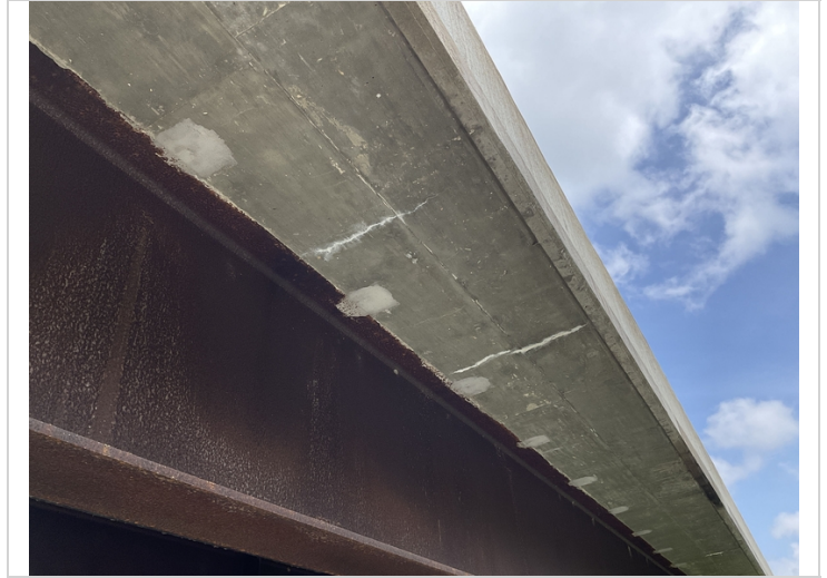
Typical efflorescence on over hangs
