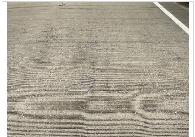
6/23 cracking in the deck mid span
