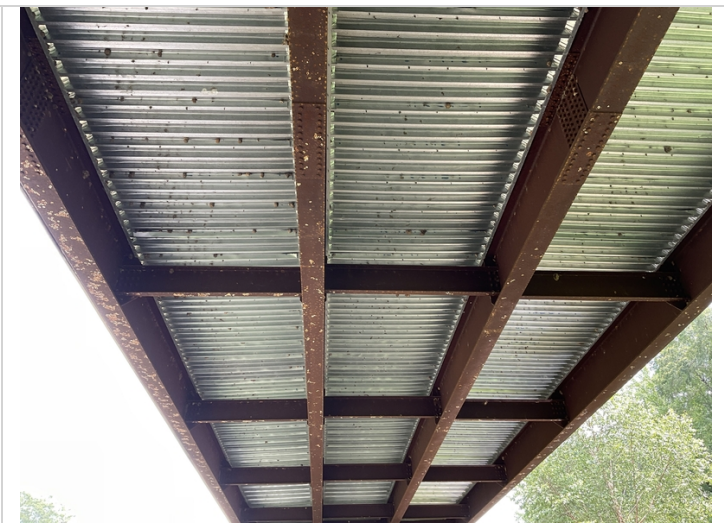
Photo of weathering steel beams over water span 5
