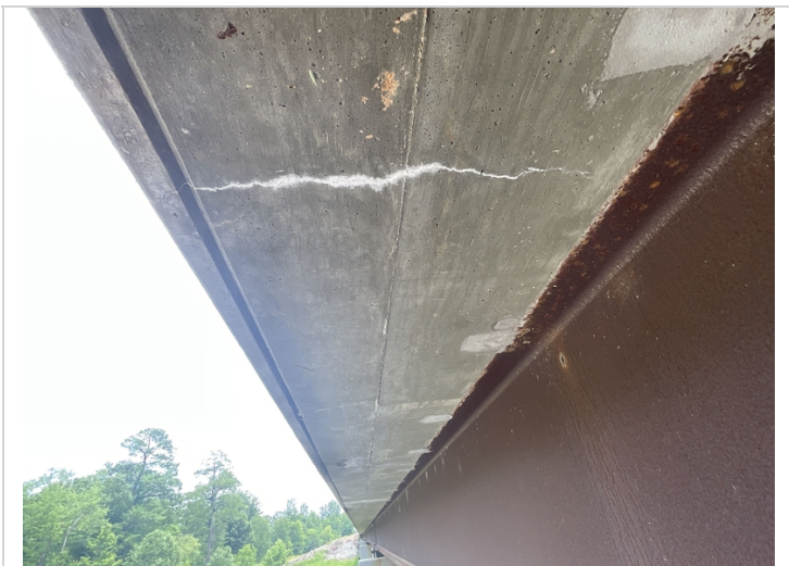
6/23 typical efflorescence on overhangs right and left side of bridge deck
