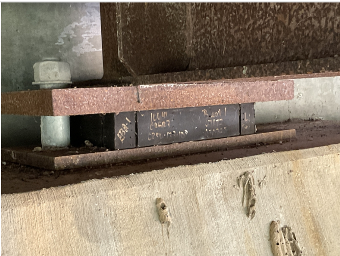
Photo of elastomeric bearing at beam 2 bent 1
