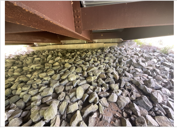
6/23 abutment photo of abutment 1 with riprap
