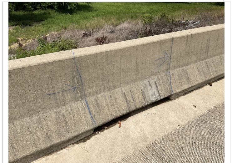
6/23 cracking in parapet wall right and left side.
