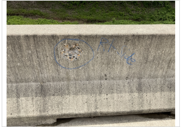
6/23 spall in concrete parapet wall Right side near end of bridge.
