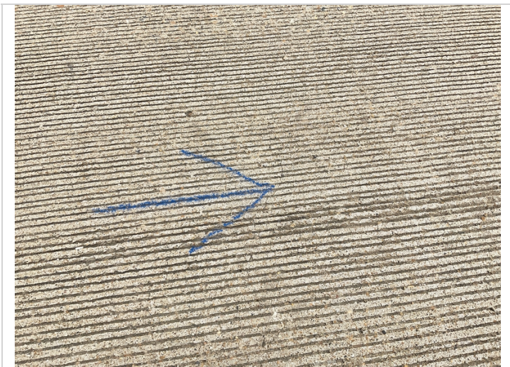
6/23 cracking in deck top side
