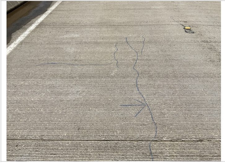
6/23 cracking in deck photo taken near end of bridge.
