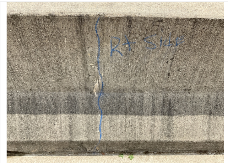
6/23Cracking with efflorescence in concrete parapet wall right and left sides.
