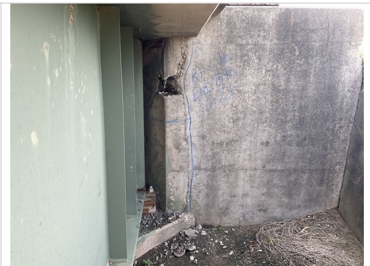
Bent 6 right side large spall with rebar exposed
