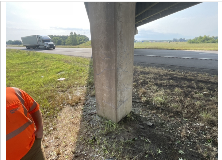
Column 1 bent 2 has cracking and delam
