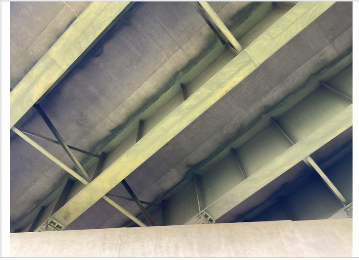
Beams chalking and oxide build up in various locations
