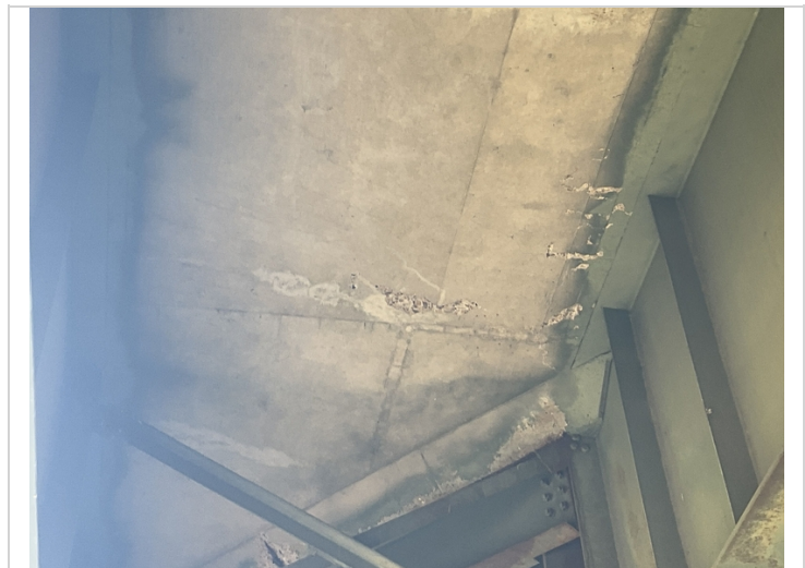
Span 1 bay 1 has spalls
