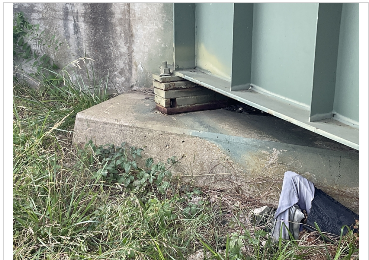
All Fixed bearings are showing signs of rusting
