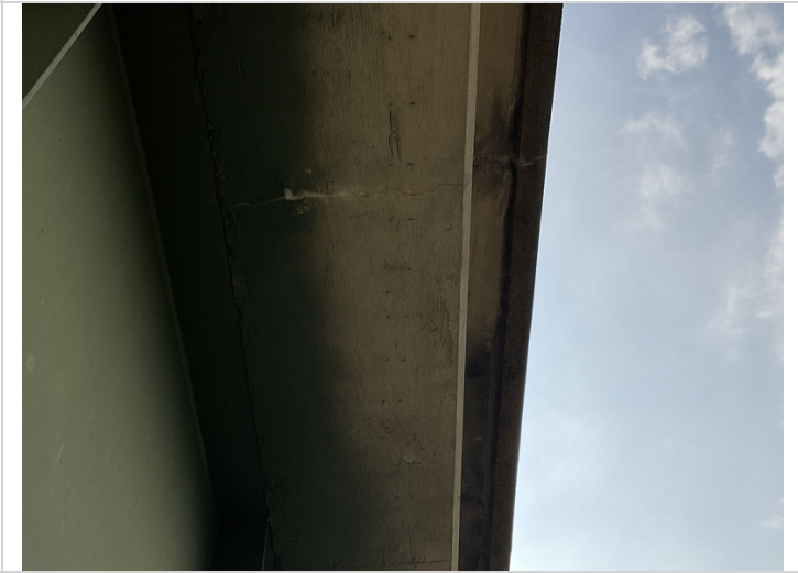
Deck over hangs have cracking and efflorescence in various locations
