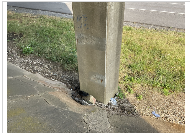
Old patch work bent 5 column 1
