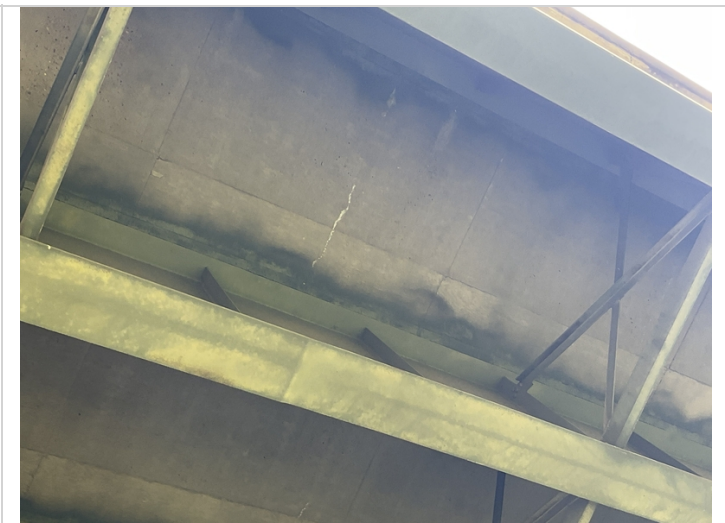
Span 3 efflorescence bay 5
