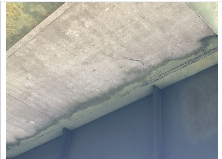
Span 1 bay 5 has spall
