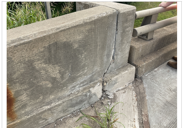
Walls beginning of bridge left and right side have delams before first joint on bridge
