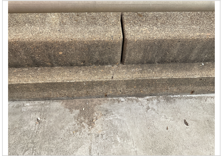
Cracking in concrete bridge railing
