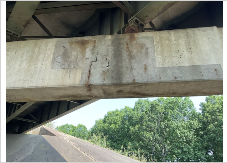
Bent 2 cap old patchwork is failing and popping out
