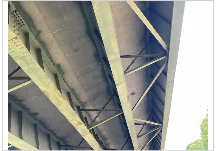
Span 2 bays 1 & 2 have spalls
