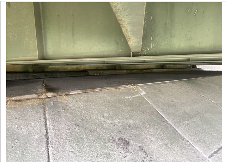
All fixed bearings are beginning to rust
