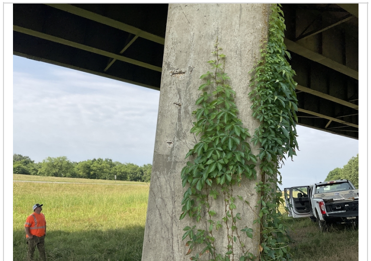
Bent 3 column 1 rebar exposed
