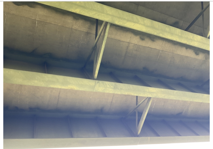
Span 3 efflorescence in various locations
