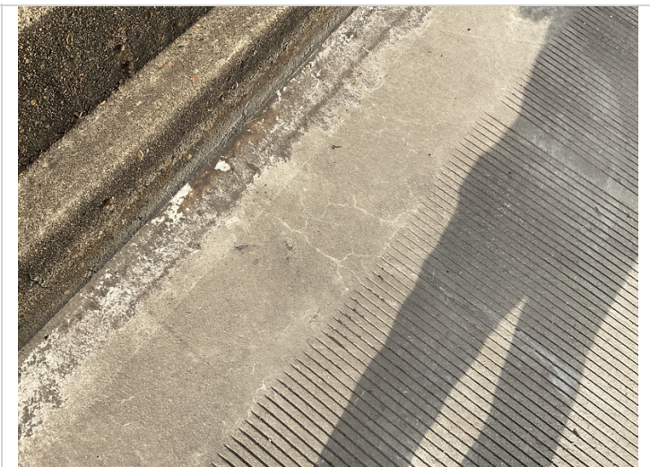
Map like cracking in various locations on deck
