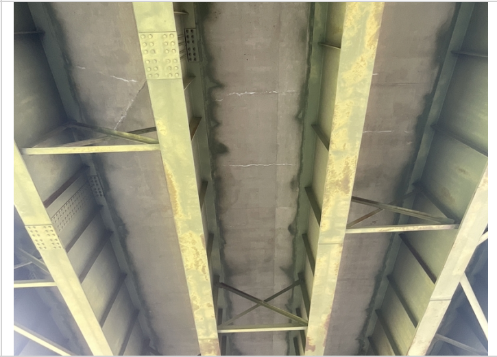
Span 2 efflorescence in various locations
