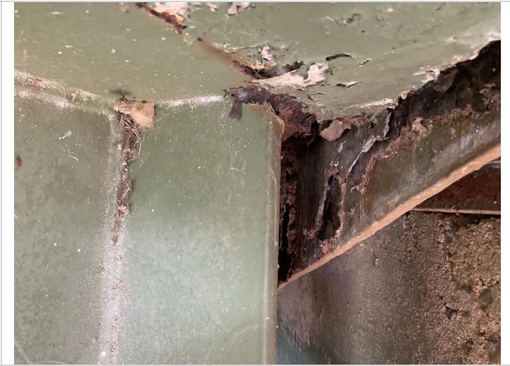
Beginning of bridge beam 1 has corrosion with section loss
