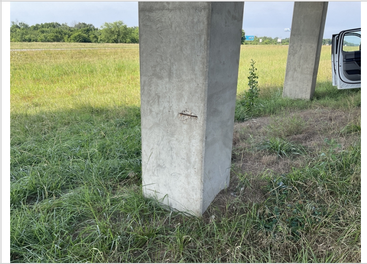
Bent 3 column 2 rebar exposed
