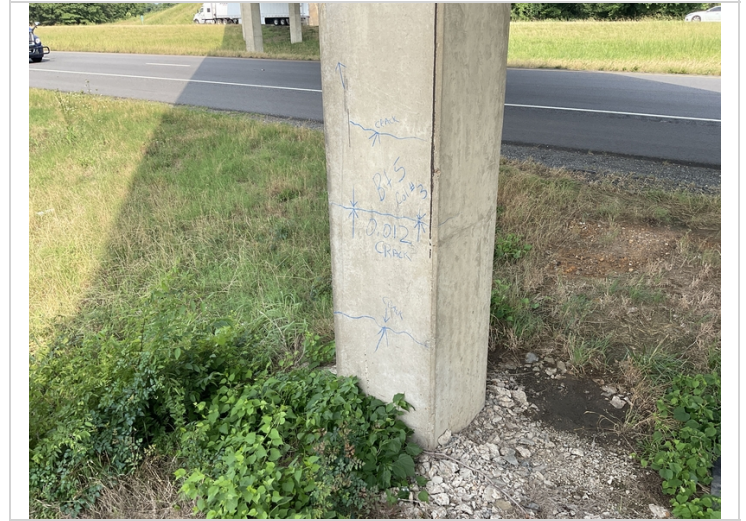
Cracking in bent 5 column 3
