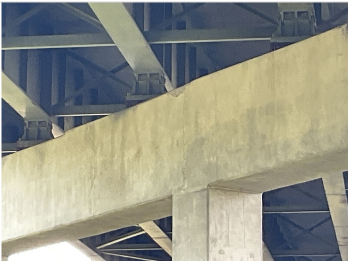
Delam bent 4 span 3 side on cap
