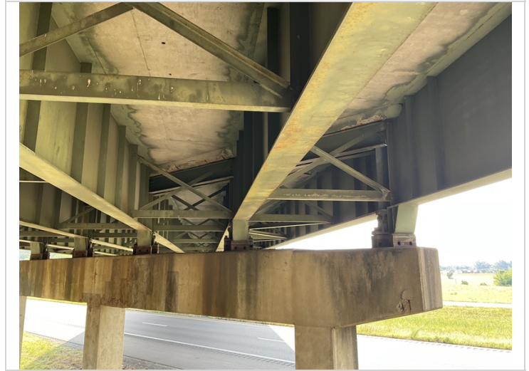
Most honches have spalls some with rebar exposed
