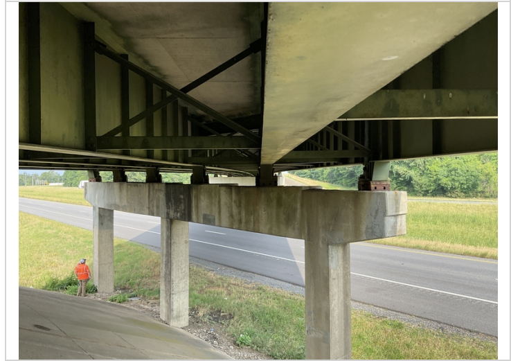
All movable bearings are showing corrosion
