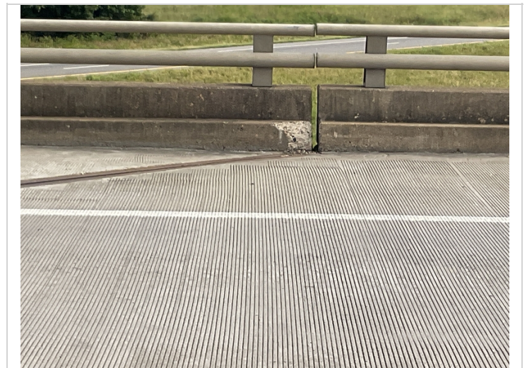
Span 4 left side of concrete railing above bent 5 spall
