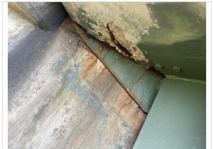
Beginning of bridge right side deck over hang has rebar exposed
