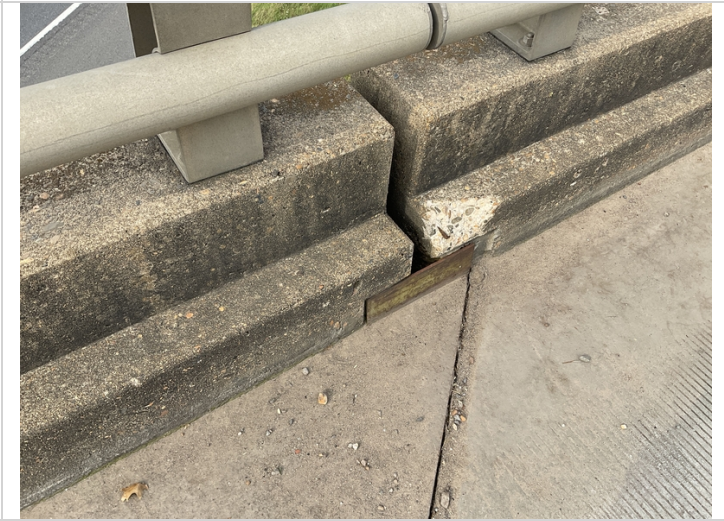
Delam Rt side end of span 1
