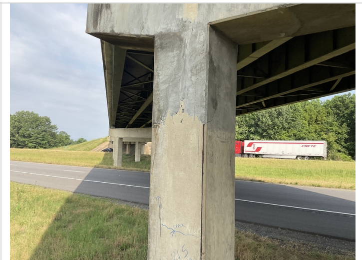
Old patch work bent 5 column 3
