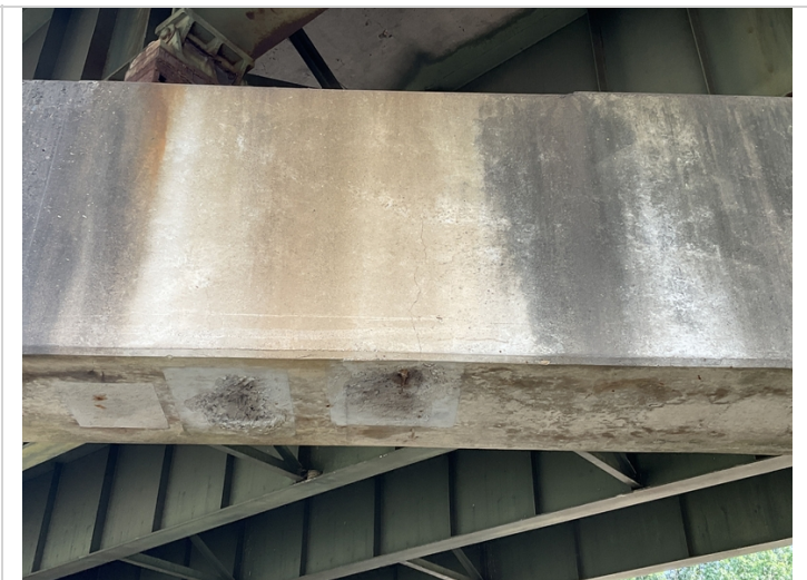
Cracking in bent 2 cap
