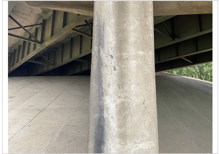
Delams with wire showing bent 2 column 3
