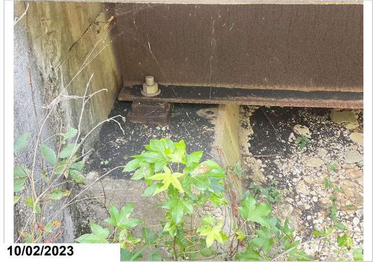
Bent 1 photo of sand blasting material left on cap from joint repair.
