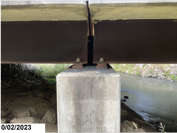
Typical bearings photo
