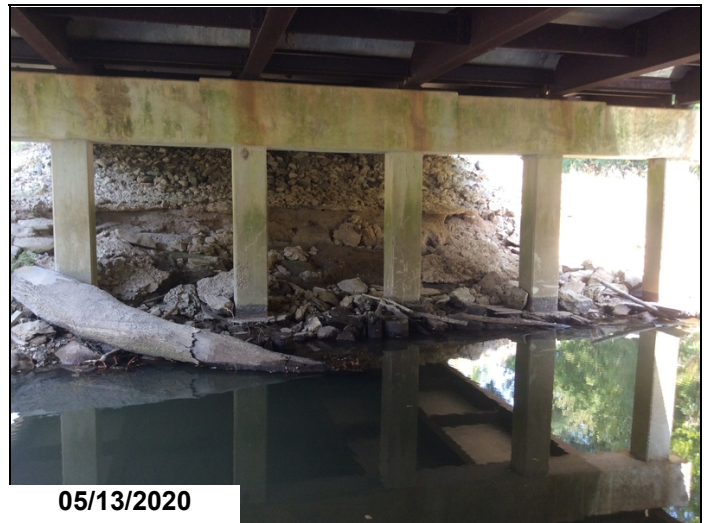
EROSION AT END BENT SLOPE
