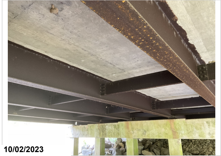
Typical superstructure photo with weathering steel beams
