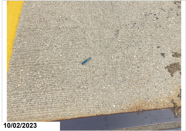
Span 1 minor cracking in top of deck
