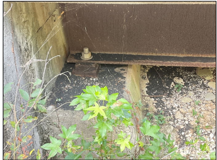
Bent 1 photo of sand blasting material left on cap from joint repair.
