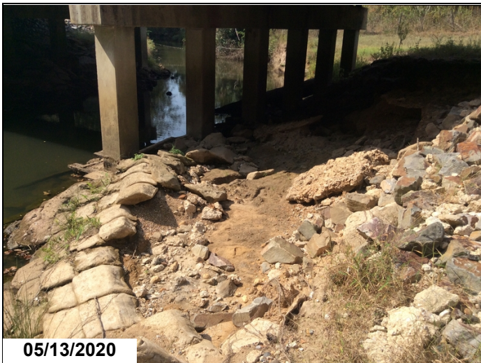
BENT 2 AND 3. MATERIAL HAS WASHED AWAY FROM COLUMNS. This photo of BT 3
