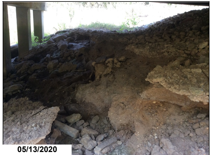
BENT 2 AND 3. MATERIAL HAS WASHED AWAY FROM COLUMNS.
