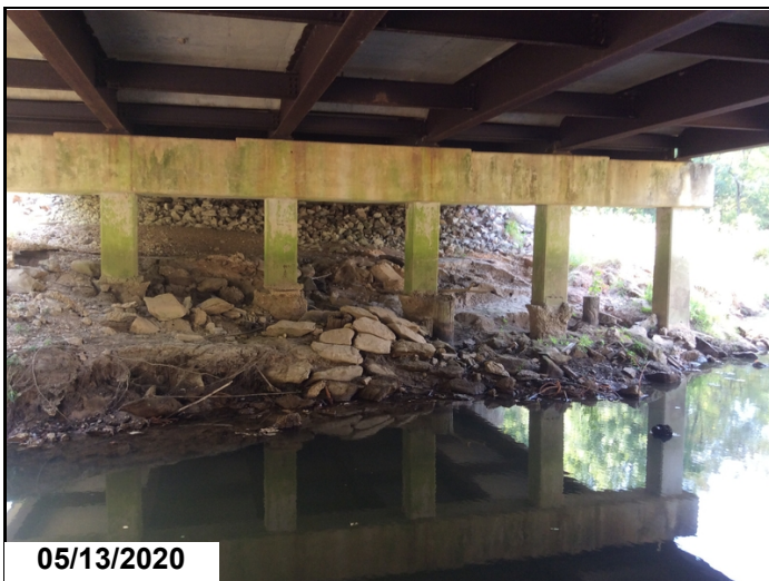
Bent 2 erosion
