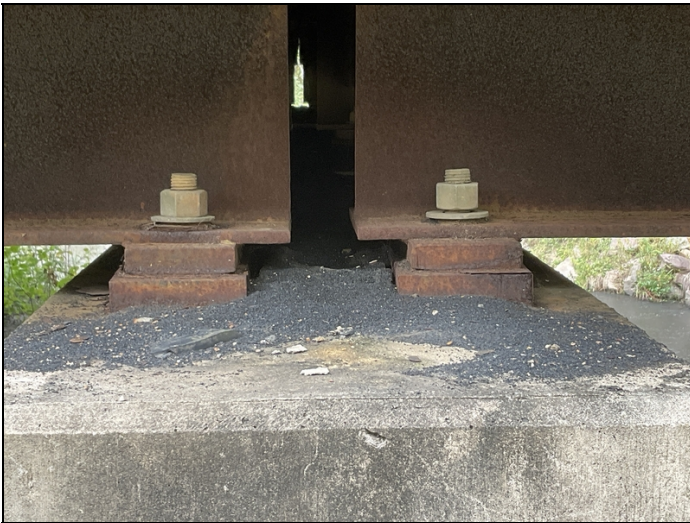
Bent 2 cap need cleaned
