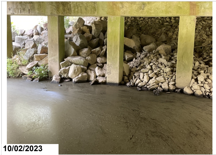
Bent 3 pile 3 honeycomb area at ground line
