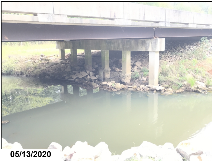
Erosion Bent #2
