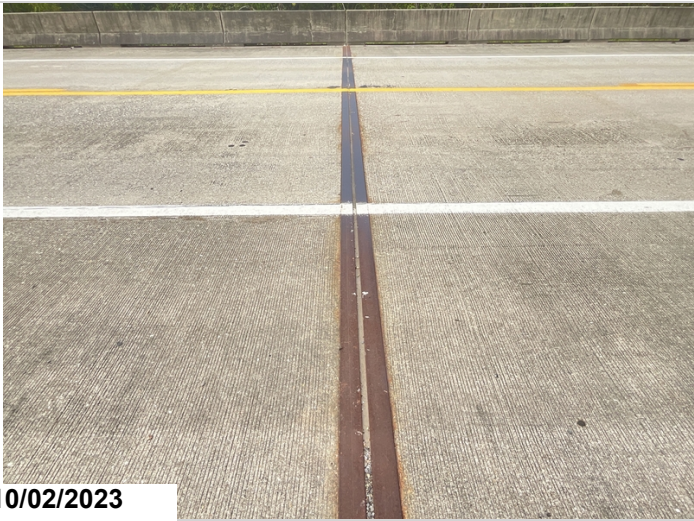
Typical joints are in good condition
