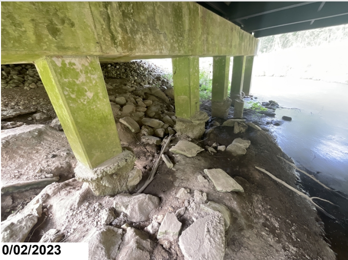
Bent 2 has some scouring and loss on rip to slope under span 1
