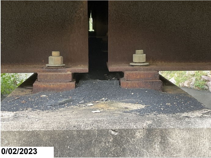
Bent 2 cap need cleaned
