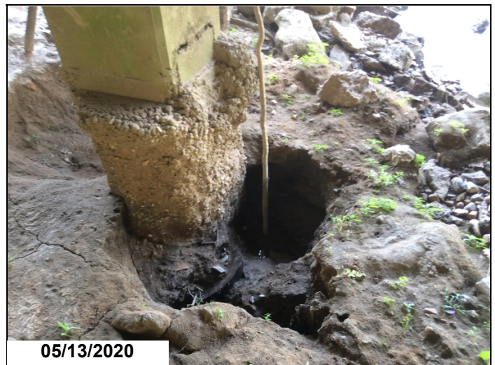
BENT 2 AT PILE 2 EROSION
