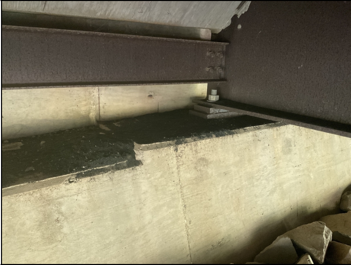
Photo of abutment 1 with sandblasting material on cap. From joint repairs in 2021.
