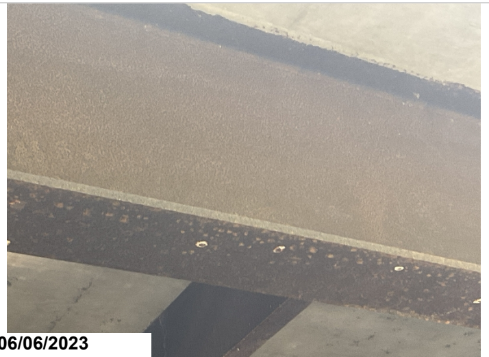
6/2023 Light brown rusting on out side beam in span span 3 left side photo taken
