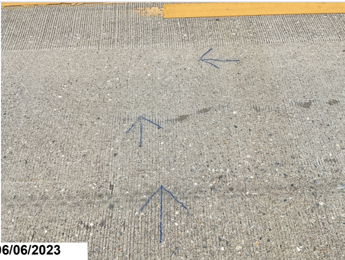
6/2023 typical cracking in deck top side most all spans photo taken in span 2 near bent 3
