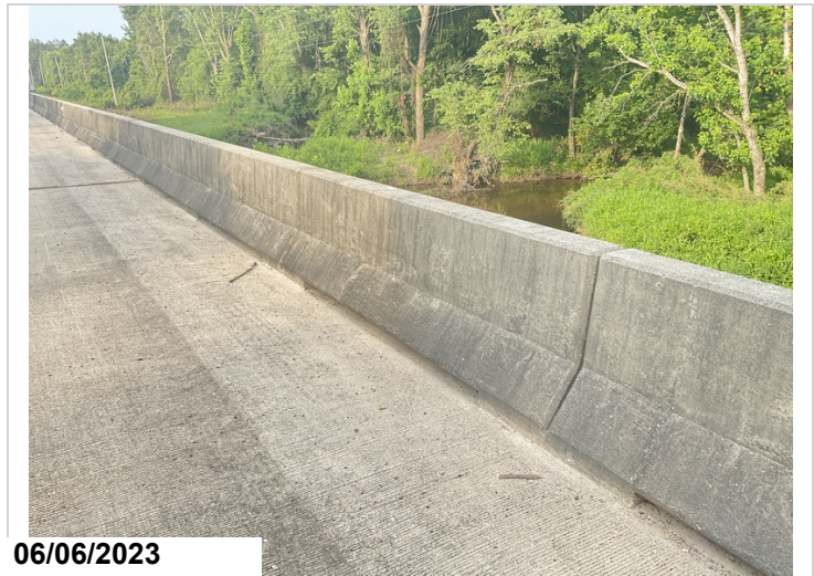
6/2023 Typical photo of concrete bridge railing in good condition
