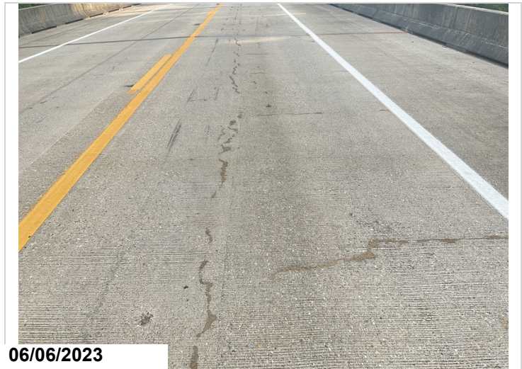
6/2023 small cracks in deck some sealed in past.
