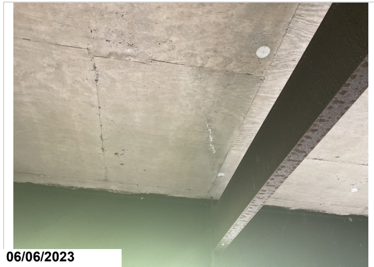
cracking with white efflorescence .photo taken in span 2 bay 1 at bent 2 area
