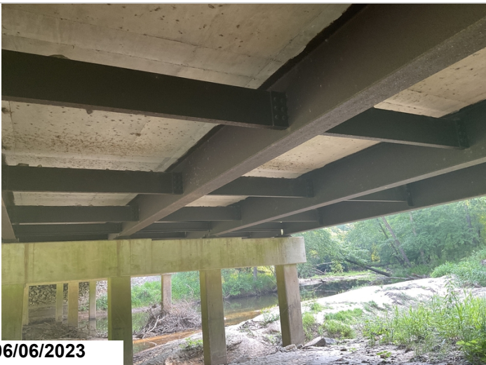
6/2023 Typical photo of wearing steel beams all spans
