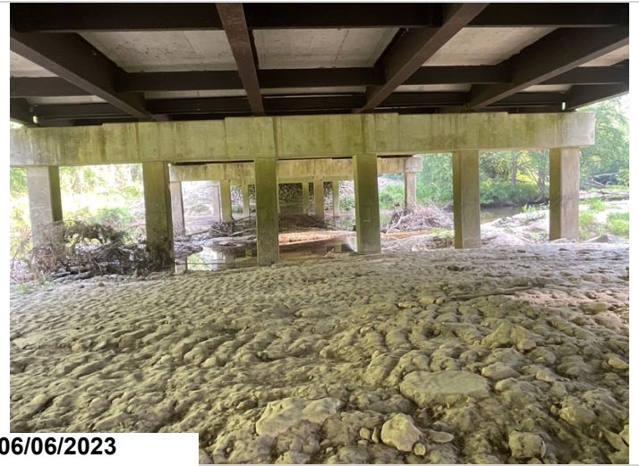
6/2023 typical bent photos steel piles with concrete encasement
