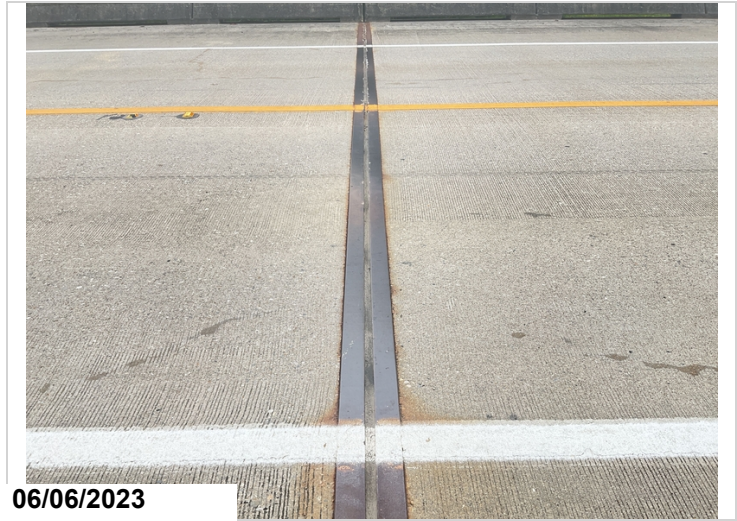
6/2023 photo of joint at bent 2 good condition.
