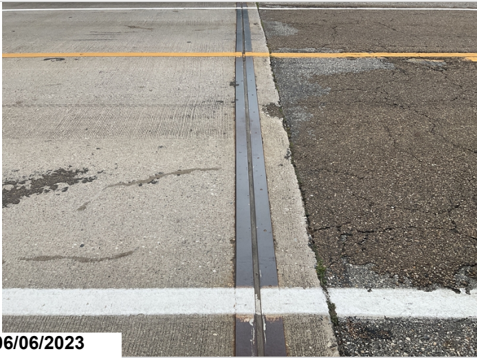
6/2023 photo of joint 1 beginning of bridge in good condition
