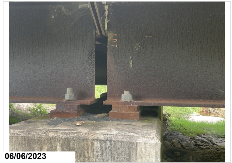
6/2023 typical photo of bearings
