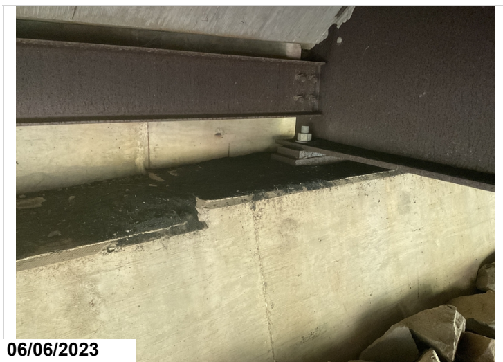
Photo of abutment 1 with sandblasting material on cap.From joint repairs in 2021.
