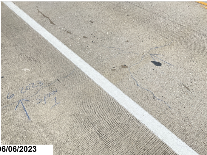
6/2023 unsealed cracks in deck photo of span 1 left side.
