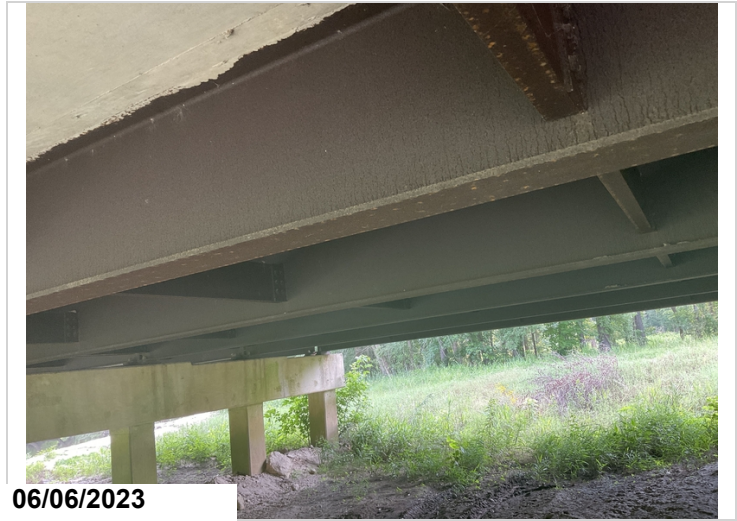
6/2023 typical photo of weathering steel beams. Photo taken in span 1
