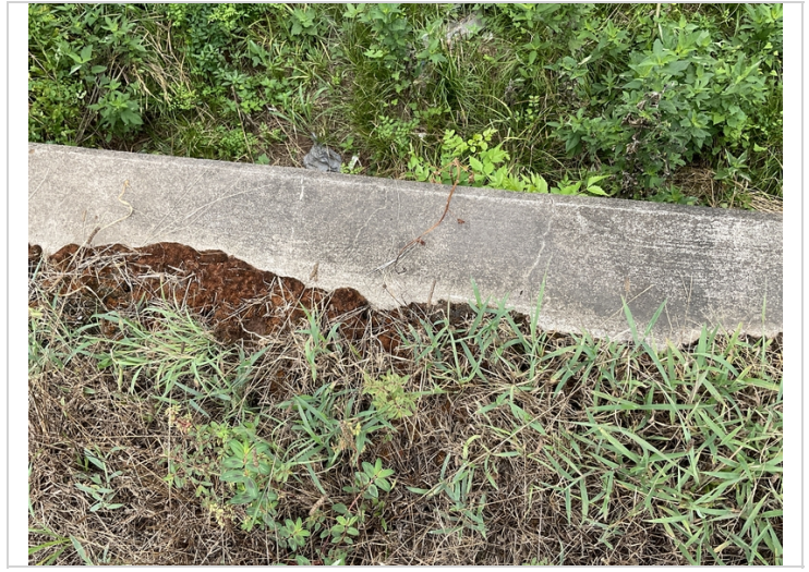
Cracking on headwall in various locations
