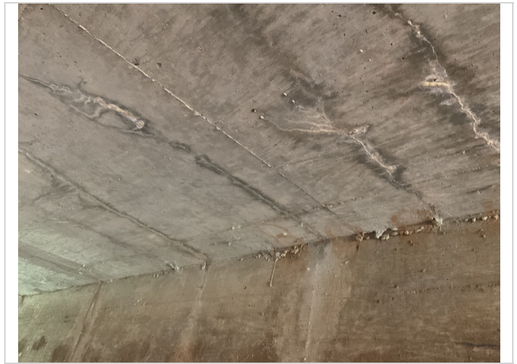
Efflorescence barrel 1
