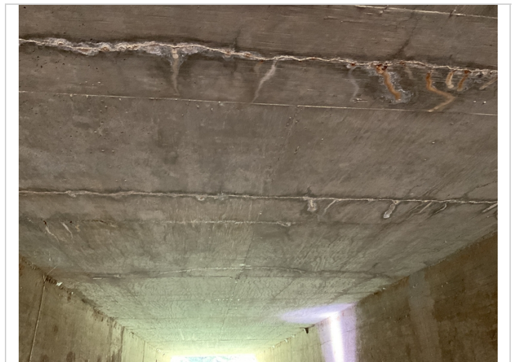
Cracking with efflorescence barrel 2
