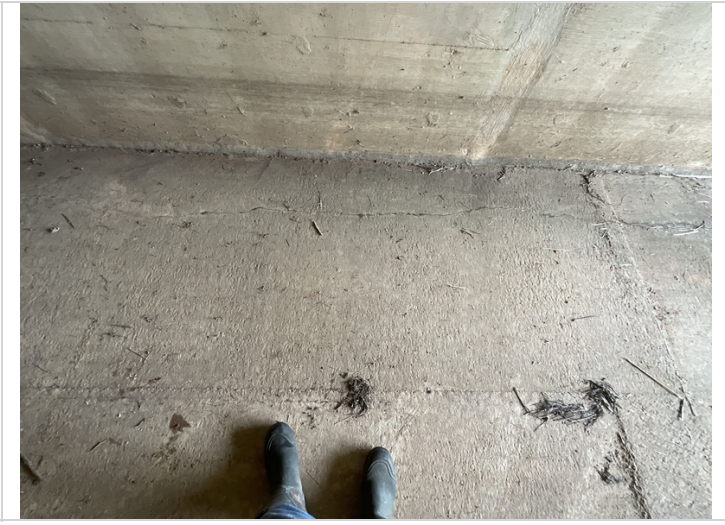
Longitudinal cracking in barrel 1
