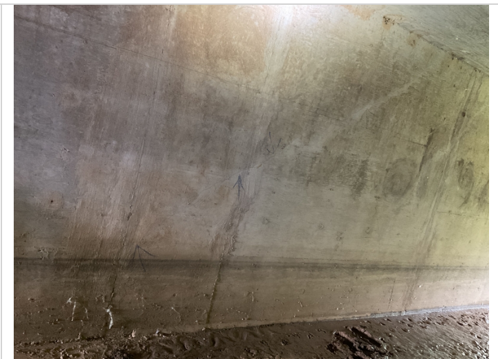
Longitudinal Cracking in barrel 2
