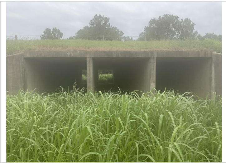
3 barrel culvert
