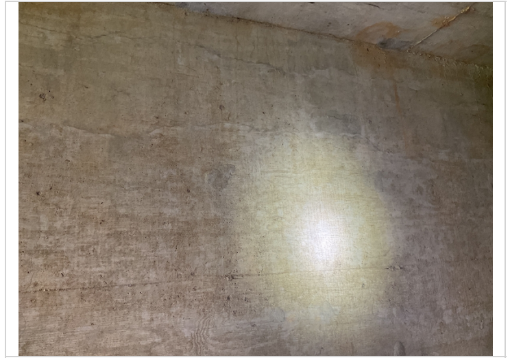
Longitudinal cracking barrel 1
