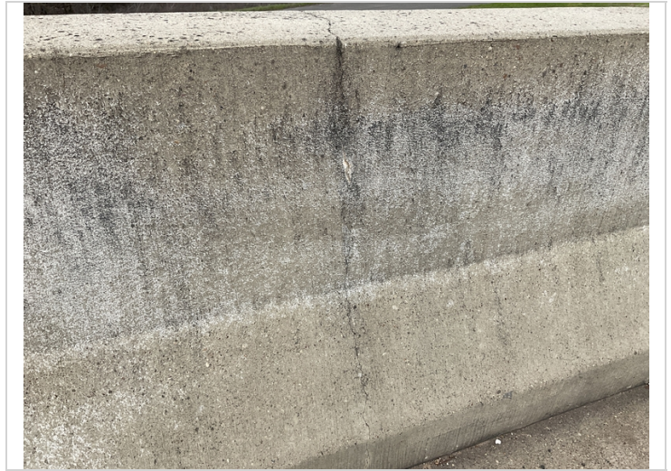
Cracking in bridge railing
