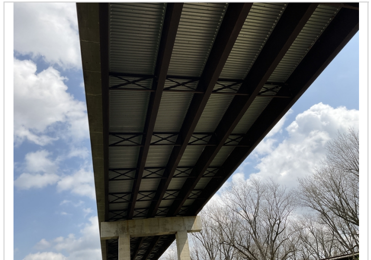
Span 13, 14, and 15 have diaphragms
