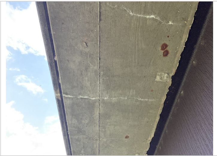
Efflorescence in overhangs
