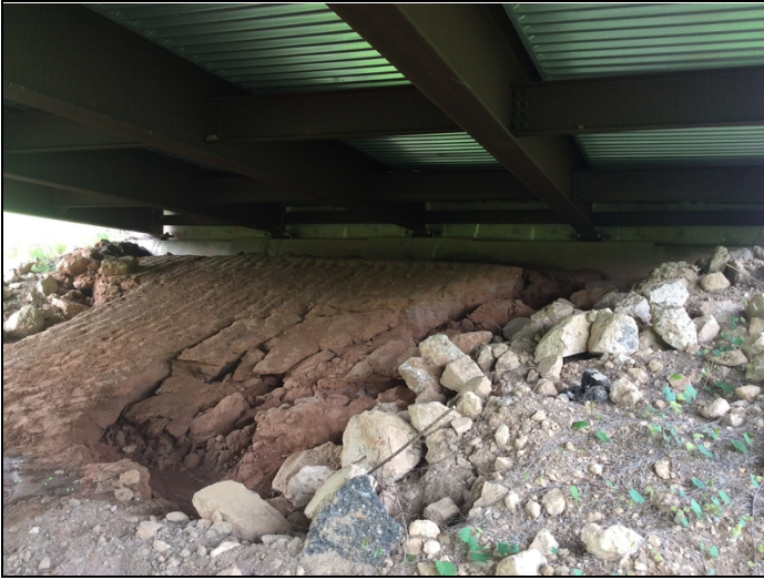
Erosion under span 1 at abutment
