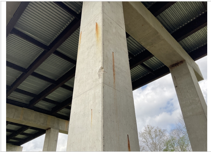
Bent 8 column 2 spall
