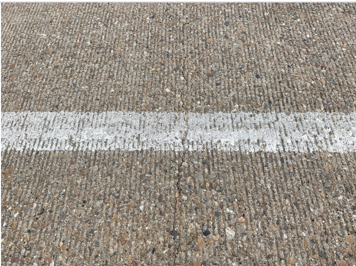
Sealable deck cracking
