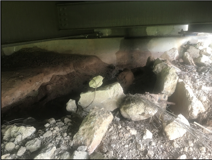
EROSION AT BENT 1 ABUTMENT AND UNDER SPAN 1
