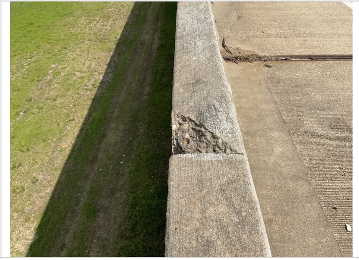
Spall in bridge railing
