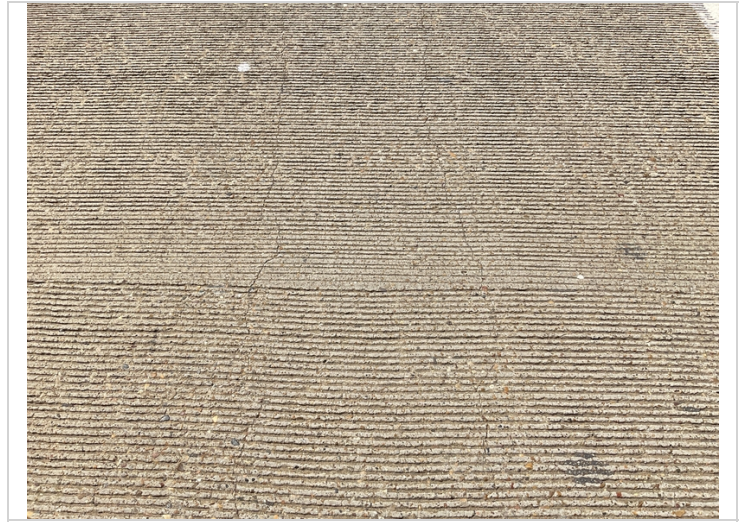
Deck cracking
