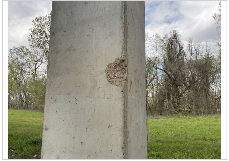
Bent 11 column 1 spall
