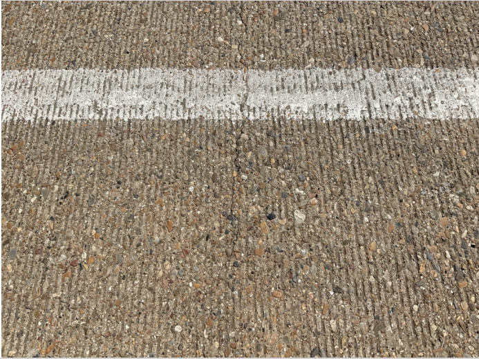
Deck cracking
