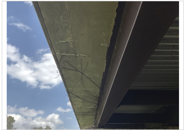
Efflorescence in overhangs
