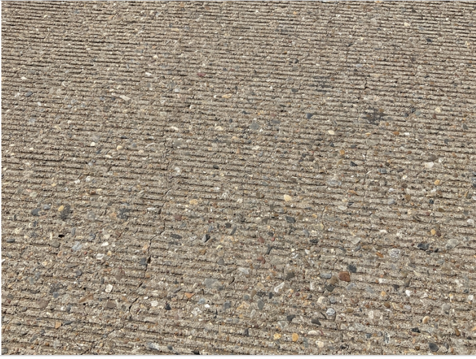
Deck cracking
