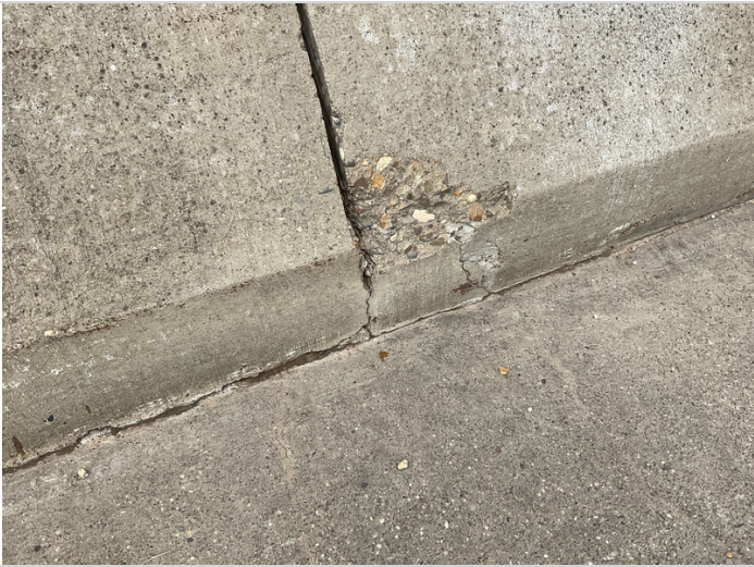
Spalls in bridge railing
