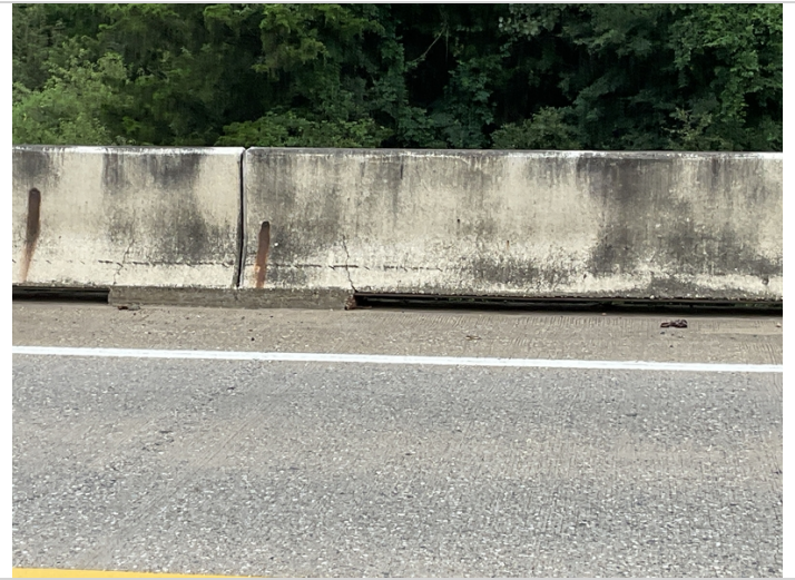
Rust staining and cracking in various locations of parapet wall
