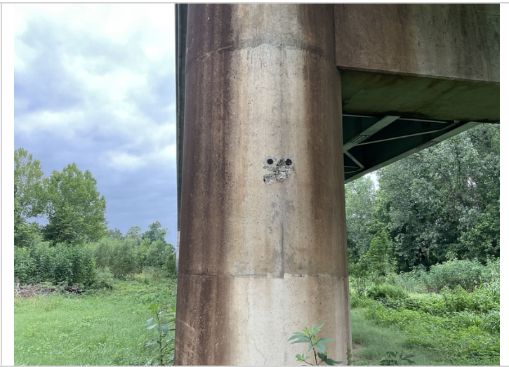
Pier 3 column 4 Delam
