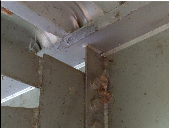
Span 9 brace weld between beams 1 and 2
