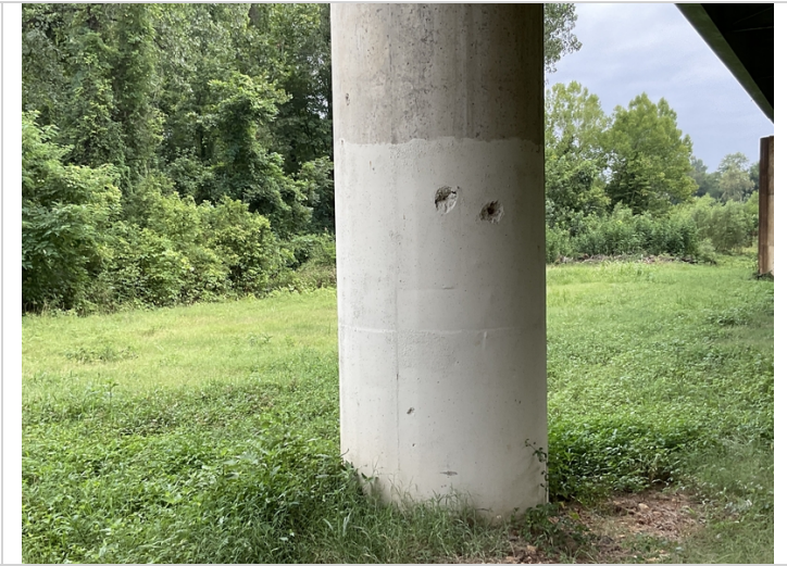
Pier 2 column 1 delams
