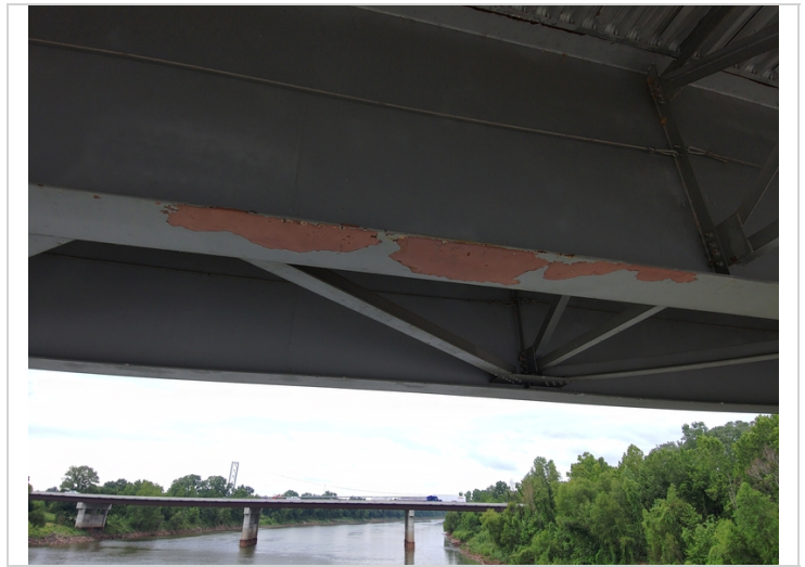
Paint loss on beams
