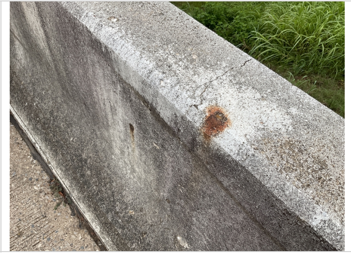
Cracking in parapet wall various locations
