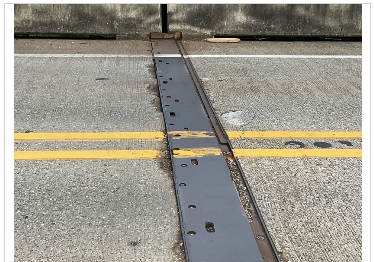
Delams around first slider plate
