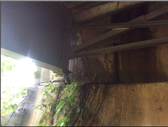
Joints leaking beginning and end of bridge causing rust on bearings.
