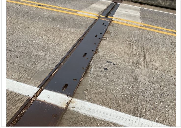
Delams around assembly joint #2
