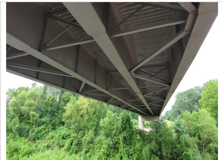
Underside of deck, steel beams
