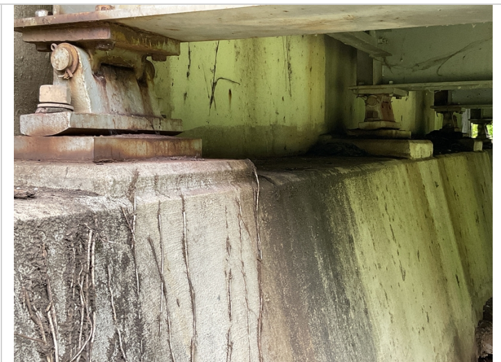
Corrosion on rocker bearings abutment 1
