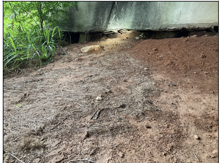
Updated erosion on bent 10
