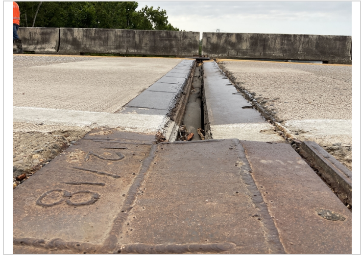
Assembly joint #2 repairs
