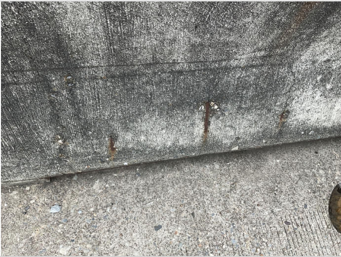
Rebar exposed in various locations of parapet wall
