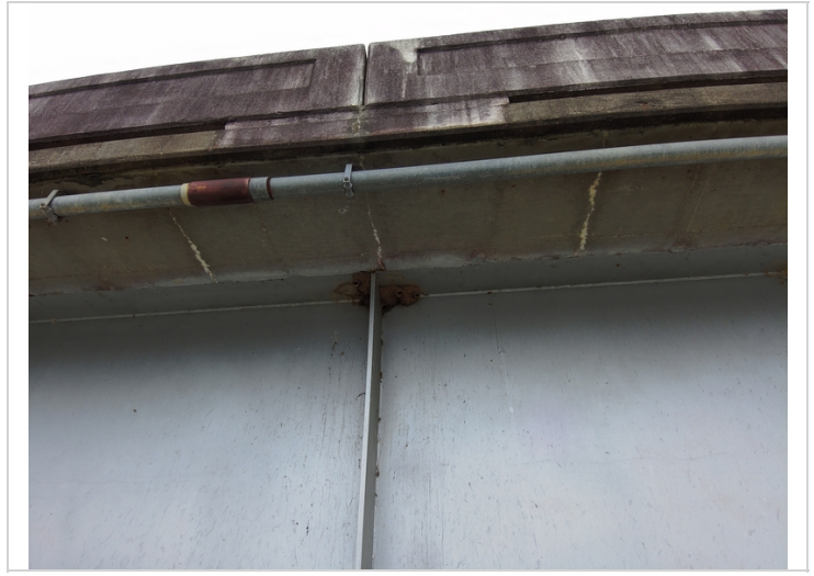
Cracking with efflorescence in overhangs
