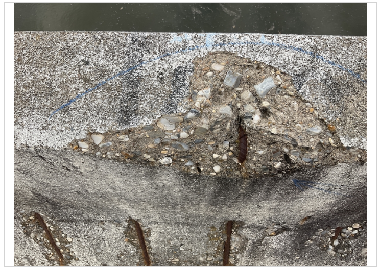
Large spall on top of parapet wall right side with rebar exposed
