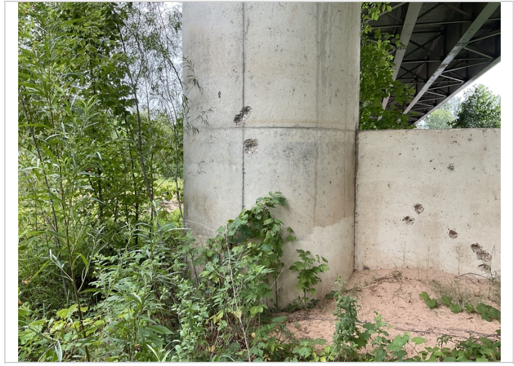
Pier 4 column 1 Delam
