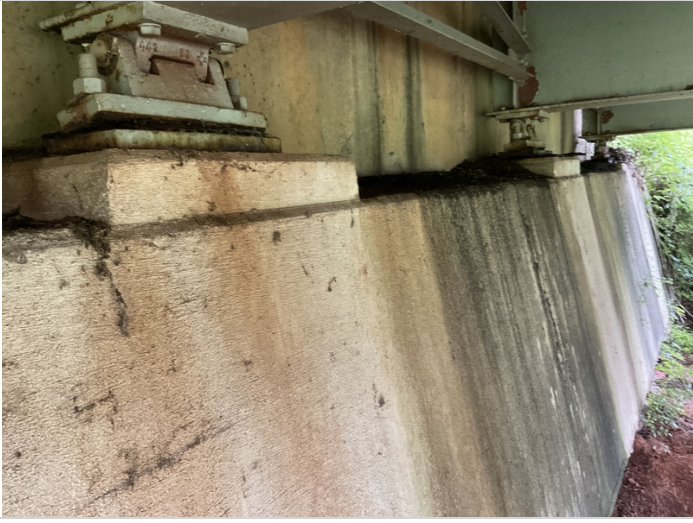
Corrosion pack rust abutment 2 bearing
