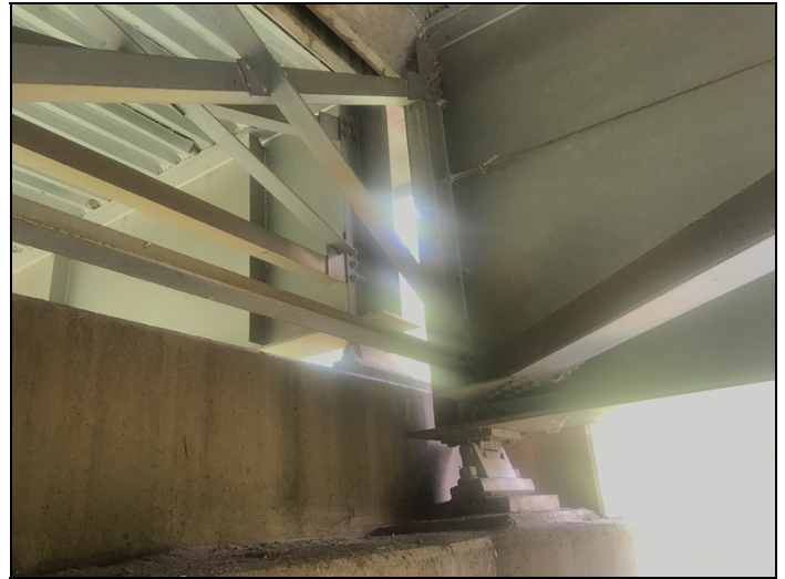
Bent 4 joint leaking causing rust on bearings and some debris on top of cap
