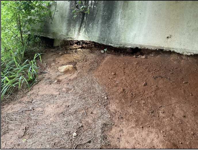
Updated erosion on bent 10
