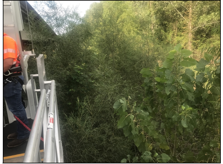
Trees need cut span 4 snoopers hitting trees at inspection
