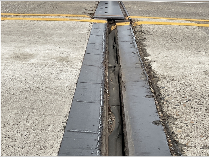
Assembly joint #2 repairs
