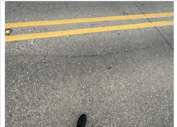
Large cracking in approach slab
