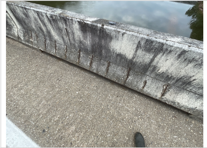
Rebar exposed in various locations on parapet wall
