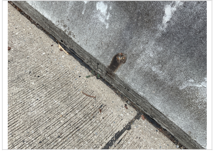
Delam in parapet wall various locations
