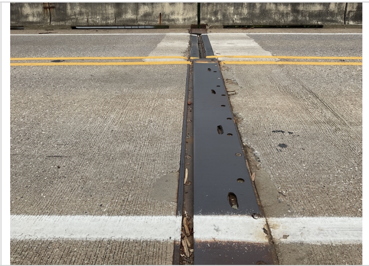
Assembly joint #2 repairs
