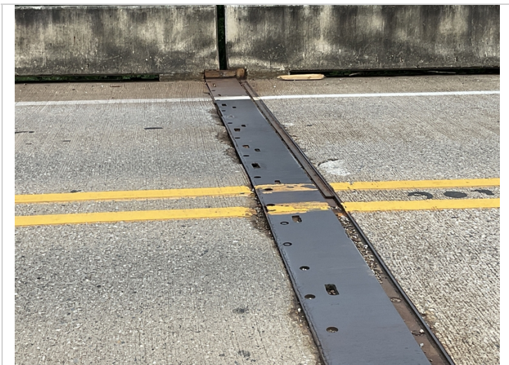
Assembly joint #1 left side has broken loose and can be heard well when any vehicle passes over it
