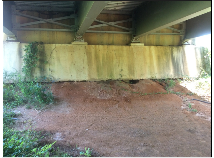
Bent 10 erosion under cap. Piling exposed
