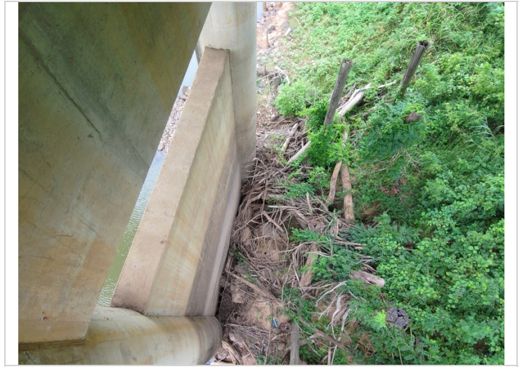
Debris buildup behind pier 7
