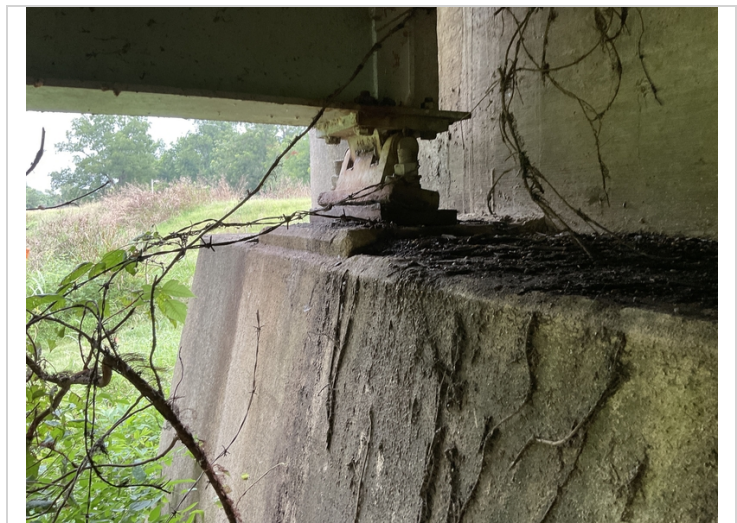
Bearing is free floating from section loss abutment 2
