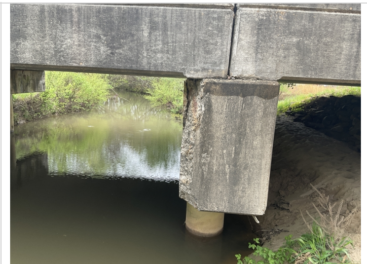
LT side spall with rebar exposed
