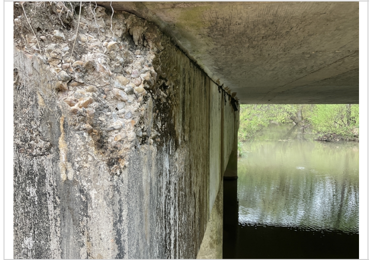
Rt side bent 2 spall
