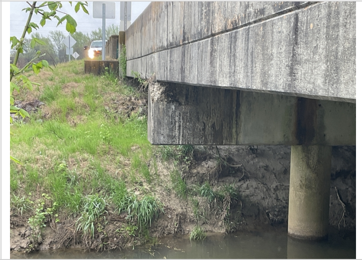
Rt side cap at bent 2 spall
