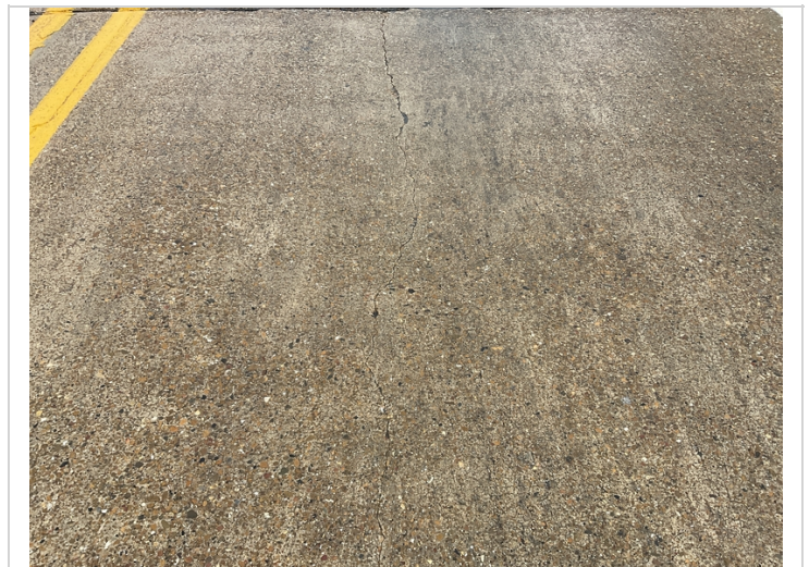
Concrete approach slab cracking both sides of bridge
