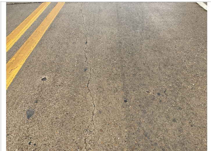
04/2022.. concrete approach slab has cracks both sides of bridge
