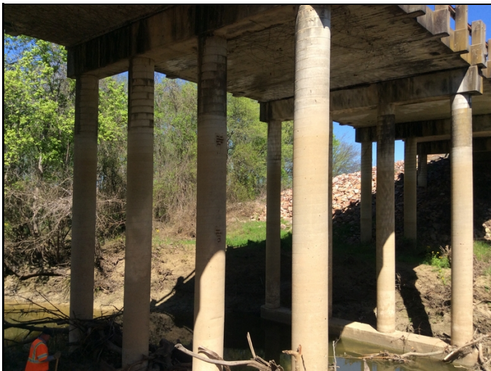
CONCRETE COLUMN AT BENT #5, COLUMN #2 (NUMBERED LEFT TO RIGHT) MINOR SPALLS WITH REBAR EXPOSED
