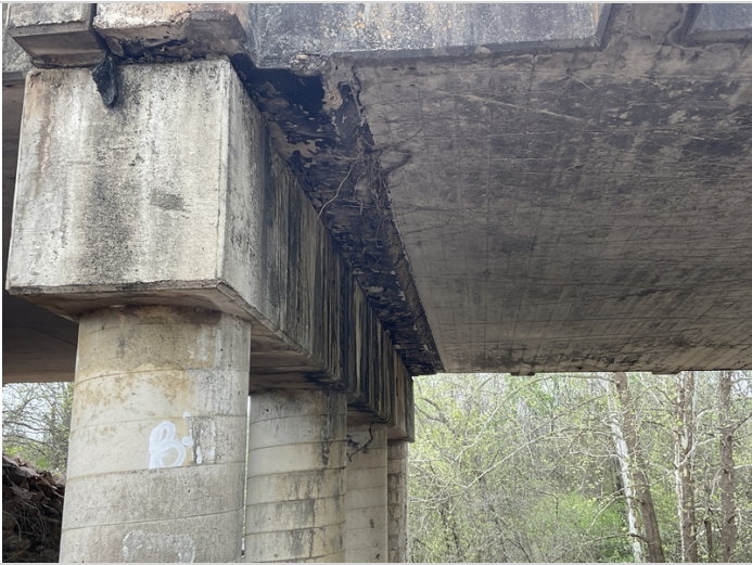
Underside of deck joints leaking
