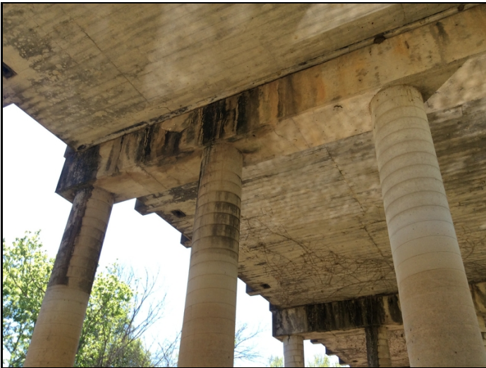
CONCRETE CAP AT BENT #4, NORTH FACE 18"X24" DELAMINATION ON CAP BETWEEN COLUMNS 1 and 2
