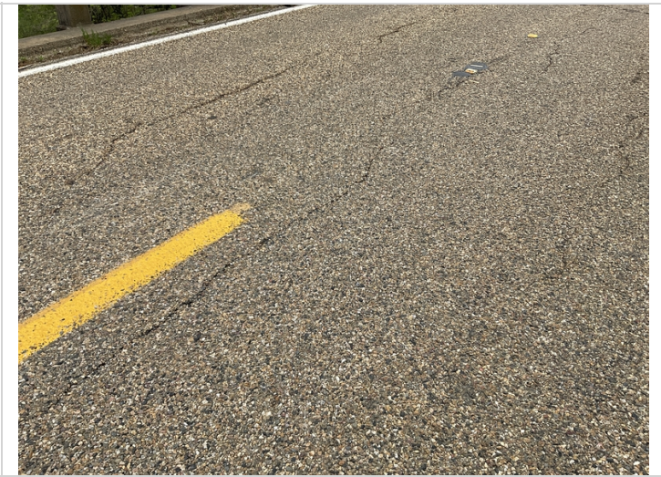
Cracking throughout deck various locations
