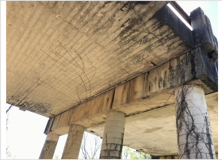
Rebar exposed span 2
