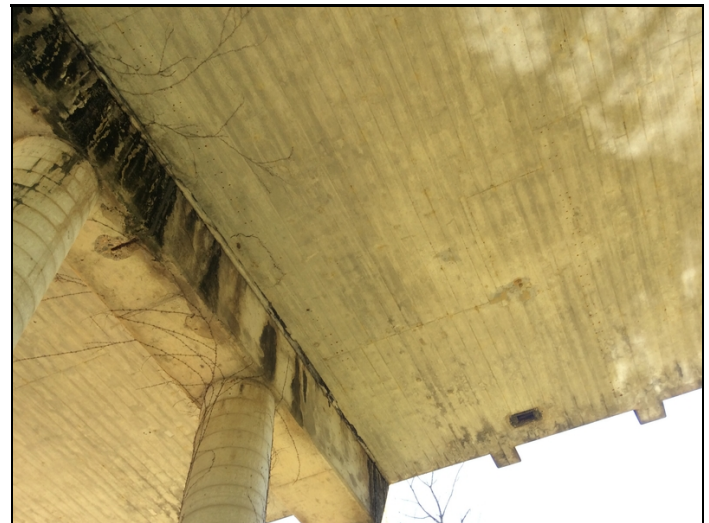
SPAN 3 DELAM BOTTOM DECK AT BT 3 16'X16' CENTER BRIDGE.
