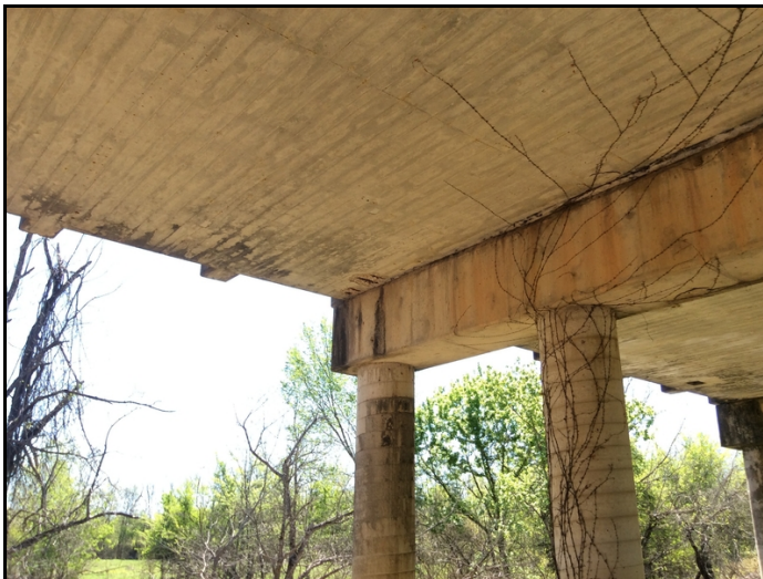
BOTTOM OF CONCRETE DECK SPAN #2 HAS A 1'X1' SPALL W/REBAR EXPOSED.
