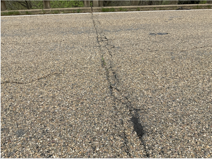
Asphalt over joints not allowing them to move properly
