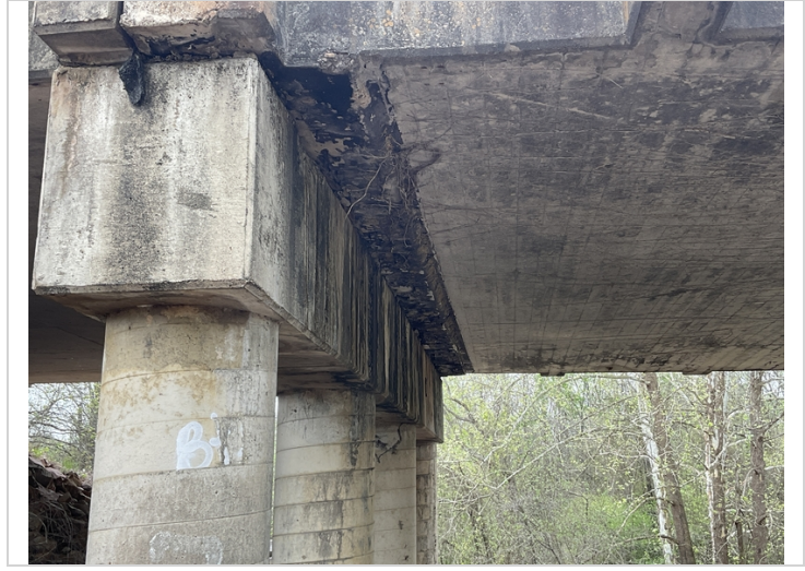
Underside of deck joints leaking
