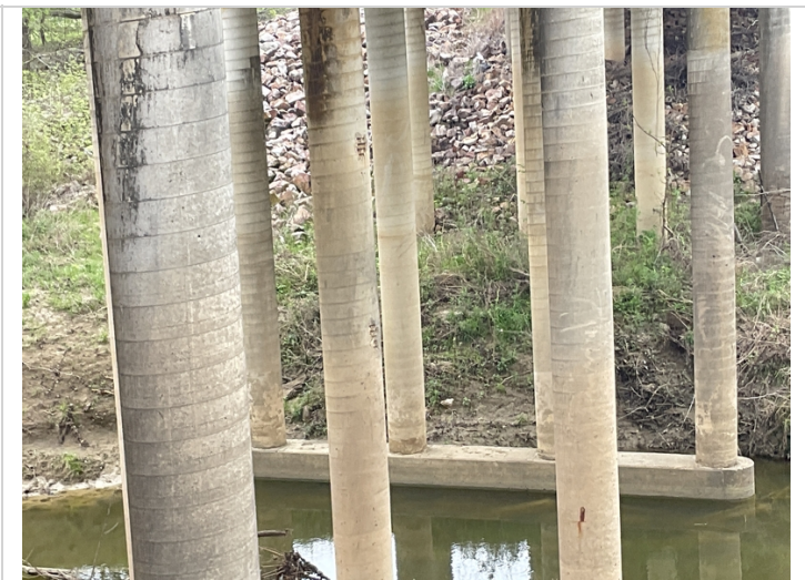
Bent 5 column 2 spalls with exposed rebar
