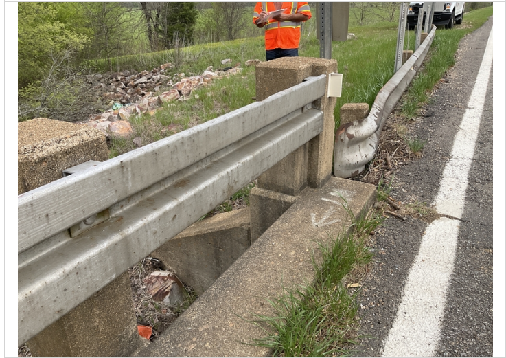
Corrosion and paint loss on both metal railings on bridge
