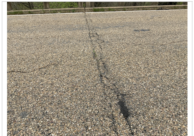
Asphalt over joints not allowing them to move properly
