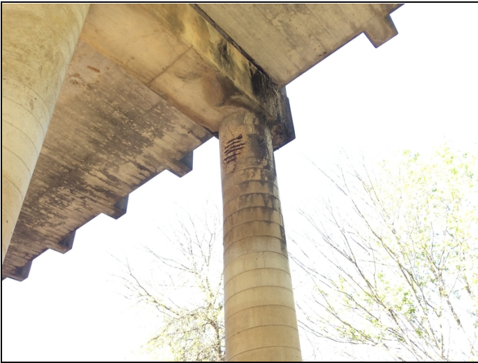
CONCRETE COLUMN #4 AT BENT #6 MINOR SPALL WITH REBAR EXPOSED APPROX. 1'X1' NUMBER LT TO RT WITH LOG MILES.
