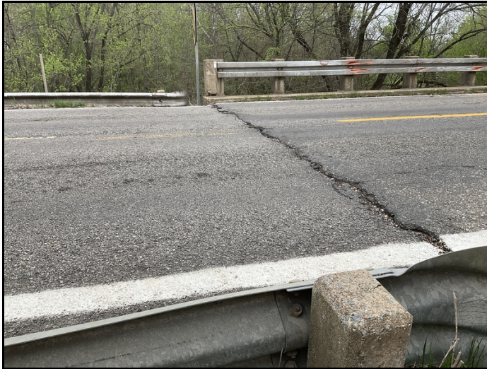
Sediment at approach roadway causing impact to beginning of bridge
