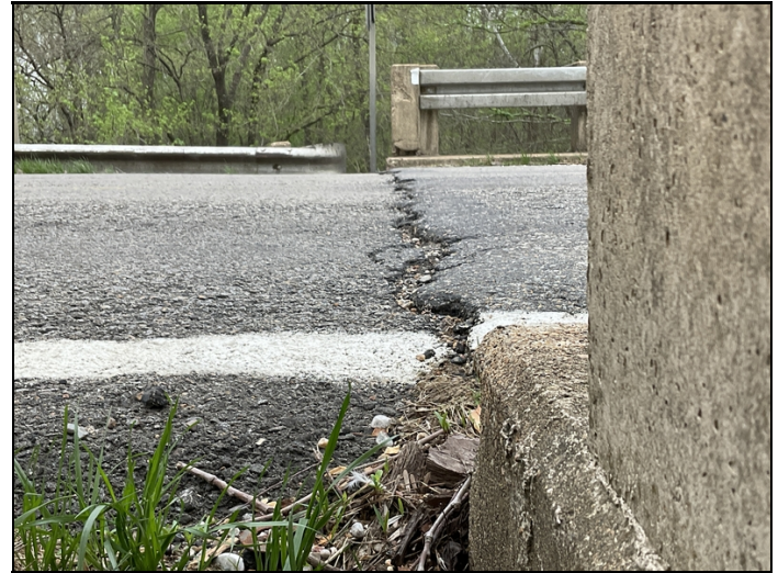
Sediment at approach roadway causing impact to bridge
