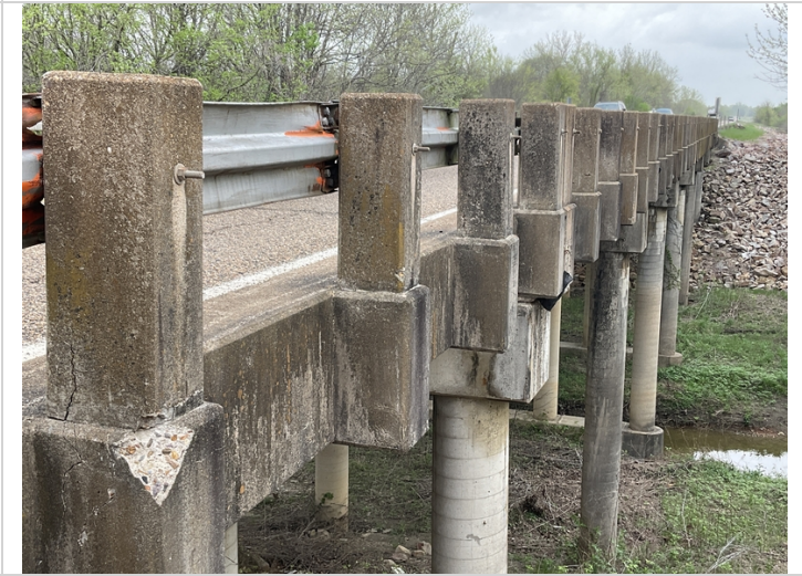
04/2022... Damage to concrete bridge railing, entire last span on LT side
