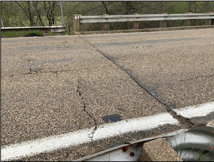
Sediment at approach roadway causing impact to end of bridge
