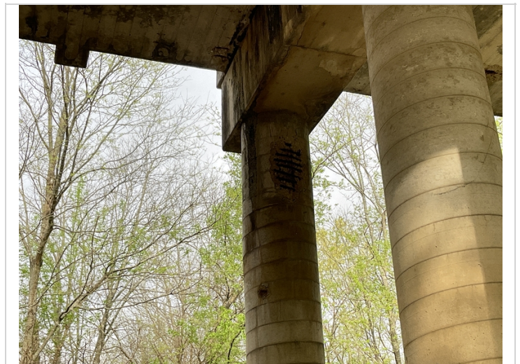
Exposed rebar on bent 6 column 4
