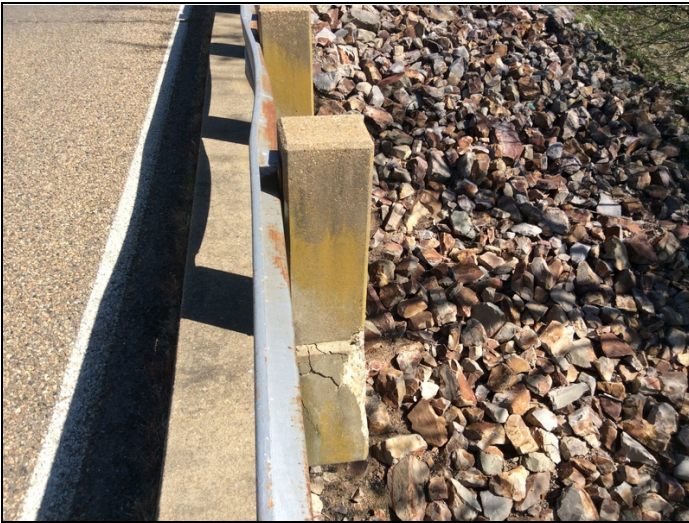
Span 2 left side post crack
