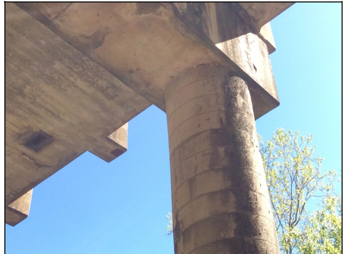
Bent 6 column 1 small crack at top of column
