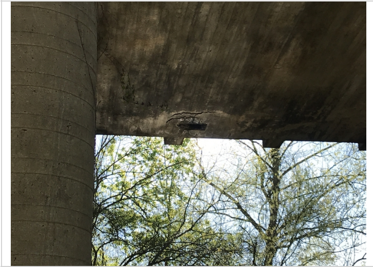
Delam at drain span 4 LT side
