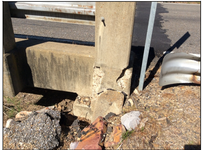
CONCRETE END POST BENT 1 RIGHT & LEFT SIDE HAS A POST THAT IS BROKEN AT THE BASE FROM COLLISION DAMAGE WITH REBAR EXPOSED.
