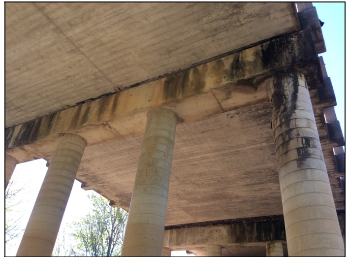
CAP @ BENT #6 HAS NUMEROUS CRACKS IN BOTTOM AREA OF CAP.
