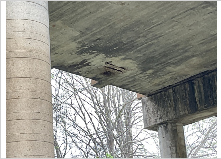
Exposed rebar on underside of deck various locations
