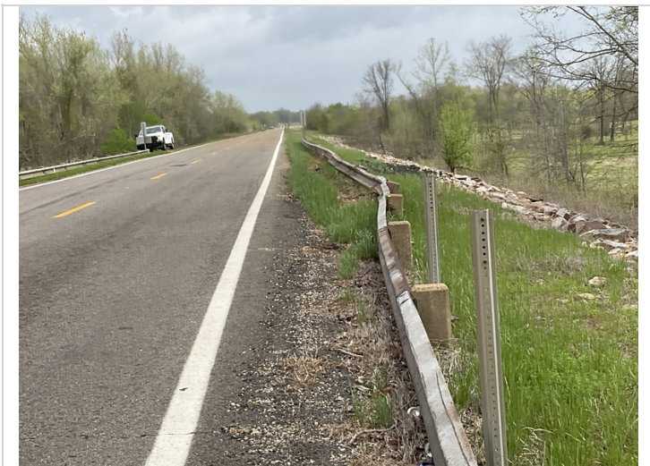
LT side metal bridge railing damage entire length of bridge
