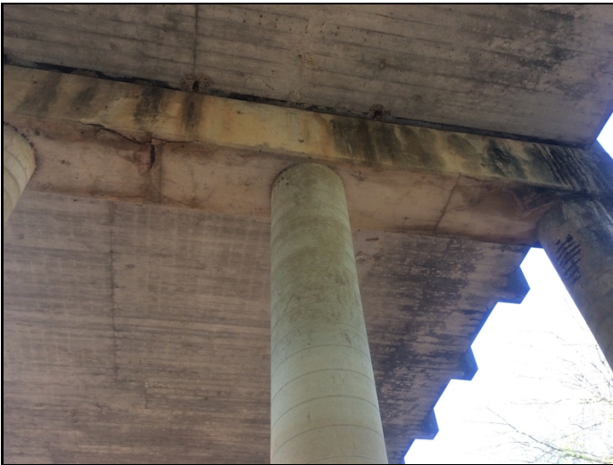
Bent 6 cap and column 4. Cracking and spall with rebar exposed
