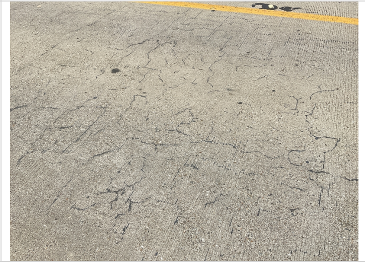
Some cracks in deck have been sealed in the past
