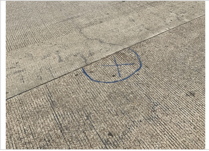
Span 4 RT side Delam. Southbound lane mid span
