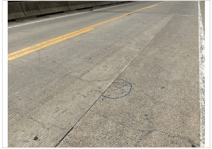
Span 4 RT side Delam. Southbound lane mid span
