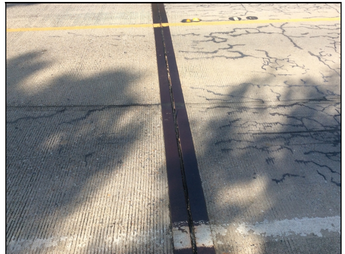
JOINT MATERIAL AT ALL BENTS NEED REPLACED
