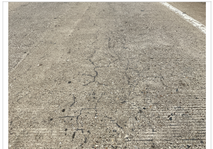
CS2 cracking in various locations of deck
