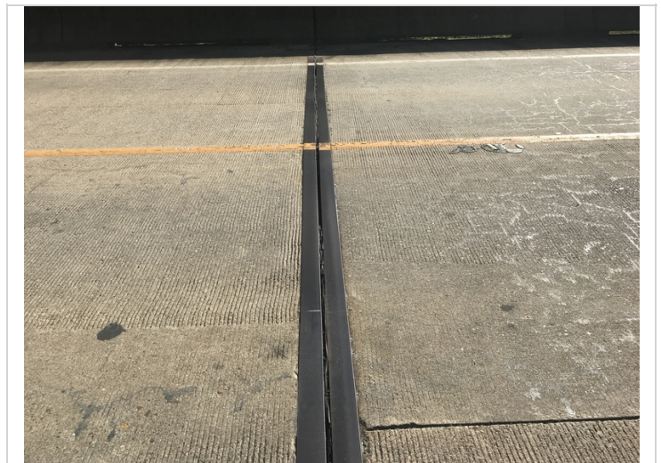
Joint material missing at bent bent #3 and #4 #5
