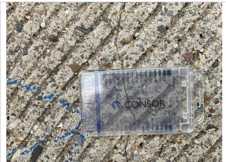
CS2 cracking in various locations of deck
