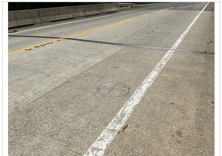
Span 4 RT side Delam. Southbound Lane near Bt 5
