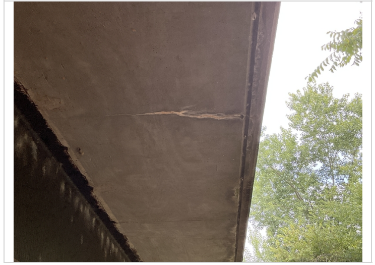
Efflorescence on overhangs various locations
