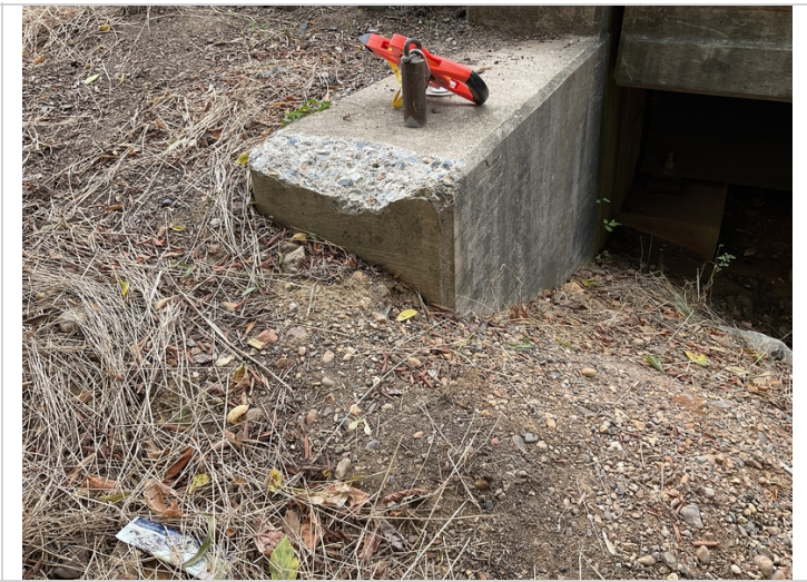
Bent 6 Abutment LT Side Spall
