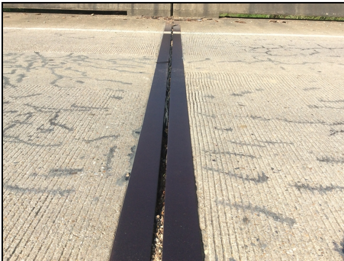
JOINT MATERIAL AT ALL BENTS NEED REPLACED
