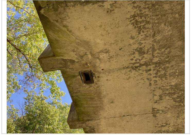
Spall in span 3 LT side underside of deck
