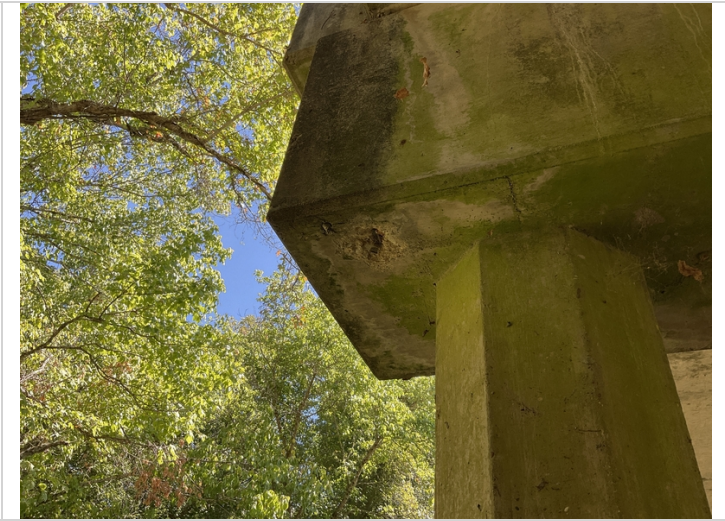
Bent 3 exposed rebar LT side of cap
