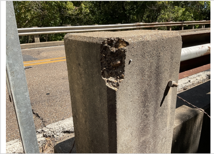
RT side beginning of bridge spall on concrete bridge railing
