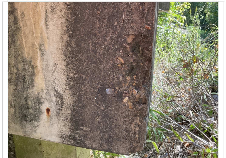
Bent 2 spall on cap RT side
