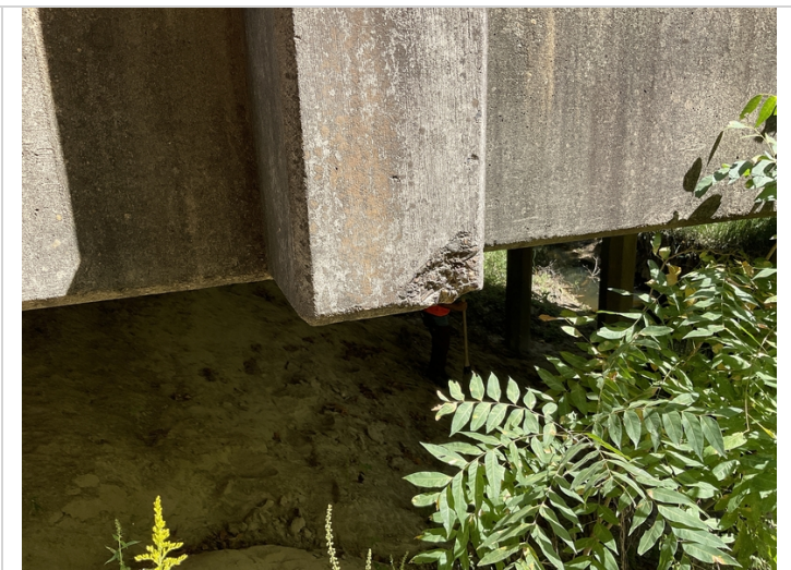
Spalls on concrete bridge railing
