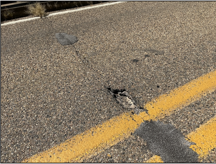
Potholes on asphalt wearing surface at all joint lines.
