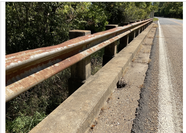
Corrosion on metal bridge railing
