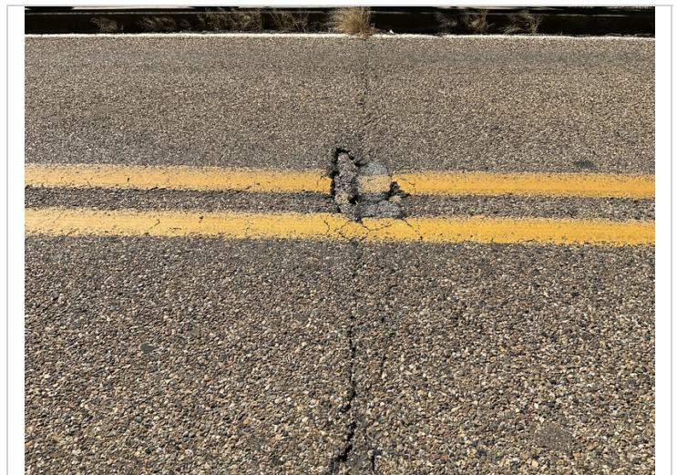
Potholes on asphalt wearing surface at all joint lines.
