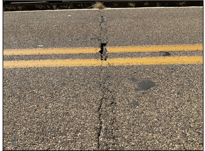
Potholes on asphalt wearing surface at all joint lines.
