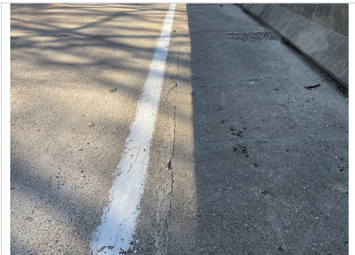
04/2022... deck cracking running entire length of bridge both sides
