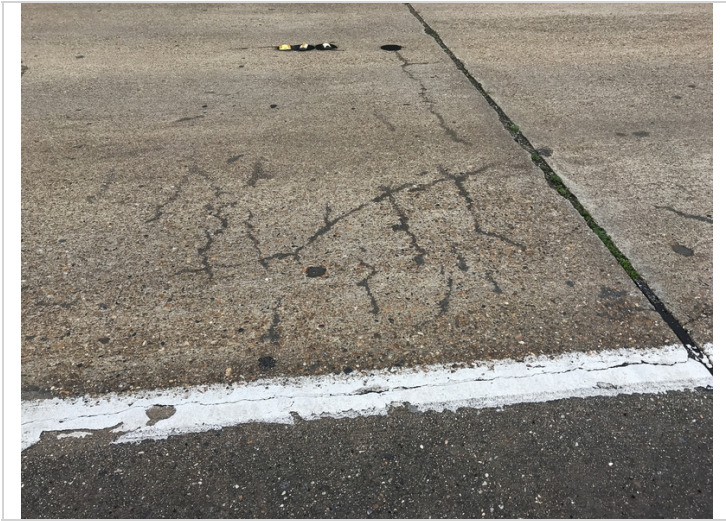
Sealed deck cracks
