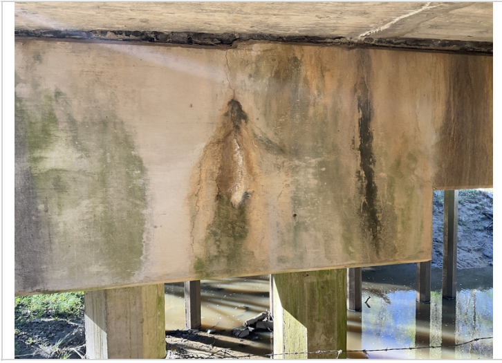
04/2022... efflorescence and cracking on caps various locations
