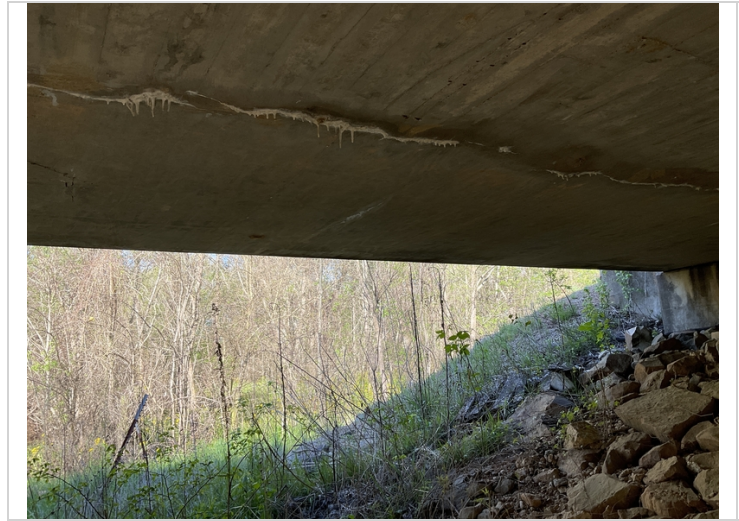
04/2022.. joints leaking along longitudinal crack with efflorescence
