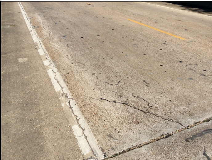
CONSTRUCTION JOINTS WHERE DECK WAS WIDENED LONGITUDINAL CRACKS WITH EFFLORESCENCE LEAKAGE AT CONSTRUCTION JOINTS.
