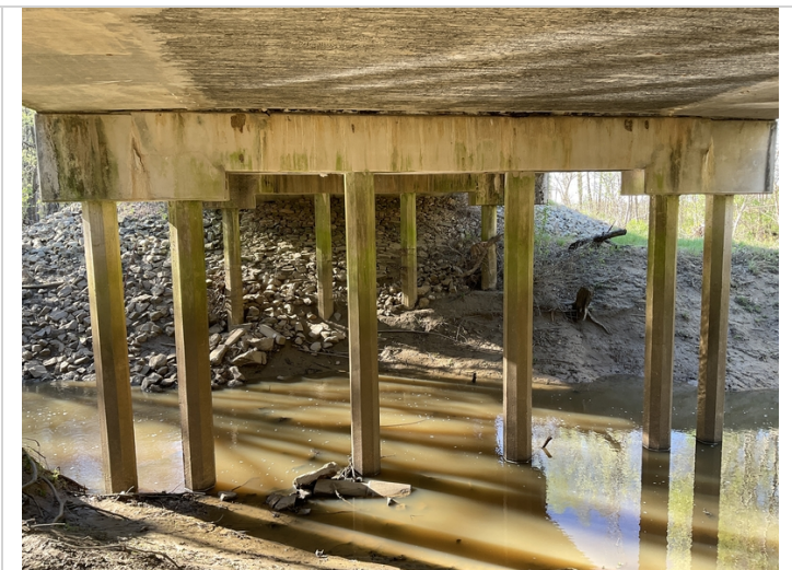
04/2022.. concrete caps and piles
