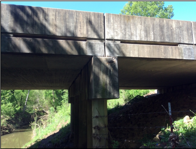
End cap BT 2 small spall
