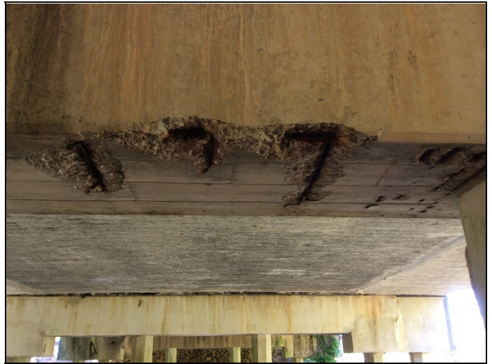
CONCRETE CAPS BENT 2 BOTTOM OF CAP HAS SEVERAL SPALLS WITH REBAR EXPOSED
