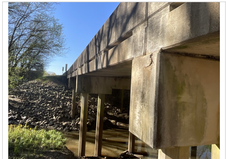
04/2022... spalls in caps at various. Locations
