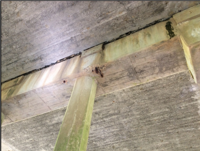
BENT 3 BOTTOM OF CAP HAS MINOR SPALLS WITH REBAR EXPOSED
