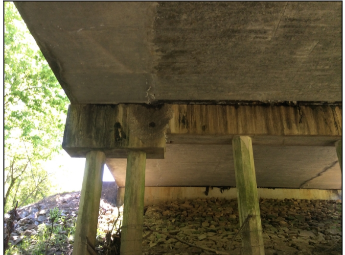
BENT 4 CAP HAS A LARGE SPALL AND SMALL SPALL WITH REBAR EXPOSED
