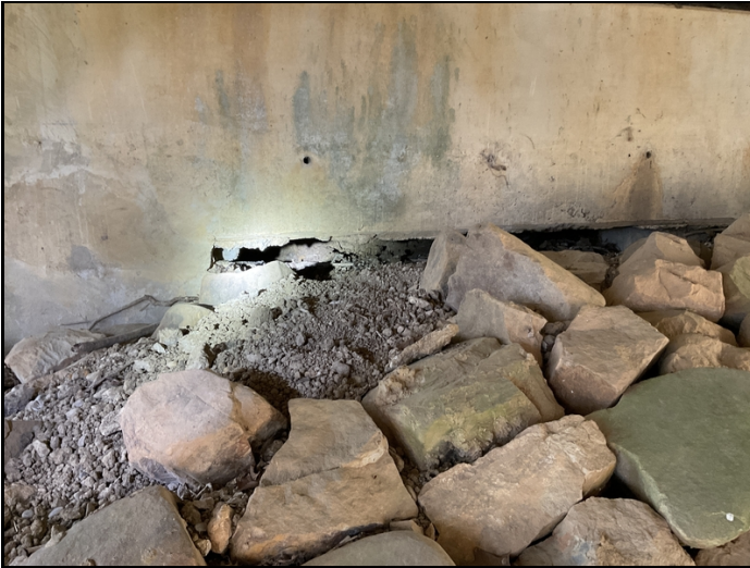
Hole under End Bent LT side
