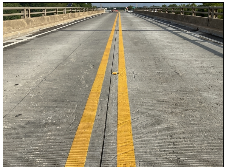
08/22 Repaired popout due to hydro overlay
