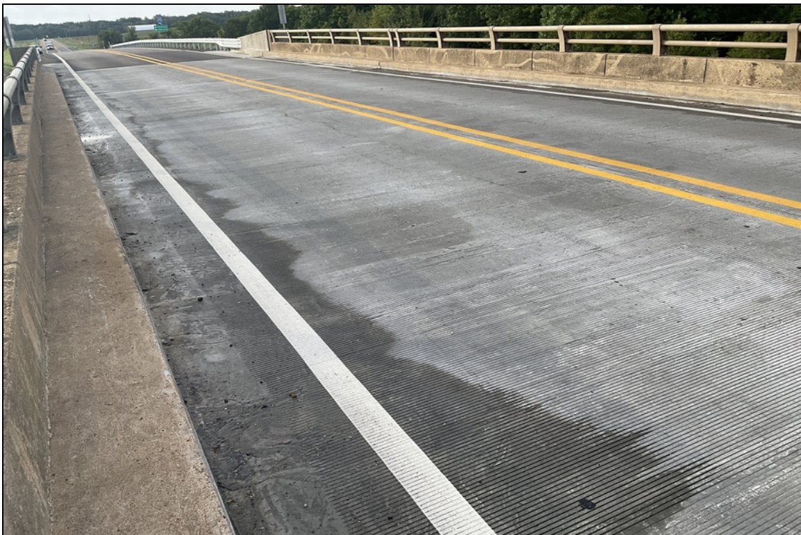
08/22 new hydro overlay per this inspection
