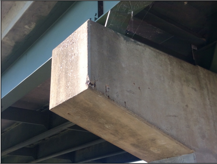
Bent 2 cap minor spall with rebar
