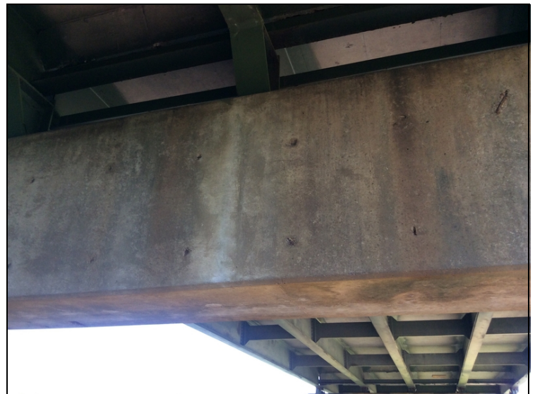
Minor areas bent 4 cap rebar exposed
