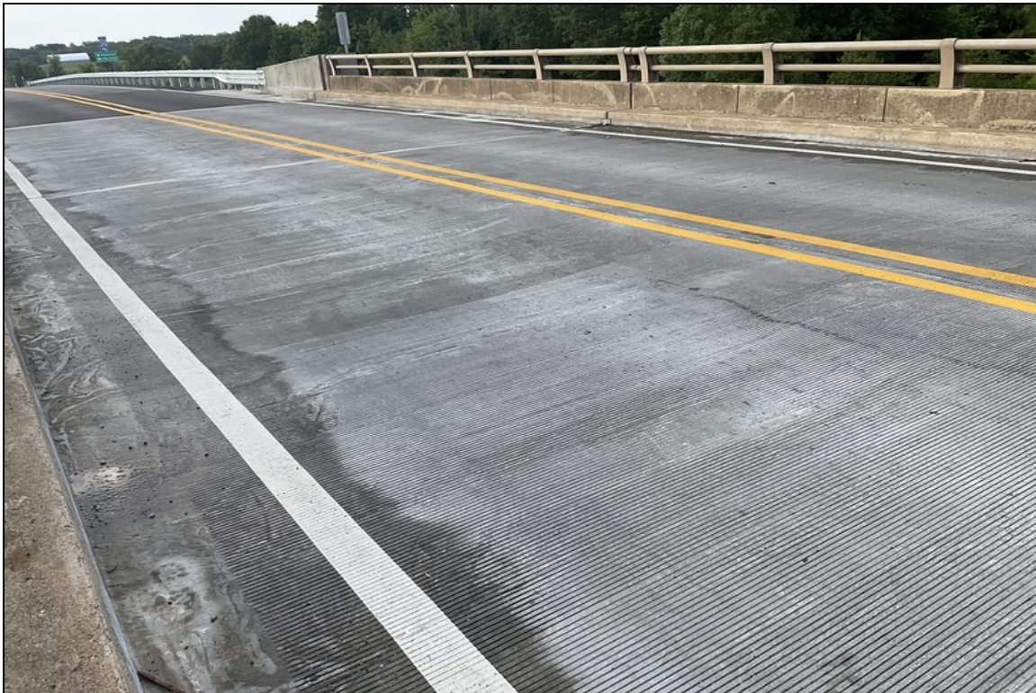
08/22 per this inspection hydro was completed on bridge deck
