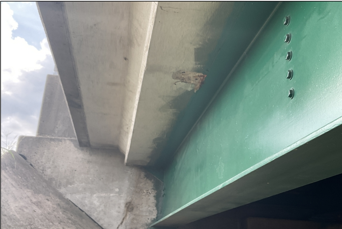
08/22 small delam span 4
