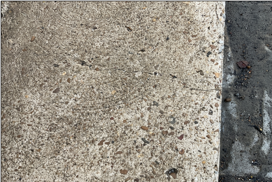
08/22 cracking in side of deck wheelguard various locations
