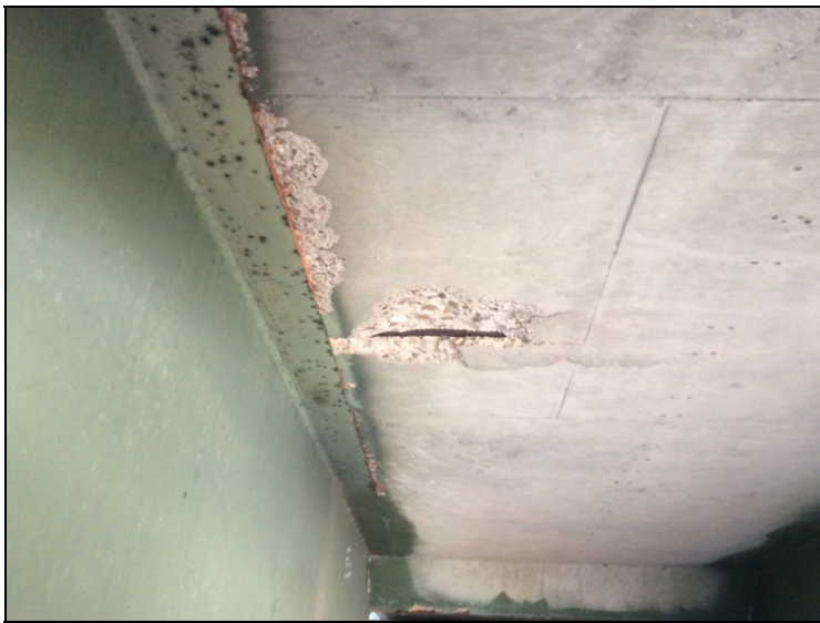
SPAN 1 SPALL WITH REBAR EXPOSED
