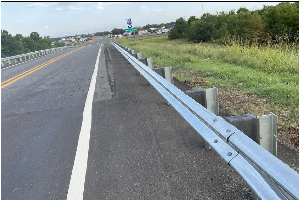
08/22 new guardrail installed per this inspection
