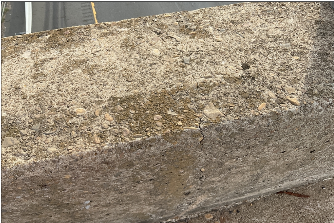
08/22 cracking in concrete bridge railing various locations
