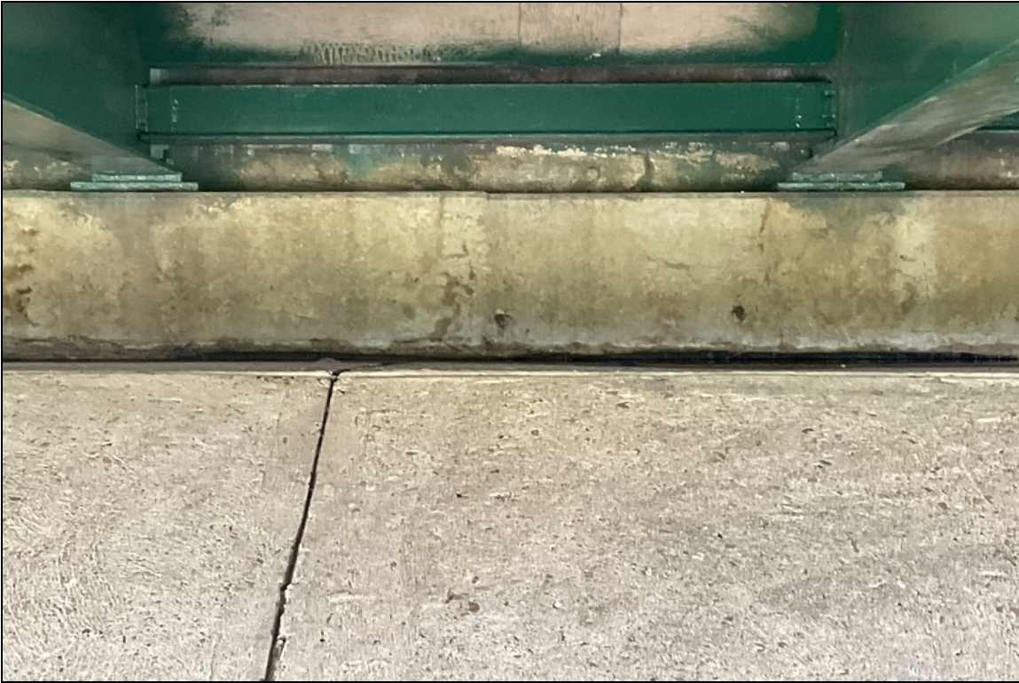
08/22 rust beginning to show on all bearings
