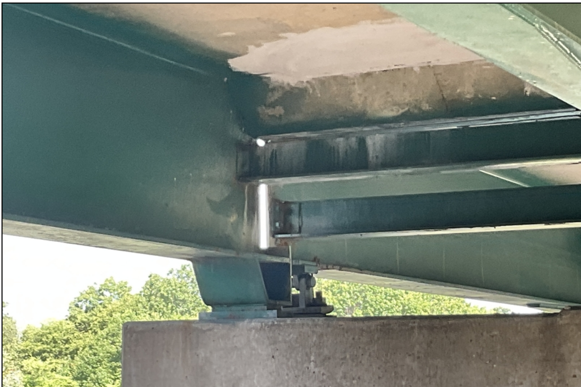
08/22 rust at end of beams various locations
