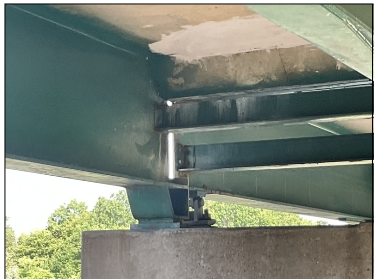
08/22 Patch work was completed when new hydro overlay was done..
