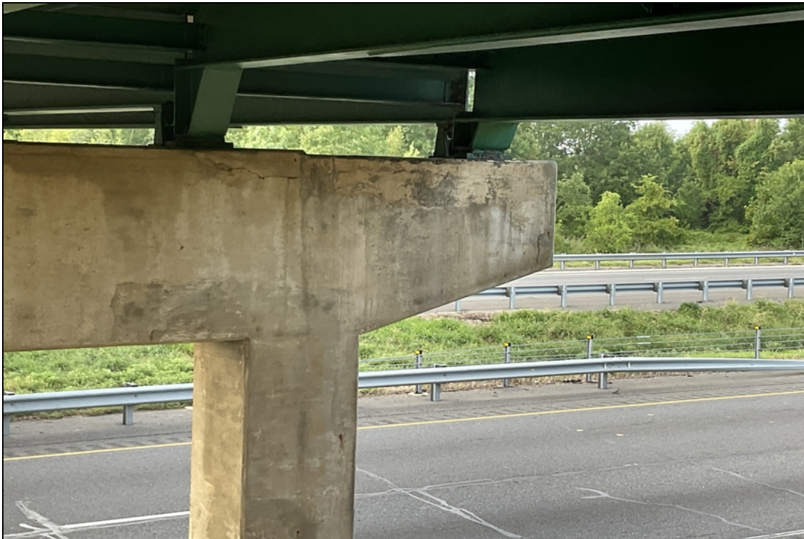
08/22 cracking on bent 2 grows to end of cap
