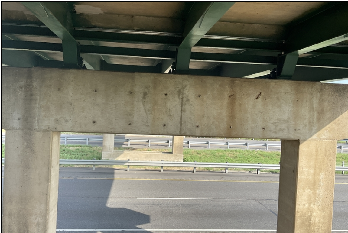
08/22 exposed rebar on bent 4
