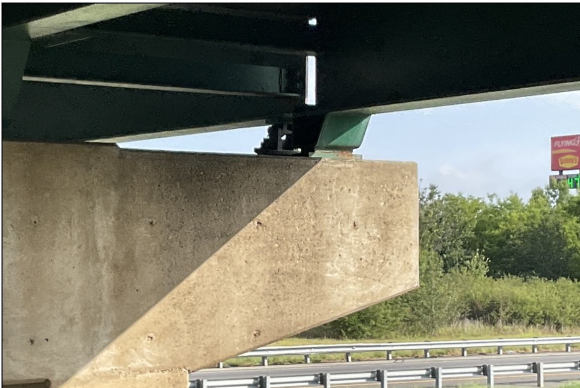
08/22 rust beginning to show on all bearings
