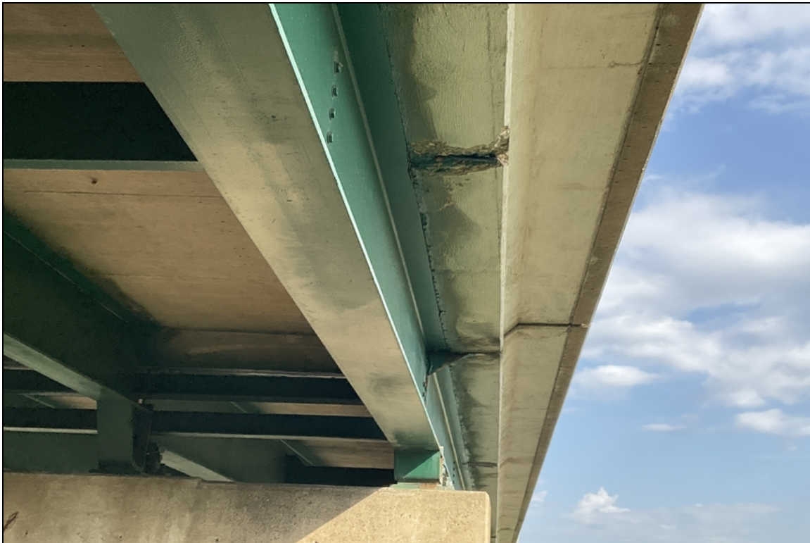
08/22 exposed rebar span 4
