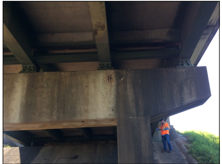
Bent 4 cap rebar exposed
