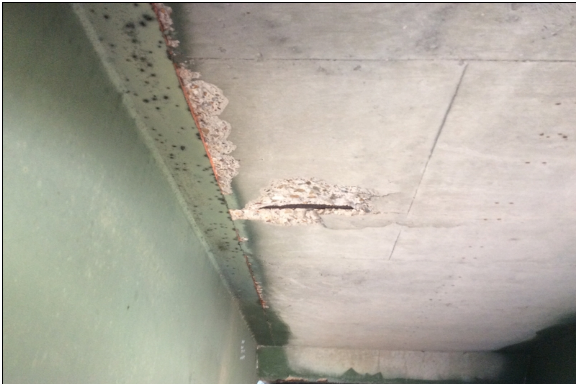
SPAN 1 SPALL WITH REBAR EXPOSED
