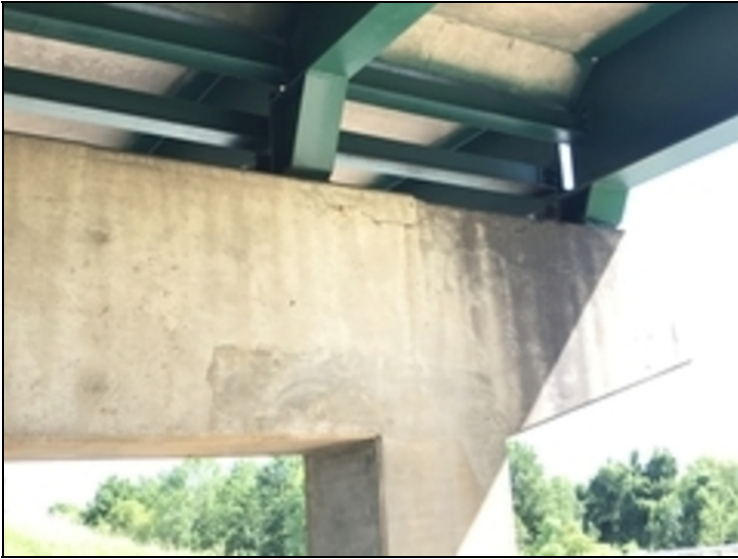
Bent 2 crack on Right side cap, under bearing, at beam 4 and 5
