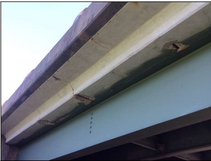
Spalls in overhangs left and right sides
