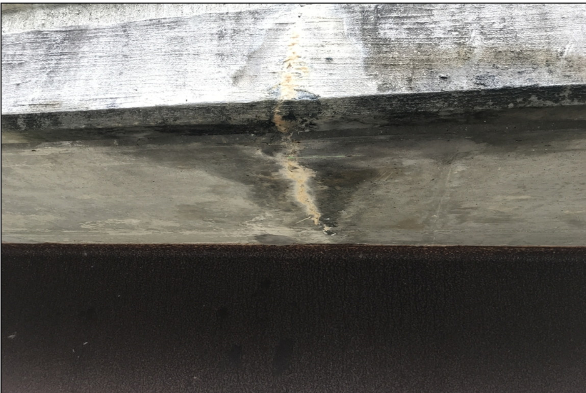
Efflorescence on the soffits with cracking
