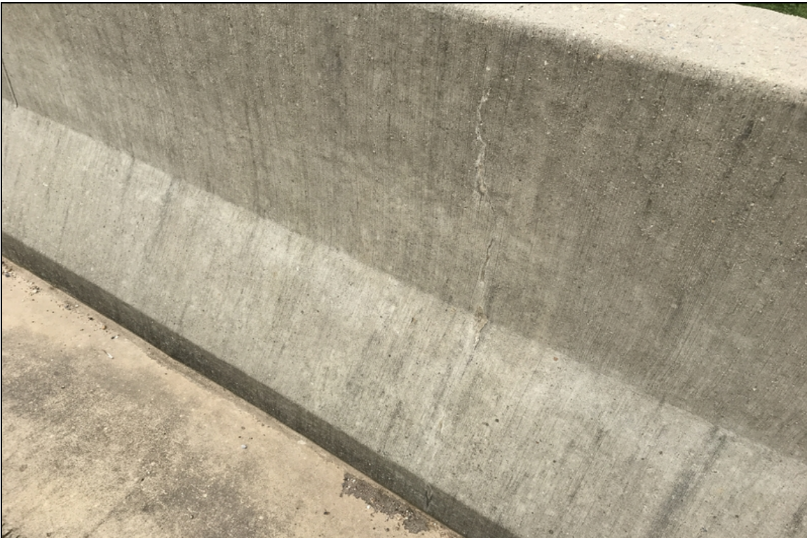
Cracks in the parapet wall
