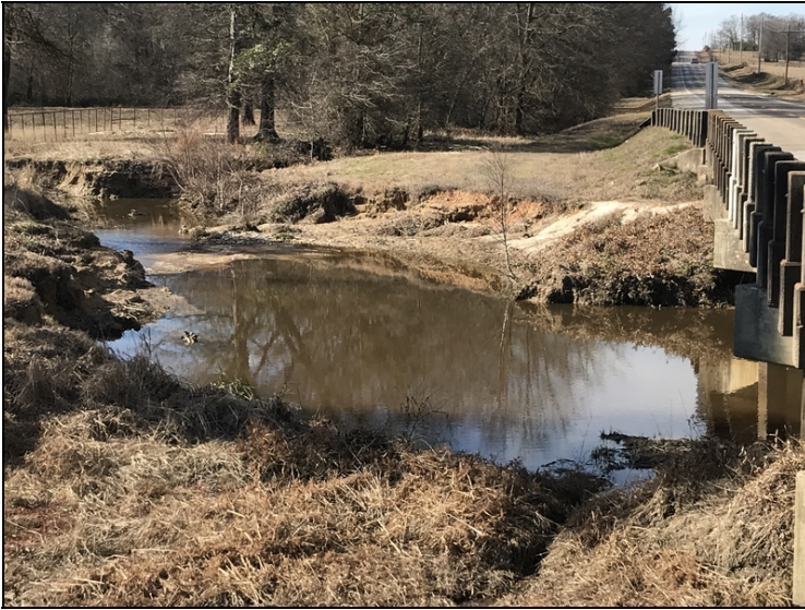
Channel erosion down stream side
