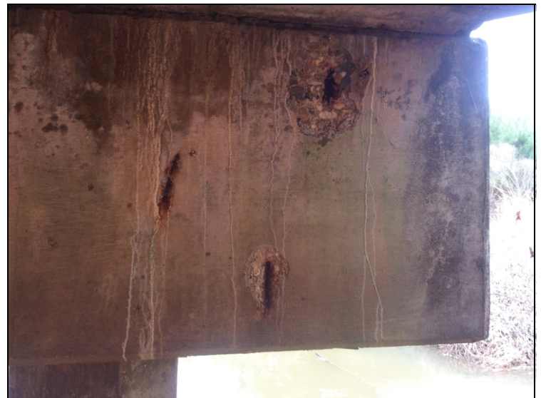
BENT 3 SPAN 3 SIDE SPALLS W/ REBAR EXPOSED
