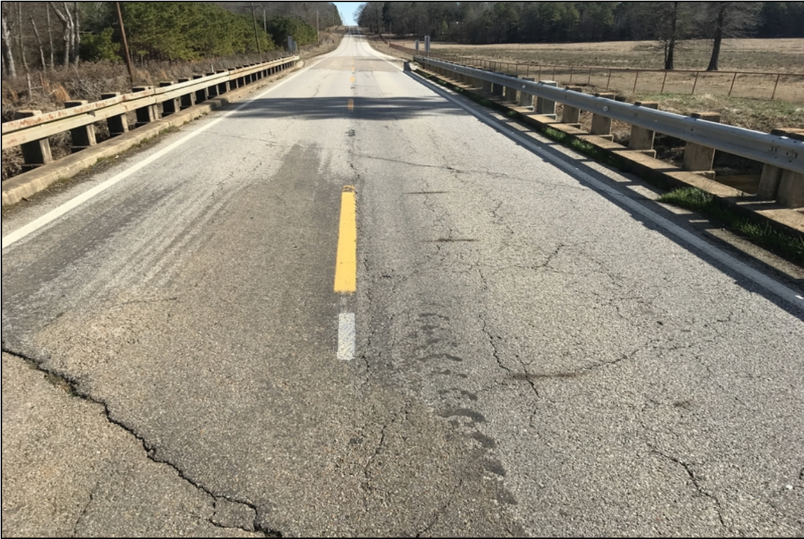
Asphalt overlay on deck is cracking
