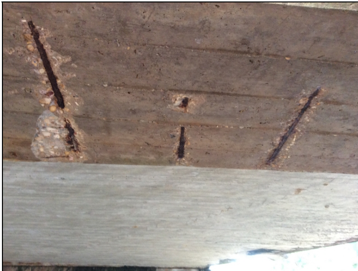
SPALLS W/ REBAR EXPOSED AT BENT 3 BOTTOM OF CAP and in span 3 left side cap
