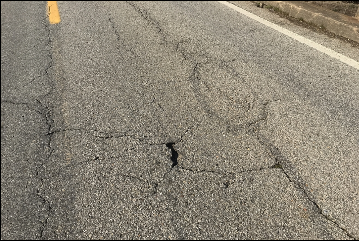
Asphalt overlay on deck
