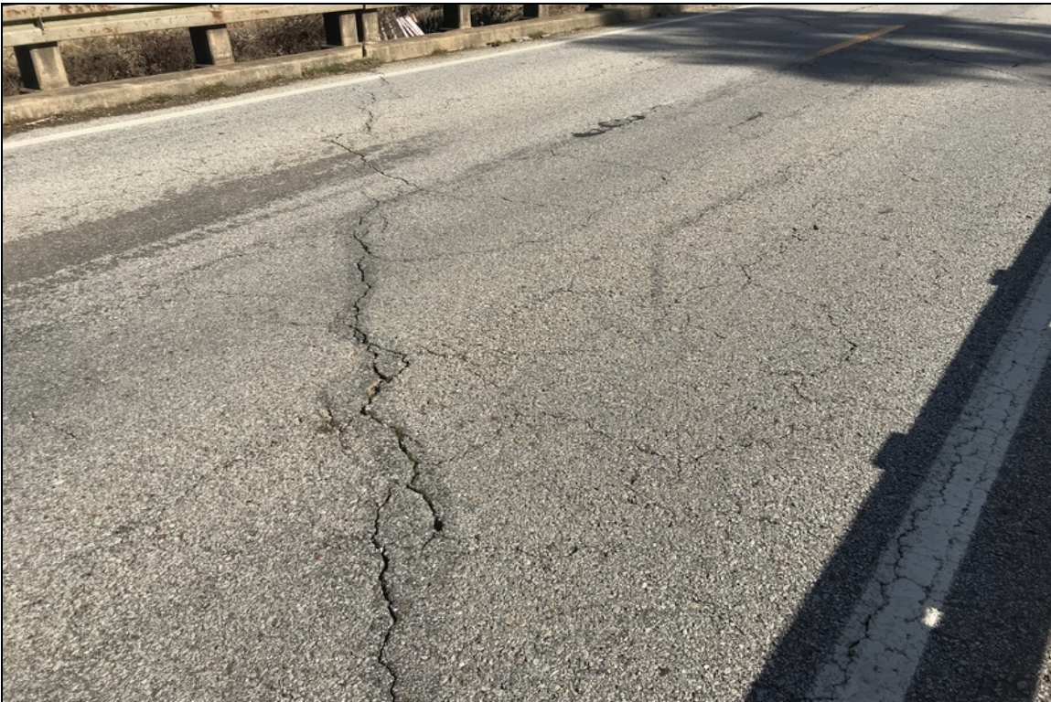
Asphalt overlay is cracking on deck
