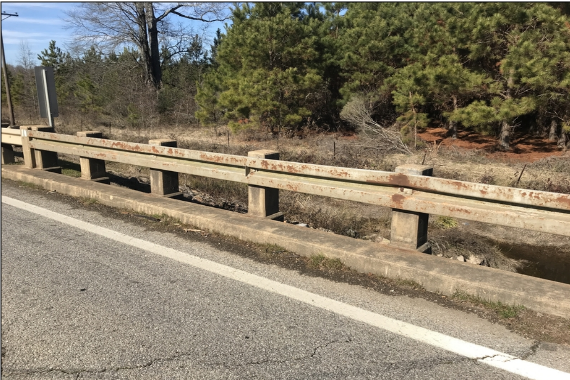
Paint loss to railings on leftside of bridge
