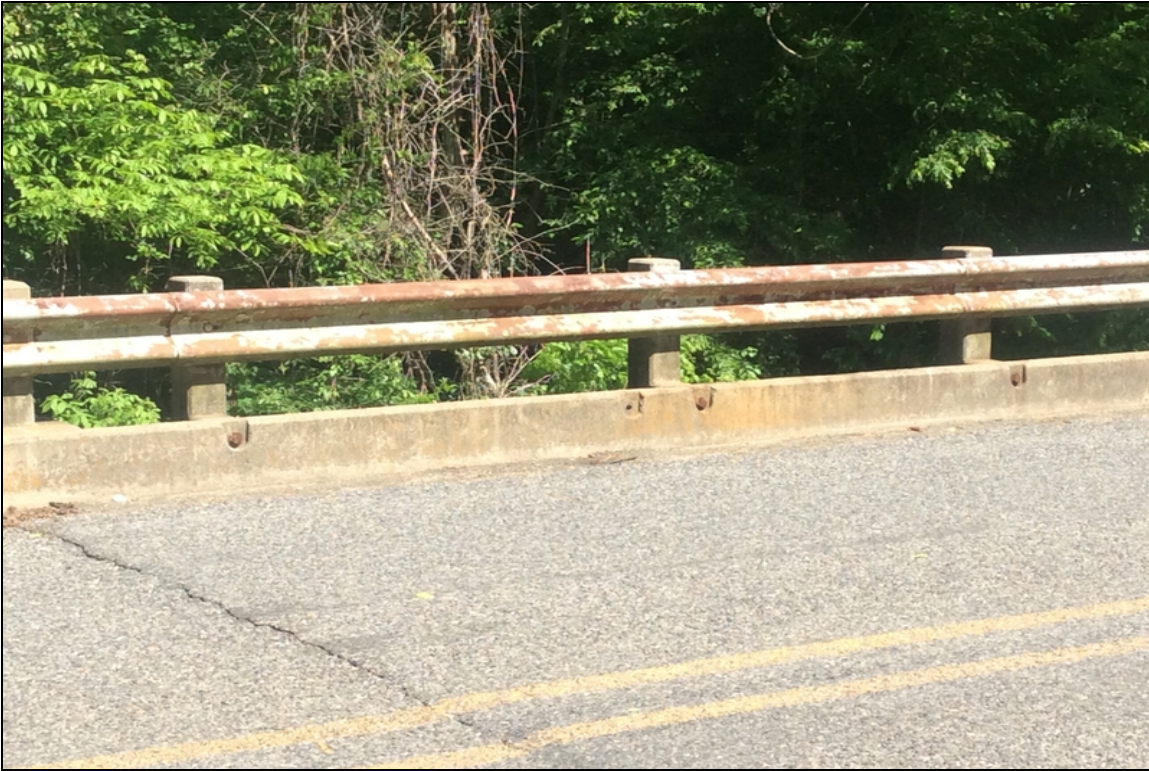
GUARD RAIL NEEDS TO BE PAINTED ENTIRE BRIDGE.
