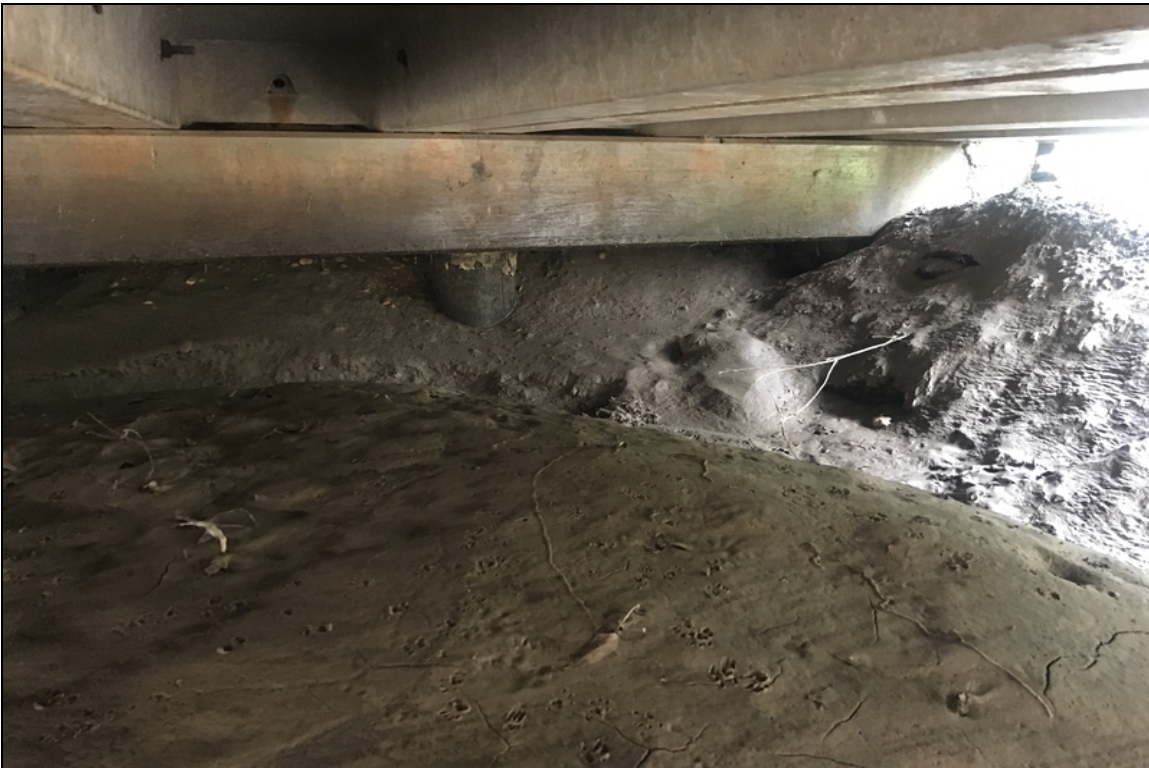
Erosion under span #1 beginning of bridge
