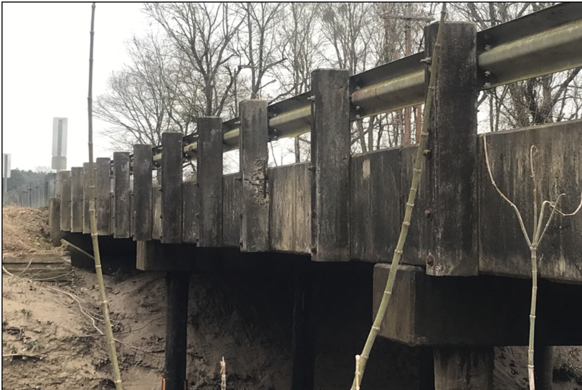
Guard rail post exposed rebar left side span #2 center post of span
