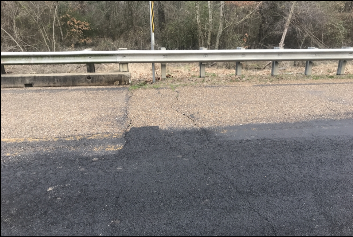
Right side of road leveled left side about an 1" low at approach on both ends of bridge
