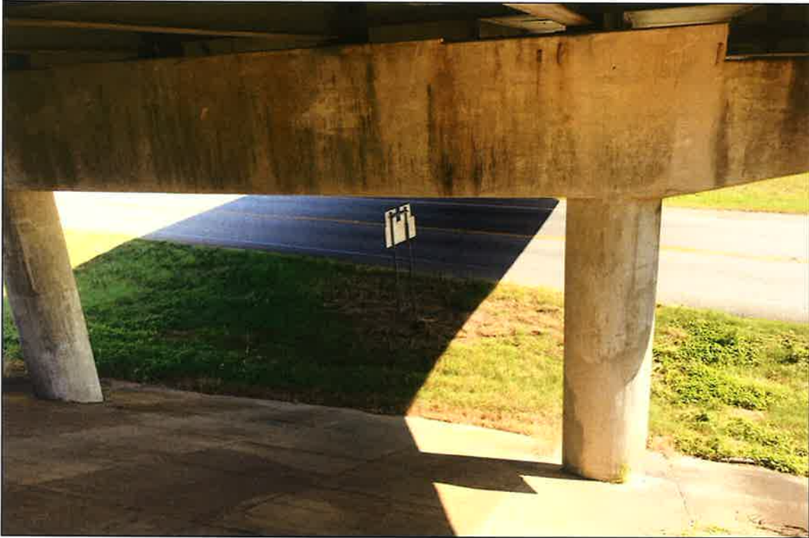
Bent 4 small crack in cap and some patch work done...
