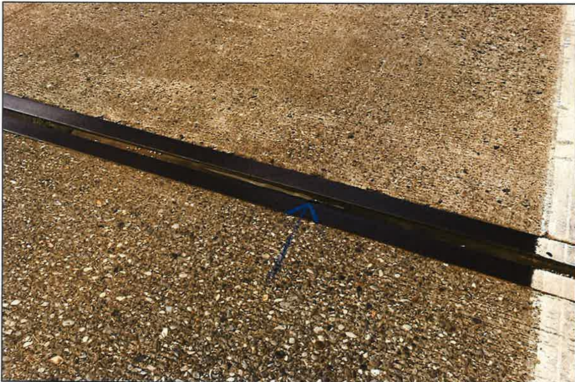
Joint 2 small hole in material....
