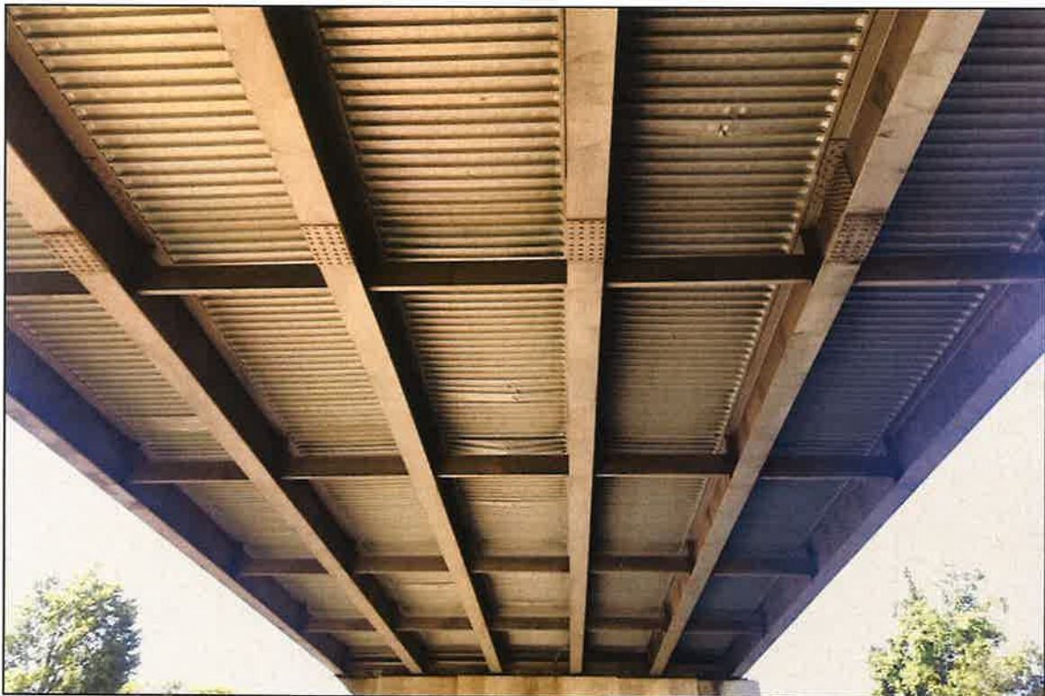
Beams sand blasted per 8/4/2020 inspection. Not painted....
