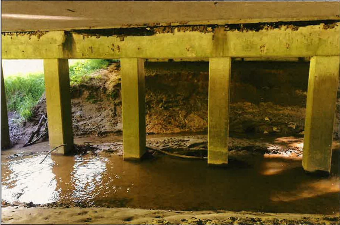
Span 3 bank slump
