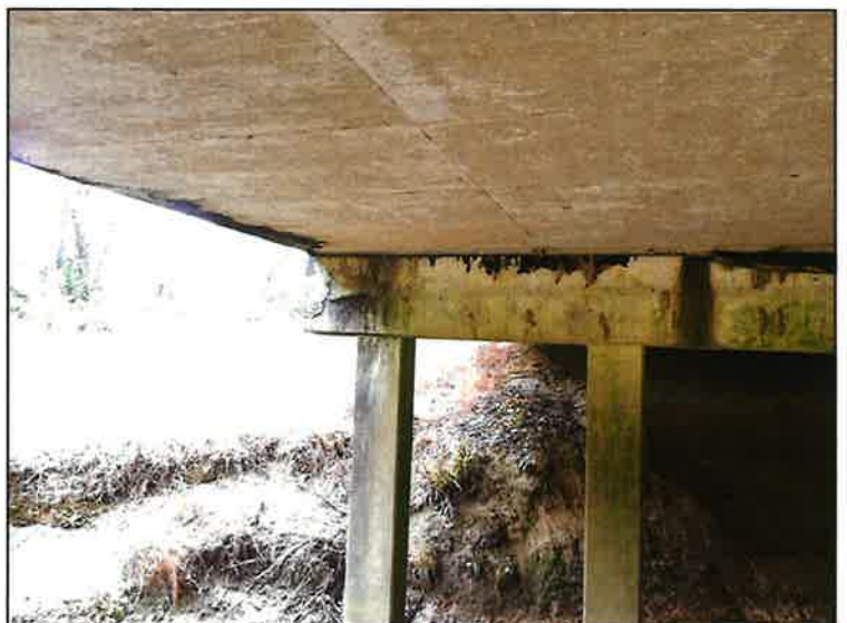
LARGE DELAM ON BT 3 LT SIDE END OF CAP
