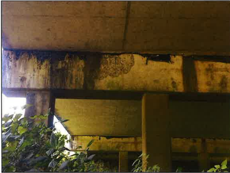
Spall with rebar exposed at bent 6
