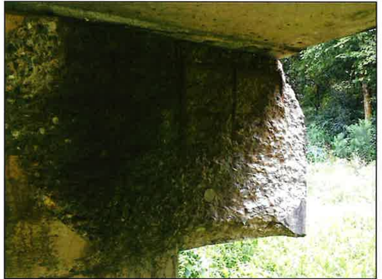
Spall at bent 7 RT side rebar exposed
