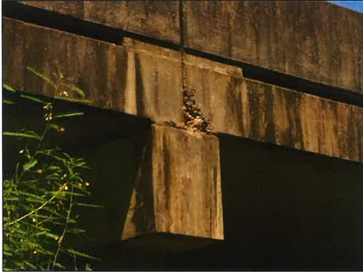
BT 5 spall in slab on the RT side
