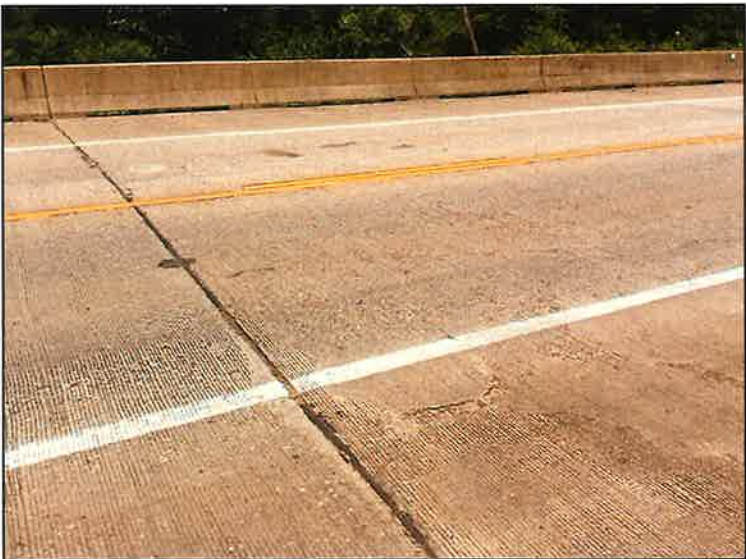
Spalls in span 4
