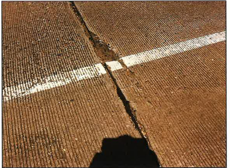
BT 5 spall in the deck
