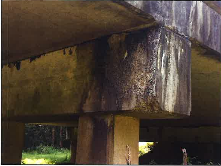
Bent 3 LT side spall with rebar exposed
