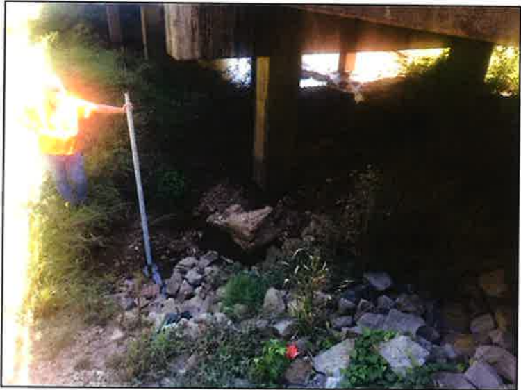
Scour hole at bent 2 left side starting...
