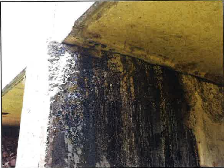
Spall with rebar exposed BT 2 RT side
