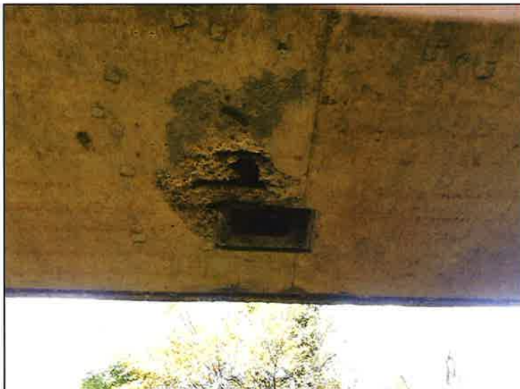
Spalls with rebar exposed at deck drains
