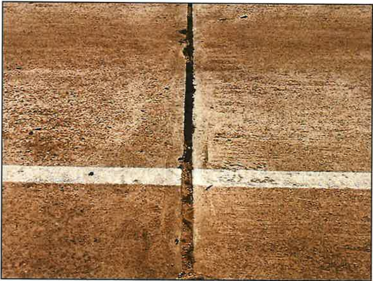
Construction joints need cleaned out and reported
