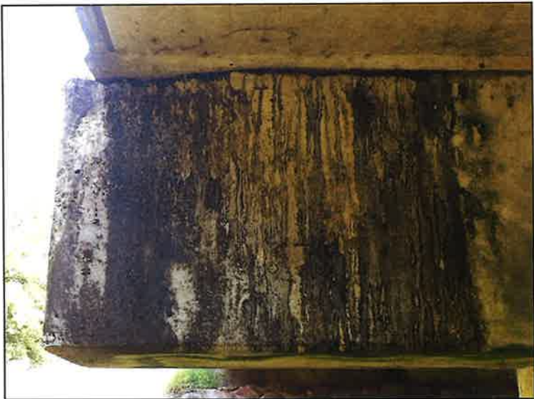
Spall with rebar exposed at bent 5 left side south face
