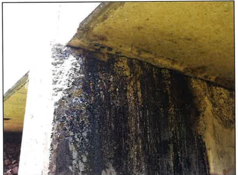
Spall with rebar exposed BT 2 RT side
