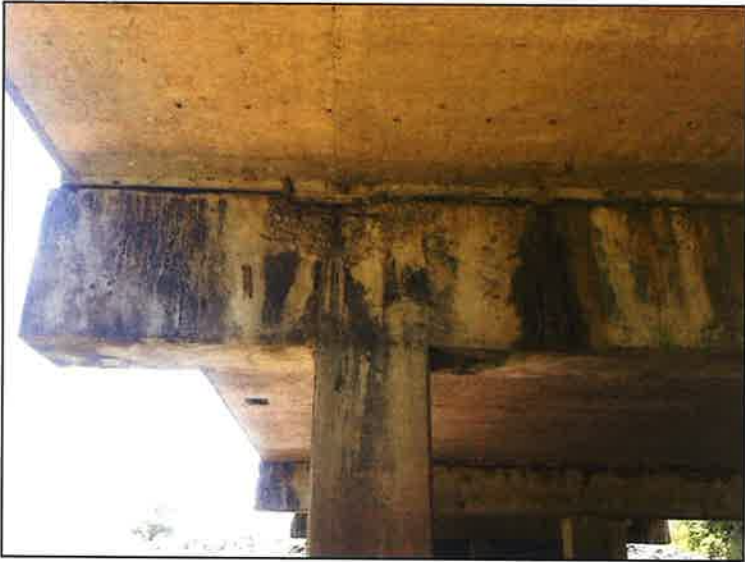
Spall with rebar exposed at bent 4 north face
