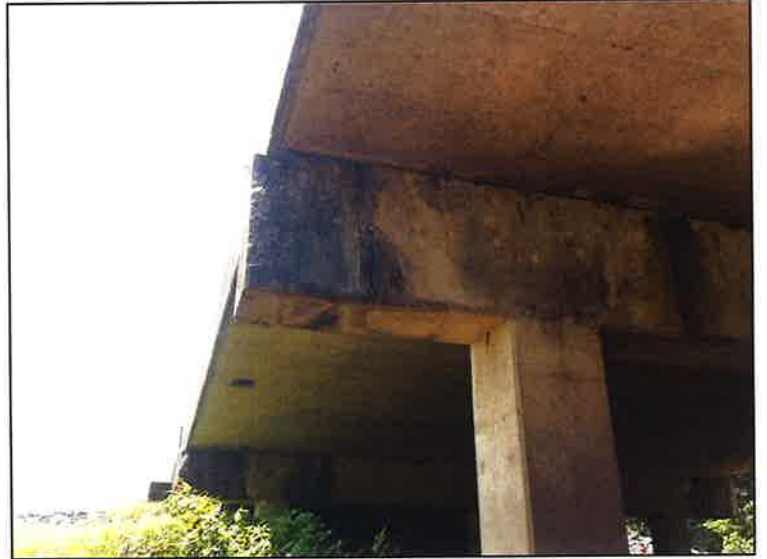
Spall with rebar exposed right side of bent 3
