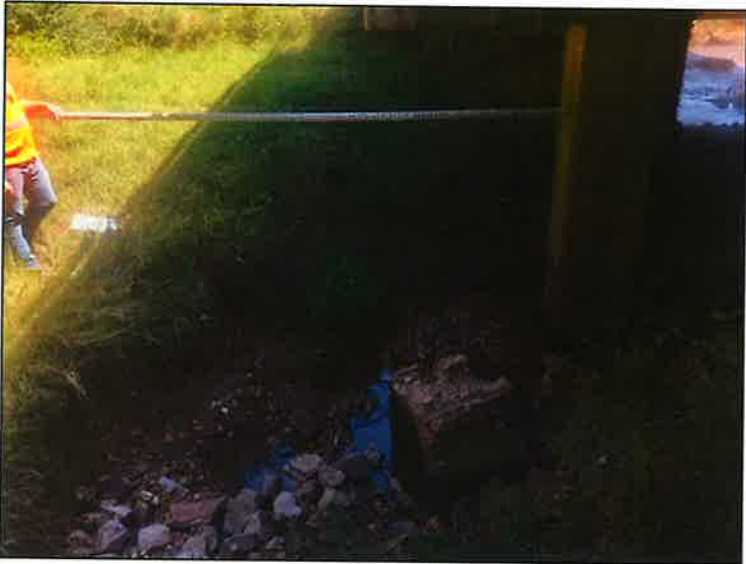
Scour hole at bent 2 left side starting...
