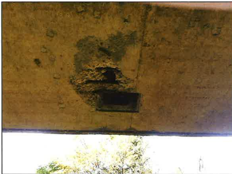
Spalls with rebar exposed at deck drains
