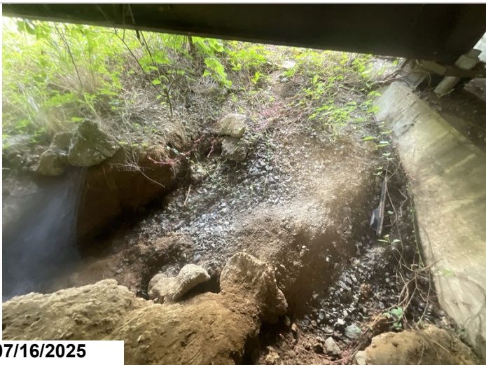
Abutment 1, under girder 5, erosion.
