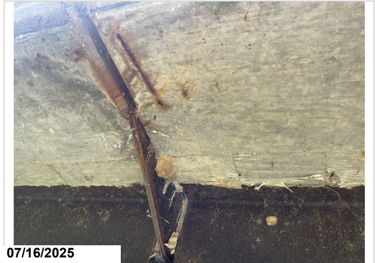
Bent 18, ahead, right overhang, exposed rebar, 2SF CS2.
