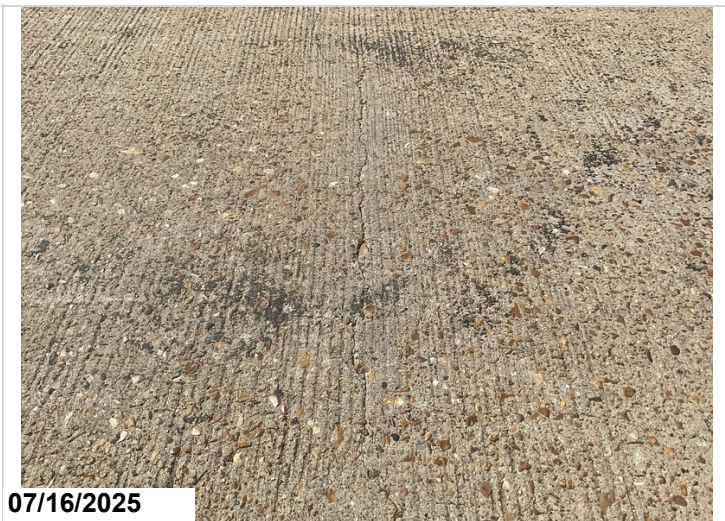
Unsealed moderate width cracks longitudinal and transverse 920 SF in CS2.
