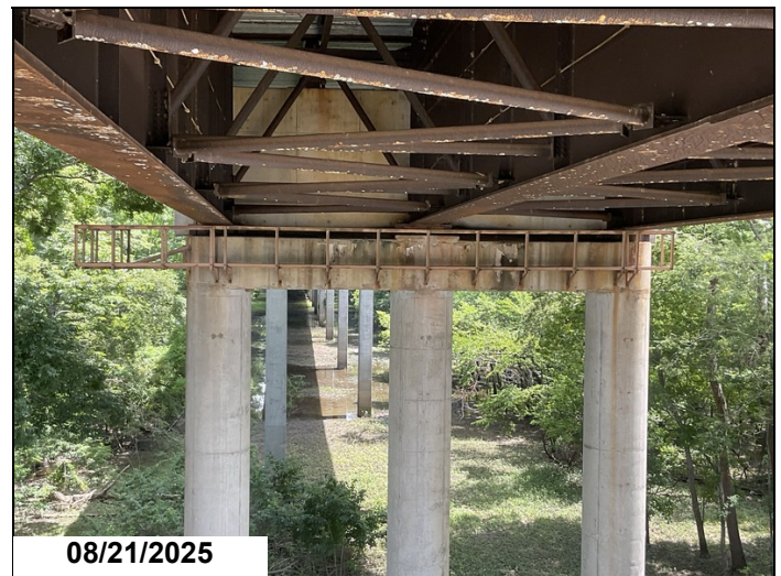
Bent 8, pier cap, cracking with efflorescence, 20LF CS3.
