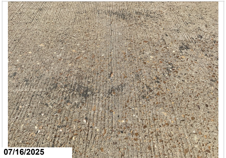
Unsealed moderate width cracks longitudinal and transverse 920 SF in CS2. photo 2.
