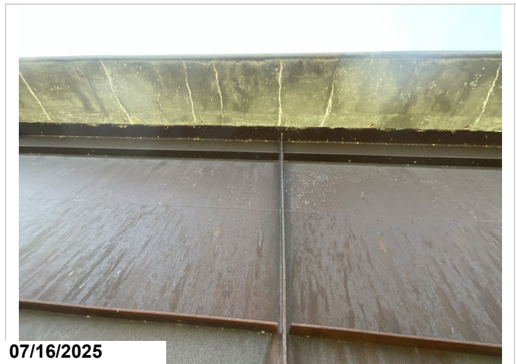
Main spans, left overhang, cracking with efflorescence, 365SF, CS2.
