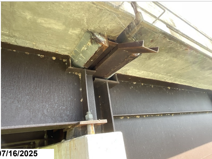
Joint system failure, Bent 6.
