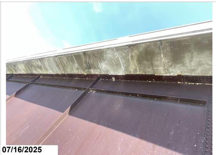
Main spans, right overhang, cracking with efflorescence, 730SF, CS2.
