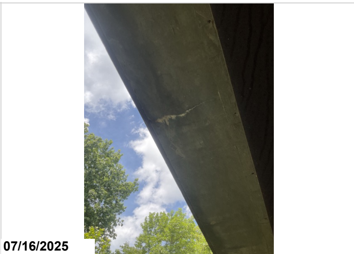
Span 12, left overhang, cracking with efflorescence, 6SF CS2. Span 12, right overhang, cracking with efflorescence, 10SF CS2.
