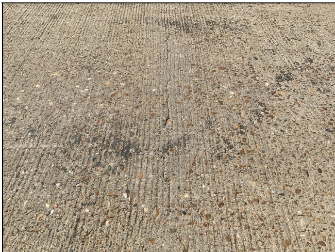
Unsealed moderate width cracks longitudinal and transverse 920 SF in CS2.
