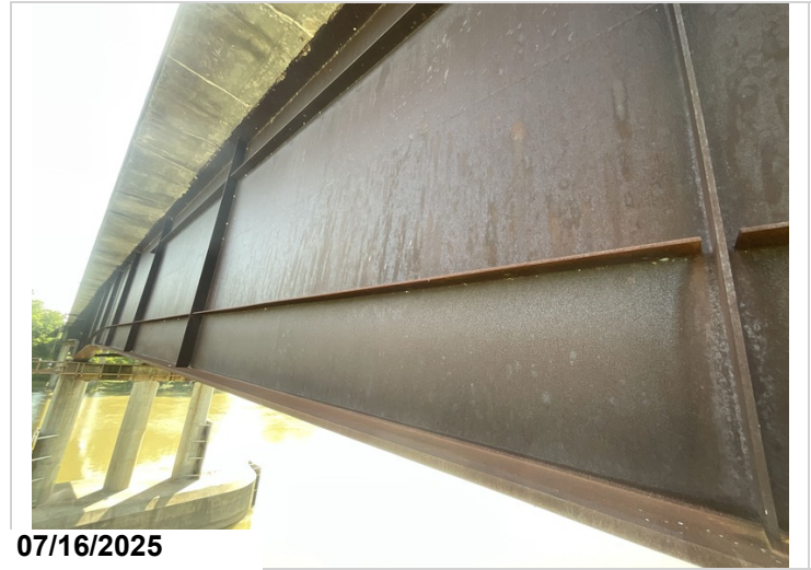
Bent1, span 6 full length falling protective coating 66,840SF CS3.
