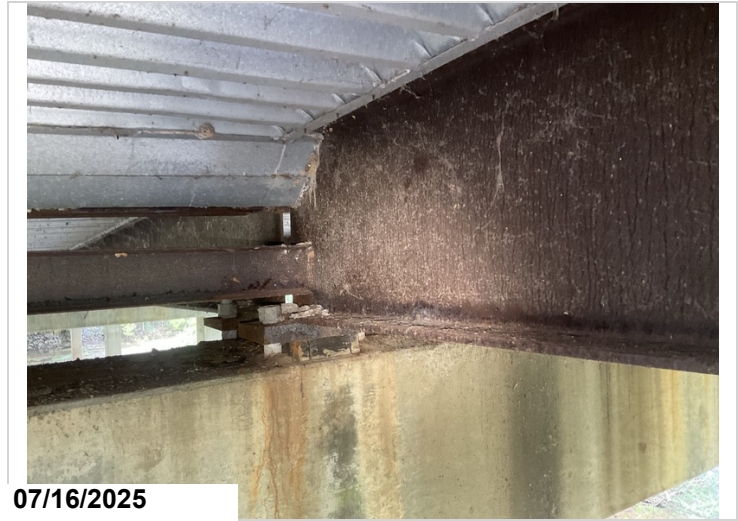
Bent 18, Span 17, girder 3, section loss, 5LF CS3.
