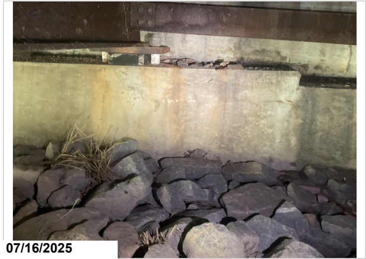
Abutment 23, Bearing 3 bearing seat cracking
