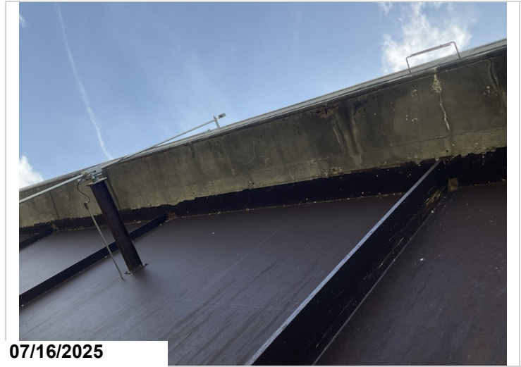
Span 7 Bent 7, spall with exposed rebar in overhang, 1SF CS2.
