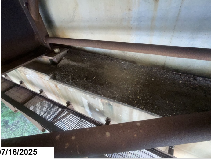
Span 7 Bent 8 cap debris buildup
