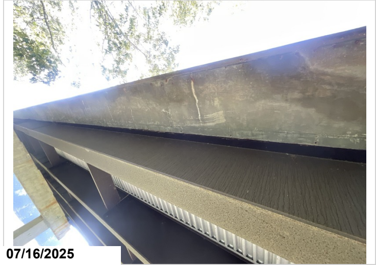
Span 3, left overhang, cracking with efflorescence, 38SF CS2. Span 3, right overhang, cracking with efflorescence, 36SF CS2.
