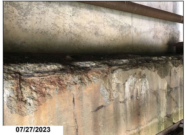
Bent 6, ahead, adjacent to bay 1, spalling with cs3 exposed reinforcing steel.
