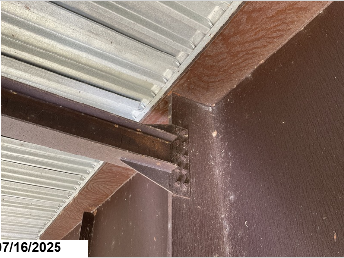
Bent 7, floor beam connector, loose bolts can't reach with Aspen A62T.
