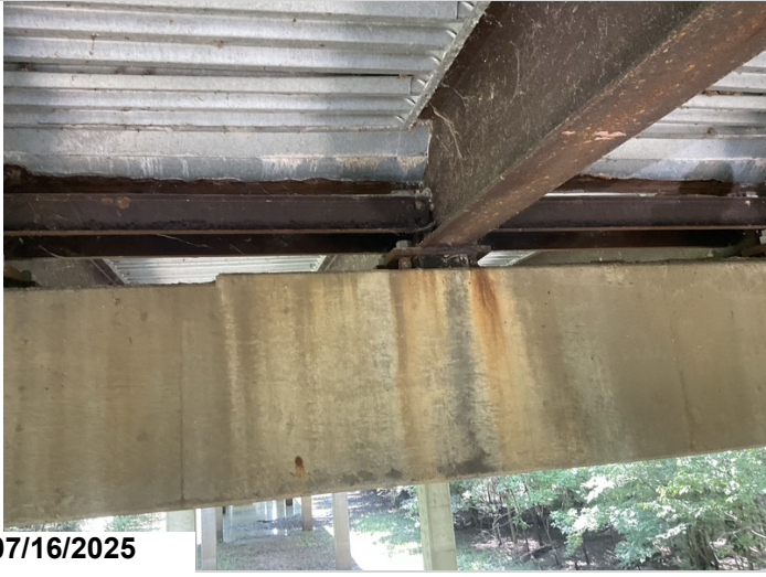
Bent 18 ahead bearing 1-6 sole plate and diaphragm corroded.
