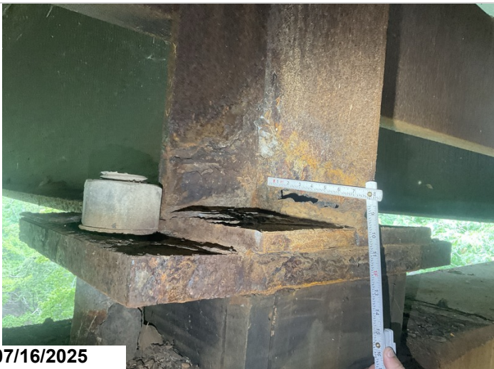
Bent 8, Span 8, girder 4, section loss beam end hole 1" x5" hole 1LF CS3.
