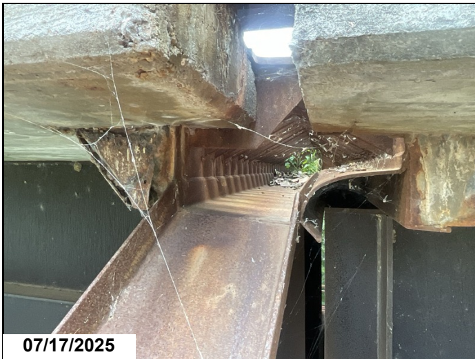
Bent 8, Joint seal failure
