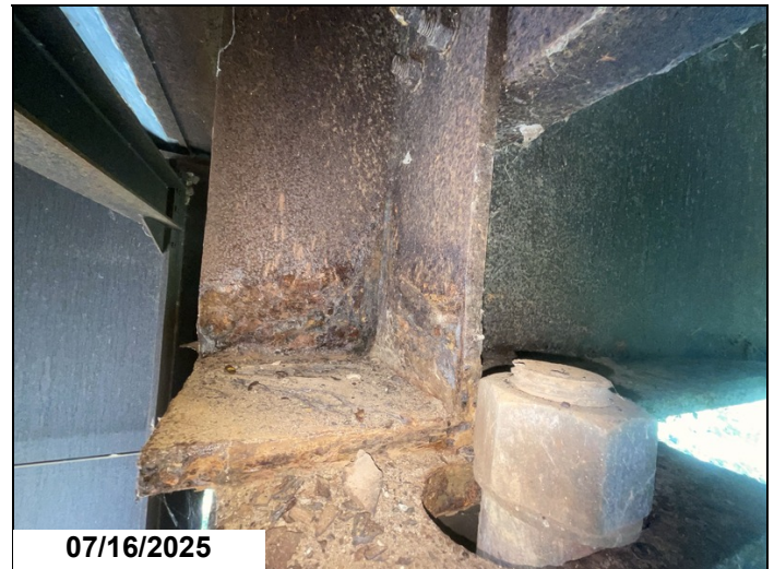
Span 7, Bent 8, Girder 2, beam end section loss up to 1/8" to web, 3LF CS3.
