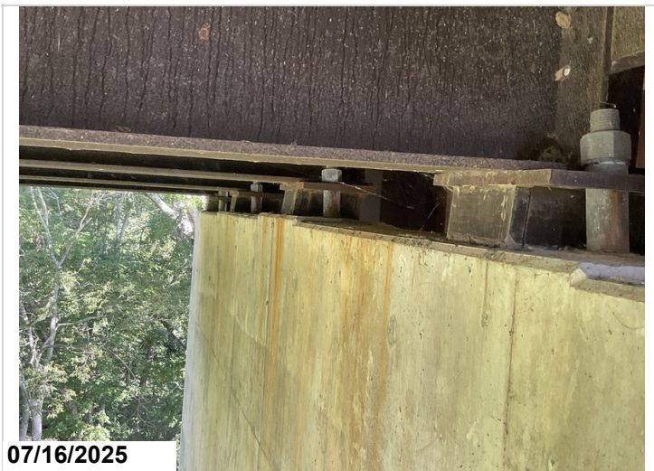
Bent 6 girder bearing distortion.
