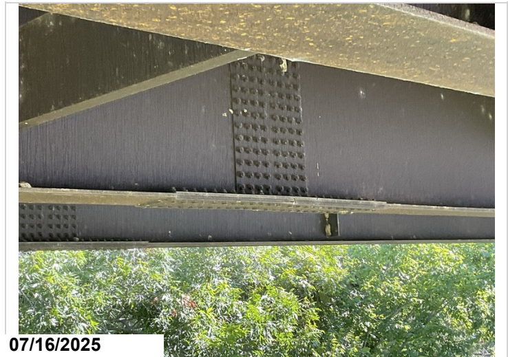
Span 5 girder 2 splice plate bottom flange, pack rusting, 1LF CS3.
