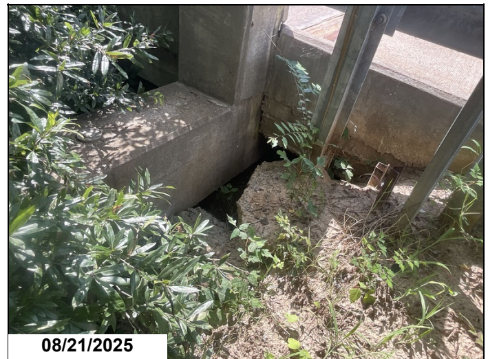
Abutment 23, right, undermining of approach slab.
