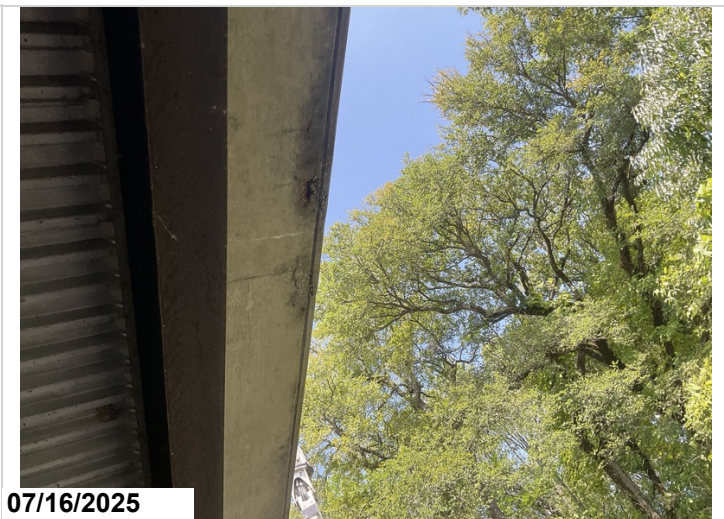
Span 17 right overhang, exposed rebar, 1SF CS2, cracking with efflorescence, 1SF CS2.
