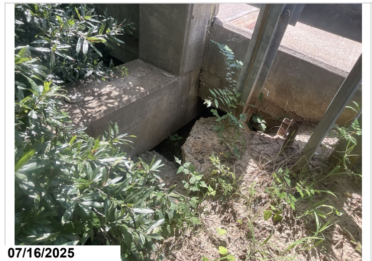
Abutment 23, right, undermining of approach slab.
