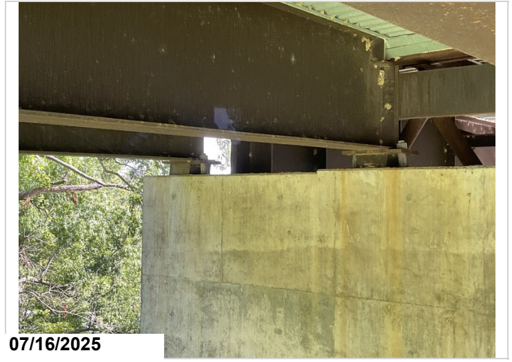
Bent 6 girder 1 out of plane distortion.
