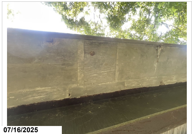
Span 17 left overhang, exposed rebar, 1SF CS2, cracking with efflorescence, 1SF CS2.
