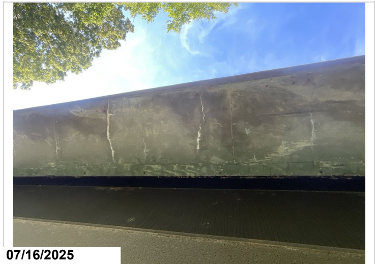
typical cracking with efflorescence in overhangs.
