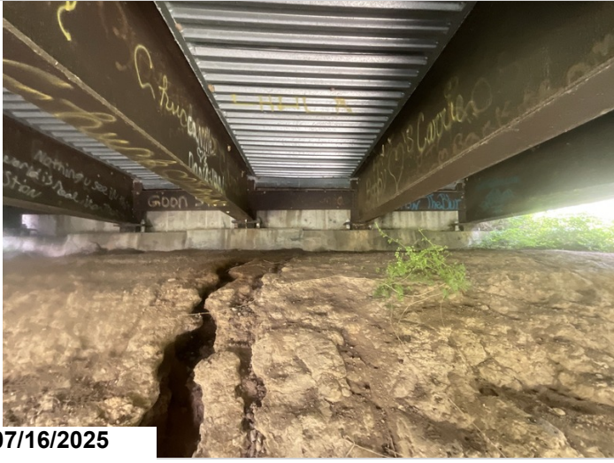
Abutment 1, erosion in the embankment under bay 2 and 3
