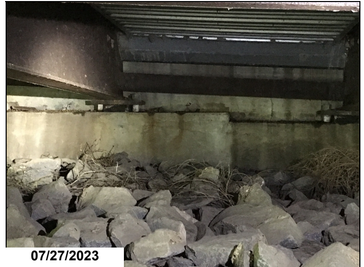
Bent 23, bridge seat, 10' horizontal cracking.
