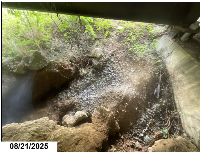
Abutment 1, under girder 5, erosion.
