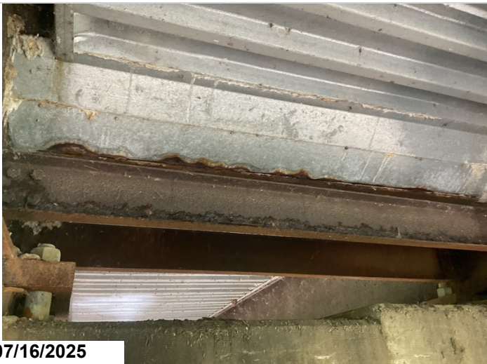
Bent 18 typical diaphragm corrosion.
