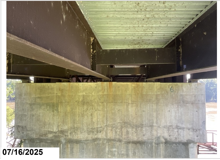
Bent 6 overview of bearing out of plane distortion.
