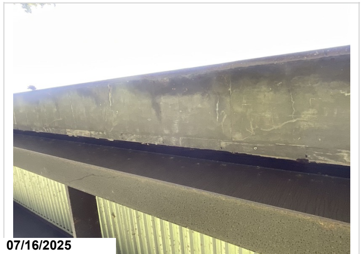
Span 4, left overhang, cracking with efflorescence, 20SF CS2. Span 4, right overhang, cracking with efflorescence, 32SF CS2.
