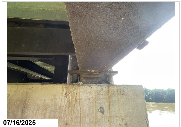
Bent 6 girder 5 bearing distortion.
