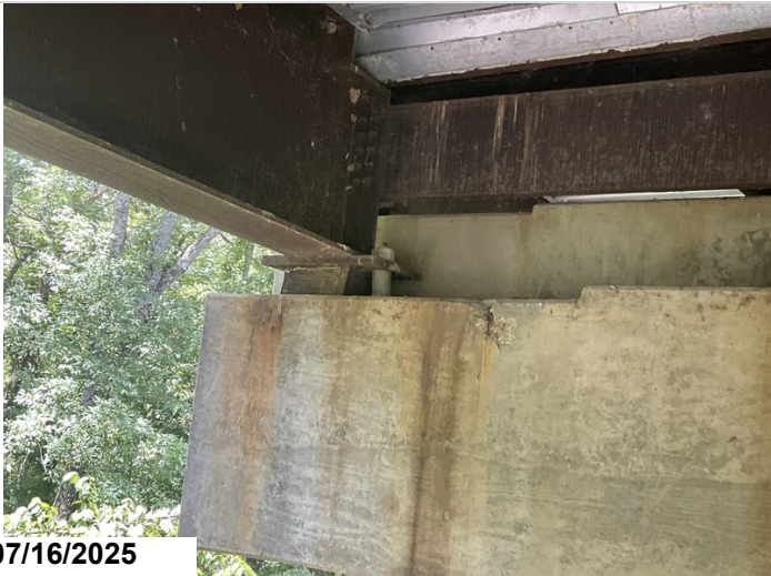
Typical condition of bearing misalignment on Bent 13, back, girder 1,3,4,5.
