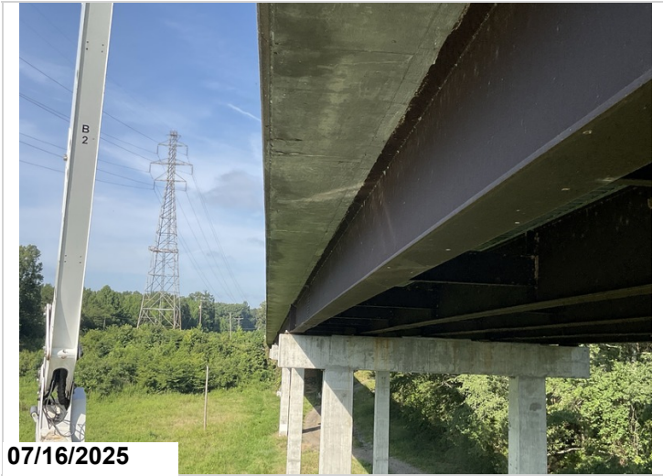
Span 5, mid span right overhang spall with exposed rebar, 2SF CS2.
