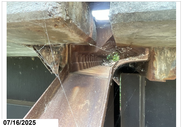
Bent 8 debris impaction
