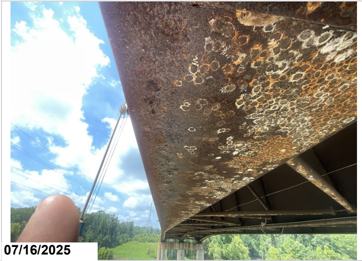
Span 7, pier 2 bottom flange of all girders, flaking rust, 9,855SF CS3.
