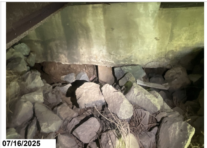
Abutment 23, undermining under girder 4, full depth, 5 feet wide.
