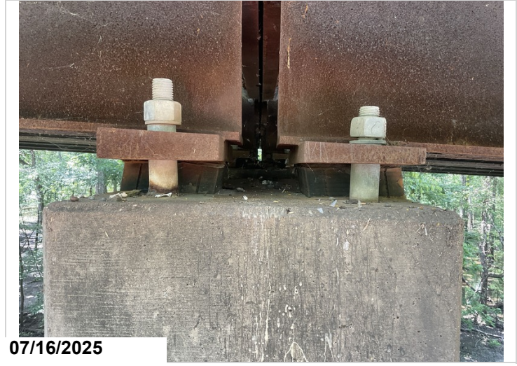
Bent 18 bearings misalignment.
