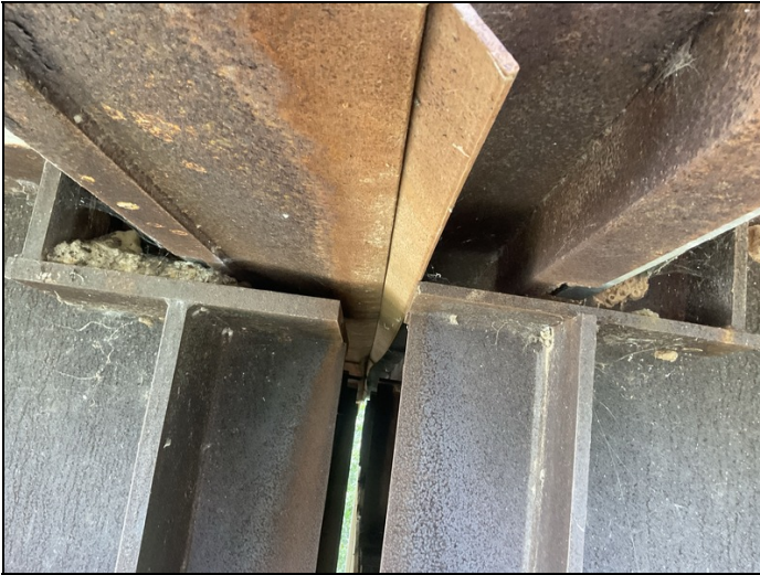
Bent 8 joint seal failure.
