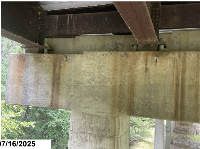
Bent 13, back, pier cap, exposed rebar, 2LF CS2, cracking with efflorescence, 1LF CS2.
