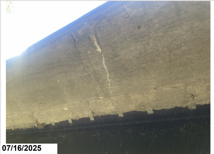
Span 18, left overhang, cracking with efflorescence, 2SF CS2. Span 18, right overhang, cracking with efflorescence, 4SF CS2.
