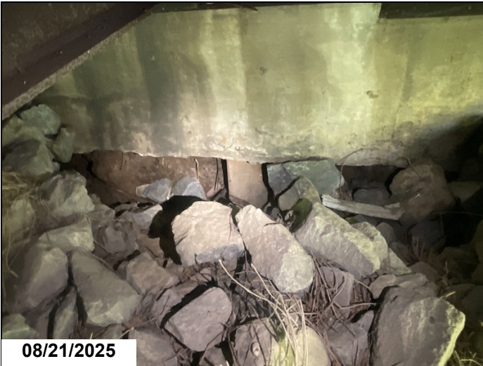
Abutment 23, undermining under girder 4, full depth, 5 feet wide.
