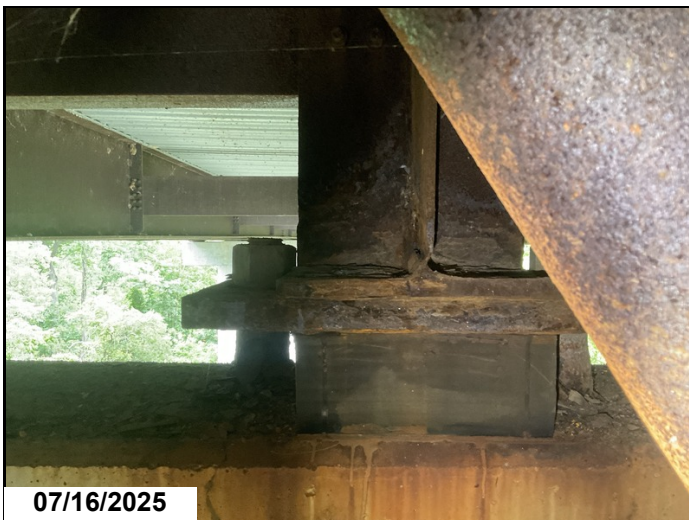
Span 7, Bent 8, Girder 4, section loss beam end hole with crushing action 1" x5" hole 1LF CS3.(CF)
