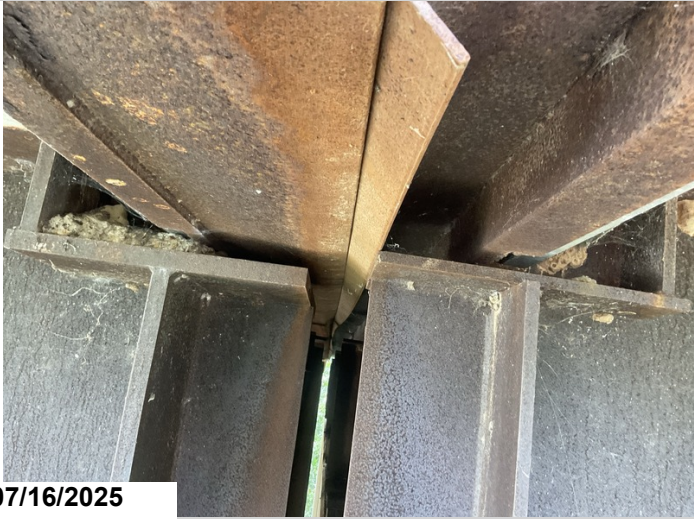
Bent 8 joint seal failure.
