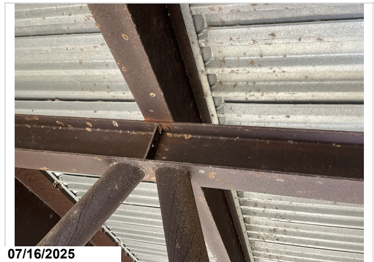
Bent 7, floor beam and stringer connection has loose bolt can't reach with Aspen A62T.
