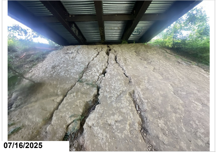
Abutment 1, erosion in the embankment under bay 2 and 3
