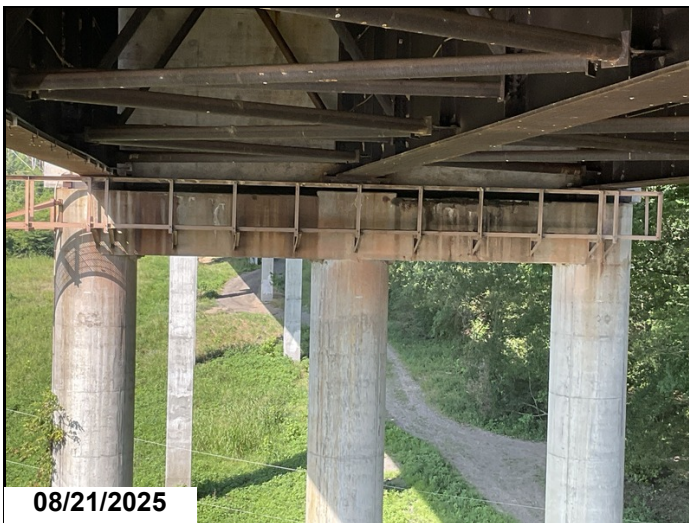
Bent 6 ahead, spalling with exposed rebar, 10LF CS2.
