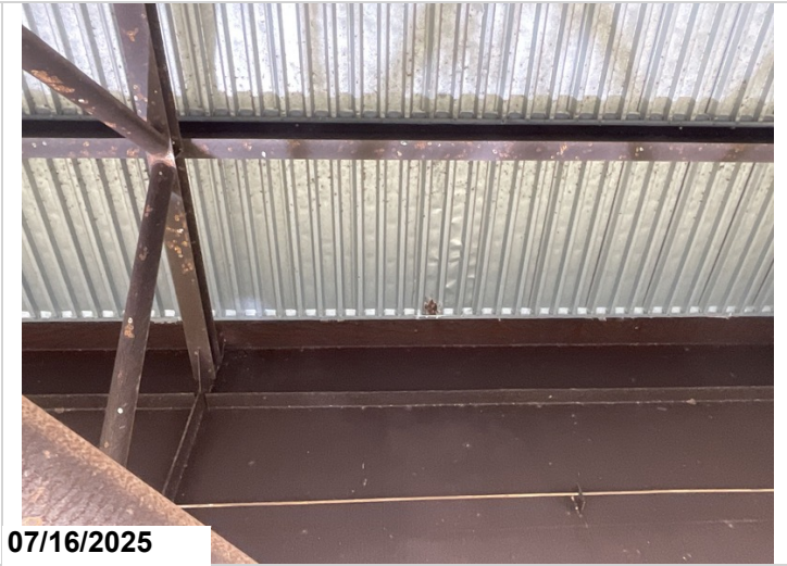
span 7 mid span, corrosion in deck pan.
