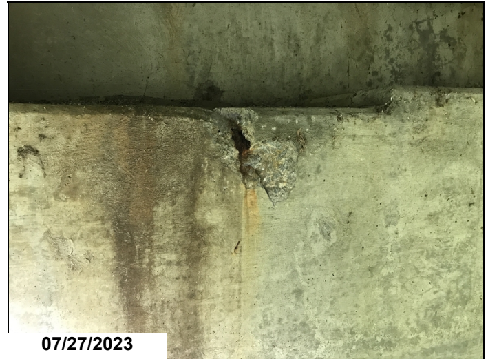
Bent 13, back, adjacent to girders 1 & 2, spalling with exposed reinforcing steel. 2ft.
