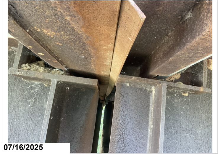
Bent 8 joint seal failure.
