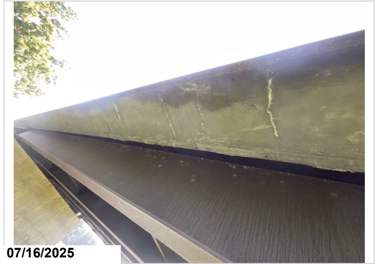
Span 5, left overhang, cracking with efflorescence, 16SF, CS2. Span 5, right overhang, cracking with efflorescence, 24SF, CS2.
