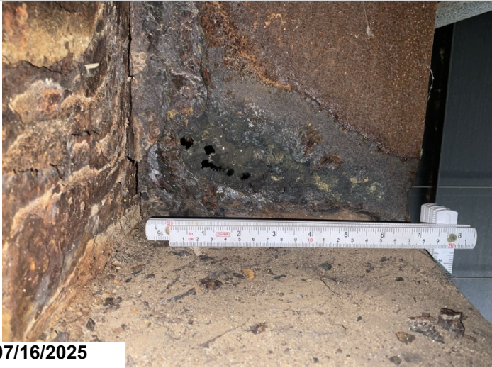
Bent 8, Span 8, girder 3, beam end section loss up to 1/2" to web 3LF CS3 1"x3" hole
