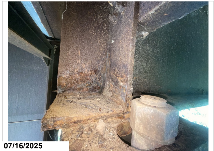
Bent 8, Span 8, girder 2, beam end section loss up to 1/8" to web, 3LF CS3.
