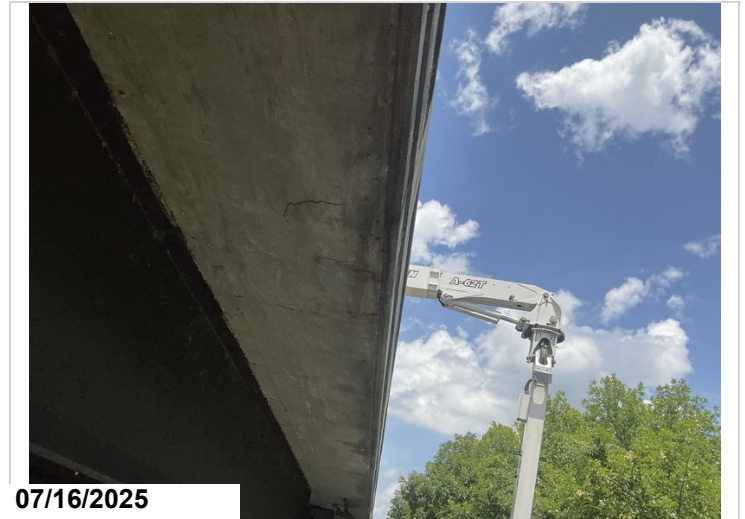
Span 12, right overhang, delaminated area, 2SF CS2.
