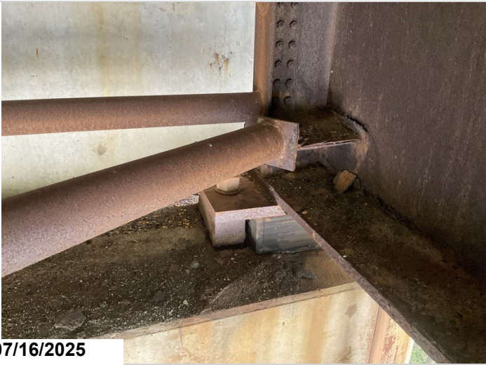
Bent 8, span 7, girder 3, laminating rust on bottom flange, 10LF CS3, laminating rust on web above flange 10LF CS3.
