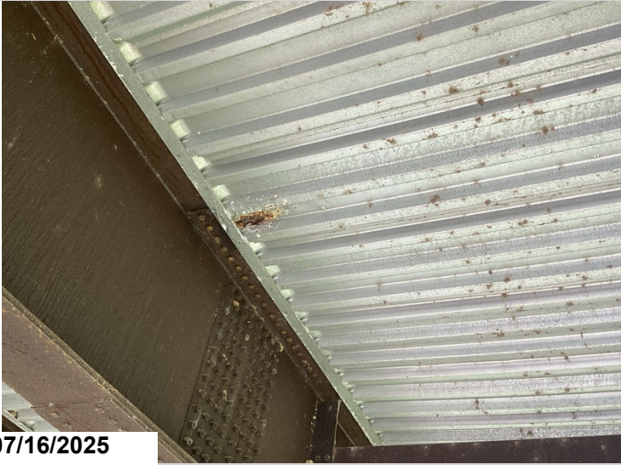
Span 3 bent 4 back, corrosion in deck pan.
