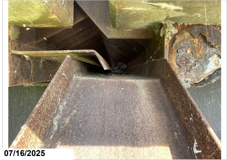
Bent 6 joint, debris impact, full width, CS2.
