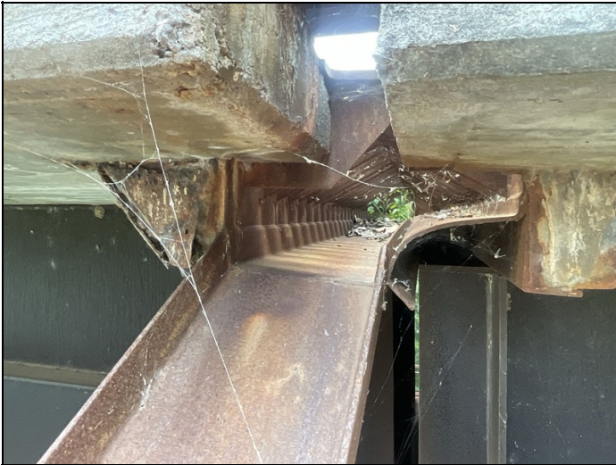
Bent 8 debris impaction
