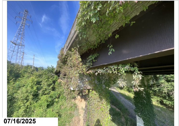
Bent 2 vegetation buildup
