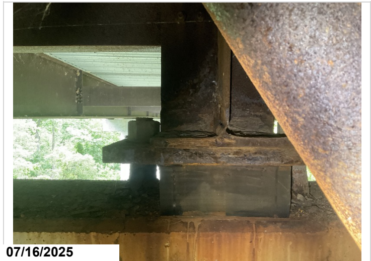
Bent 8, Span 8, girder 4, section loss beam end hole 1" x5" hole 1LF CS3.
