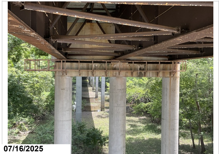
Bent 8, pier cap, cracking with efflorescence, 20LF CS3.
