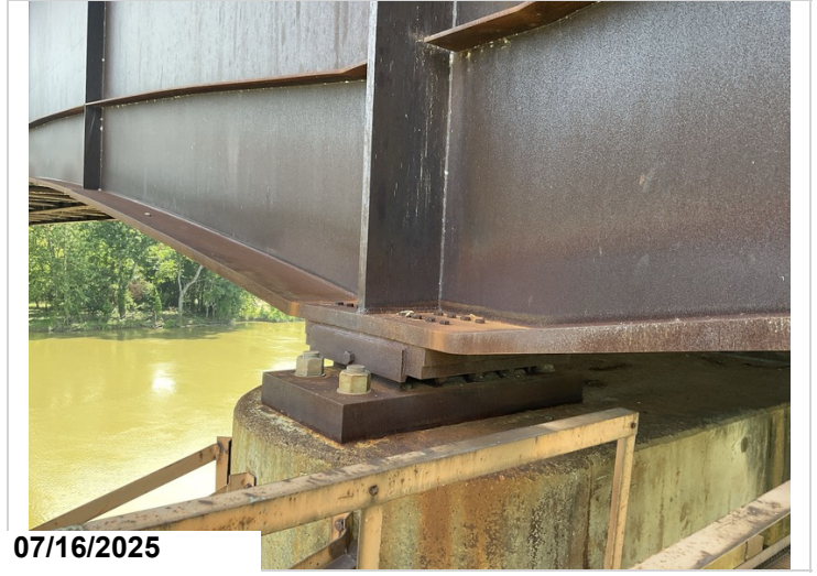
Typical condition of bearing at Bent 7.
