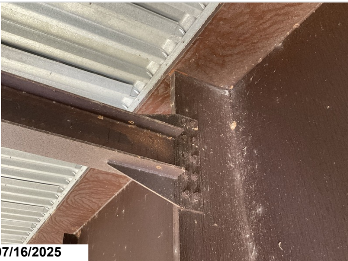
Bent 7, girder 2 right, stiffener above bent, fretting rust.
