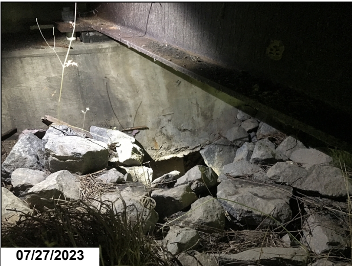
Bent 23, adjacent to girder 5, undermining 3' wide by 2' deep, exposing a pile.
