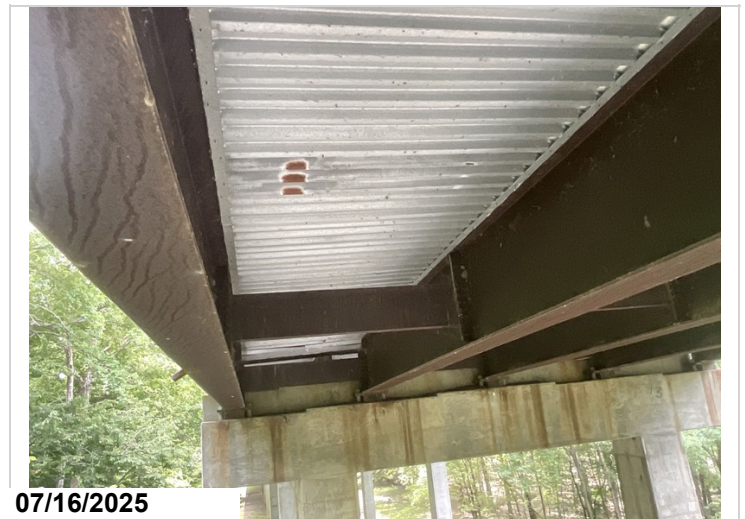
Deck pan corrosion in bay 1 span 12.
