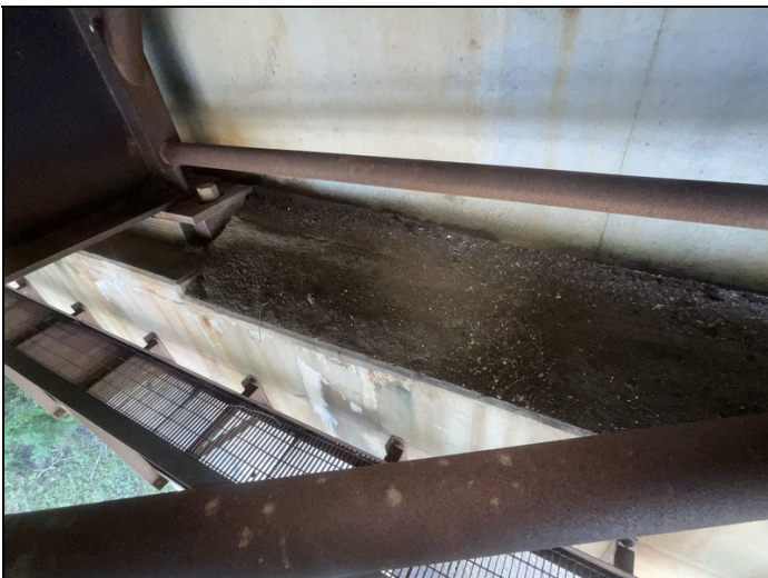
Span 7 Bent 8 cap debris buildup
