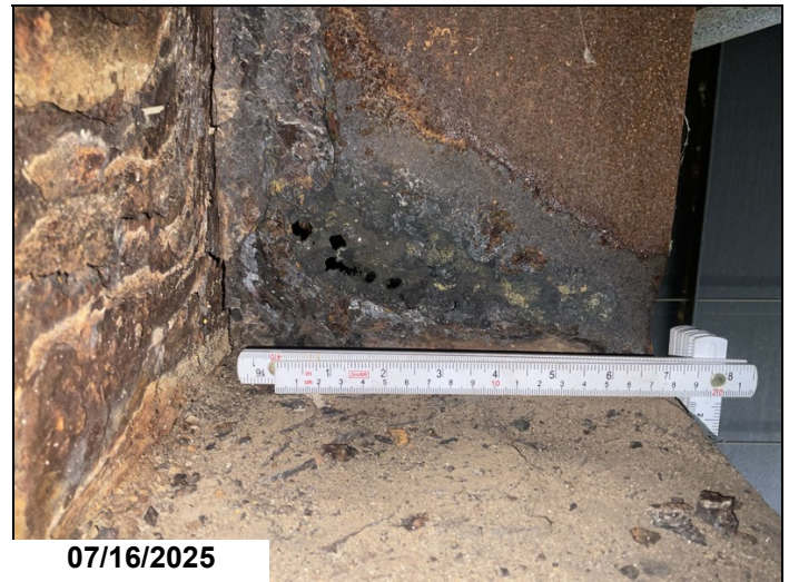
Span 7, Bent 8, girder 3, beam end with crushing action section loss up to 1/2" to web 3LF CS3 1"x3" hole.(CF)
