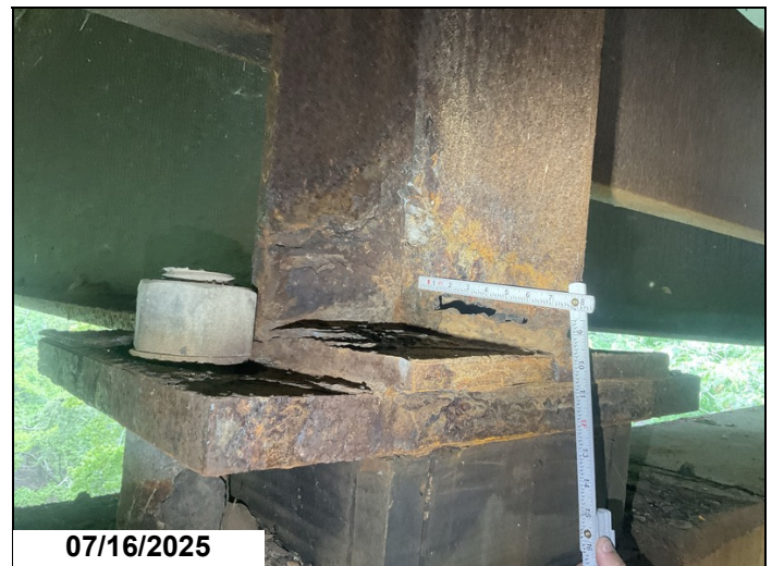
Span 7, Bent 8, Girder 4, section loss beam end hole 1" x5" hole 1LF CS3. Photo 2
