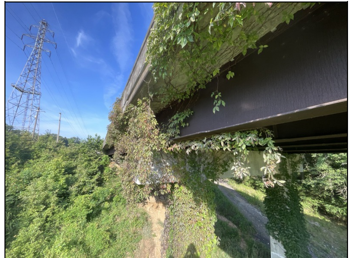
Bent 2 vegetation buildup
