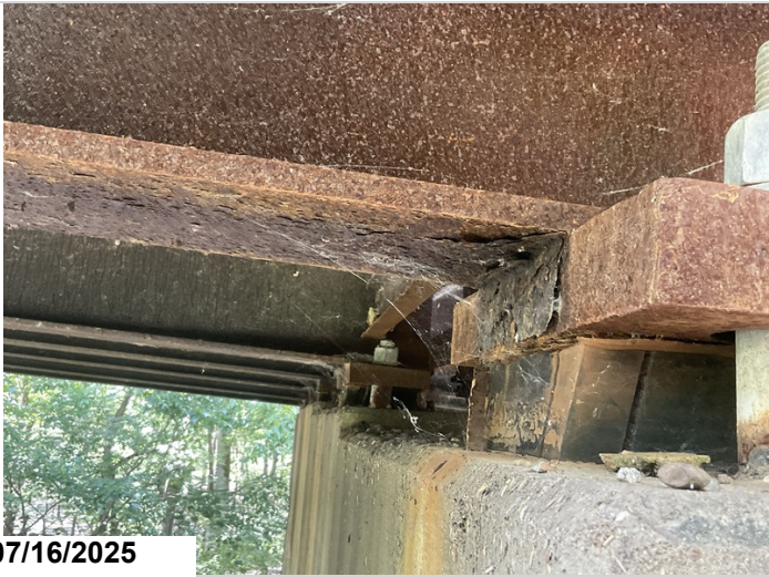
Bent 18, span 17, girder 4 and 5, bottom flange, corrosion, 4LF CS2.
