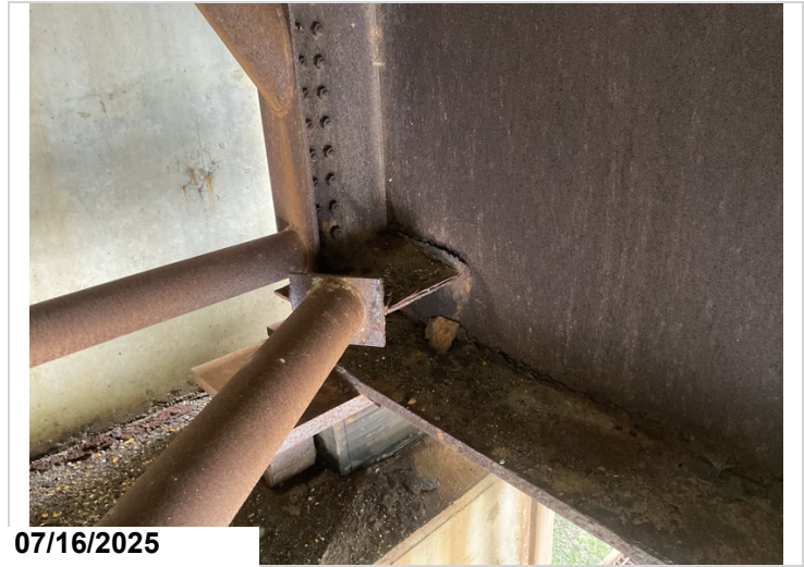
Bent 8, span 7, girder 3, laminating rust on bottom flange, 10LF CS3, laminating rust on web above flange 10LF CS3.
