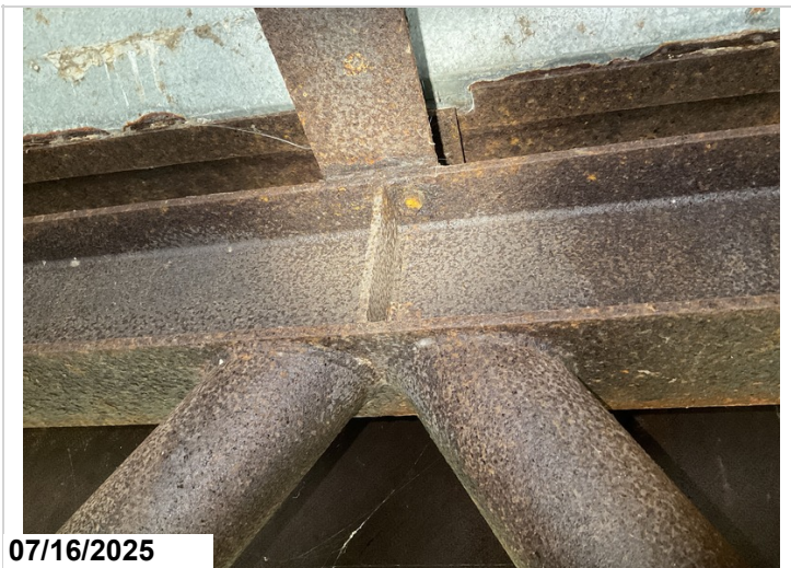
Span 7 bent 8 stringer/floor beam connection area corrosion around bolt.
