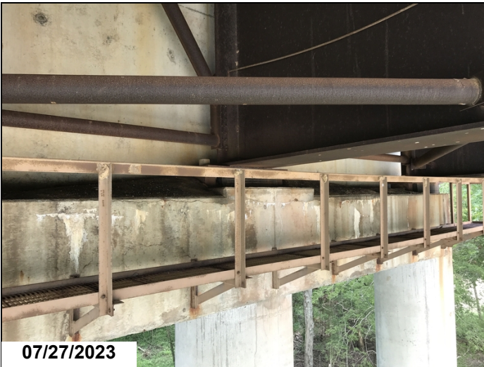
Bent 8, back, 15' of cracking with cs3 efflorescence. 7' of cs2 cracking.
