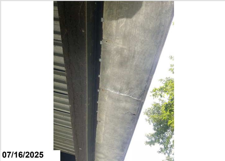
Span 13, left overhang, exposed rebar, 1SF CS2, cracking with efflorescence, 4SF, CS2. Span 13, right overhang, cracking with efflorescence, 4SF, CS2.
