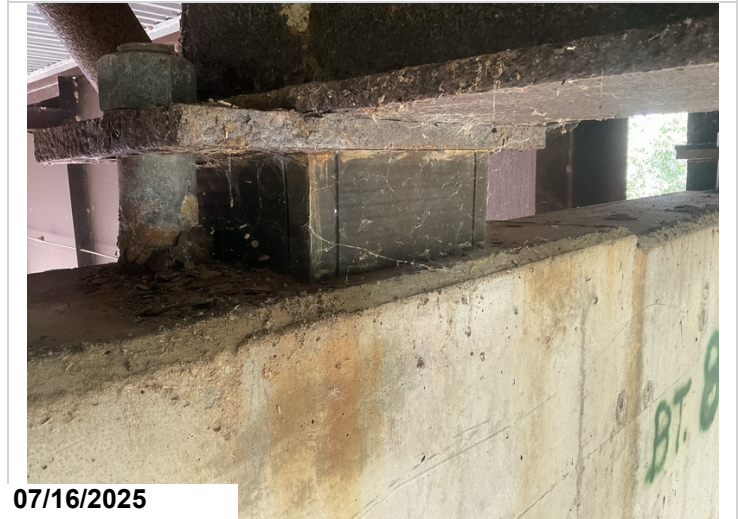
Bent 8 typical bearings.
