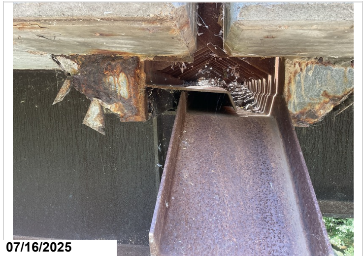
Bent 13 joint debris impaction.
