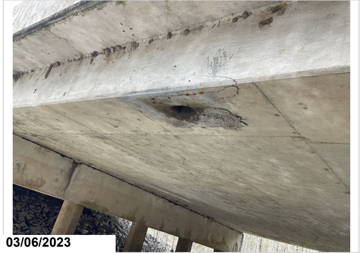
Span 2 right at midspan at drain opening has cracking and delams.
