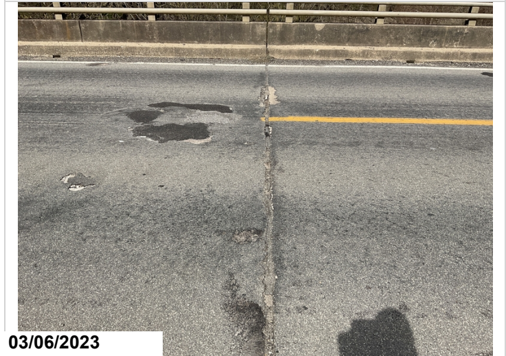
Bent 3 joint seal has debris impaction.
