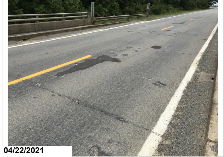
Wearing surface - Span 1 left: Spalling (potholes)
