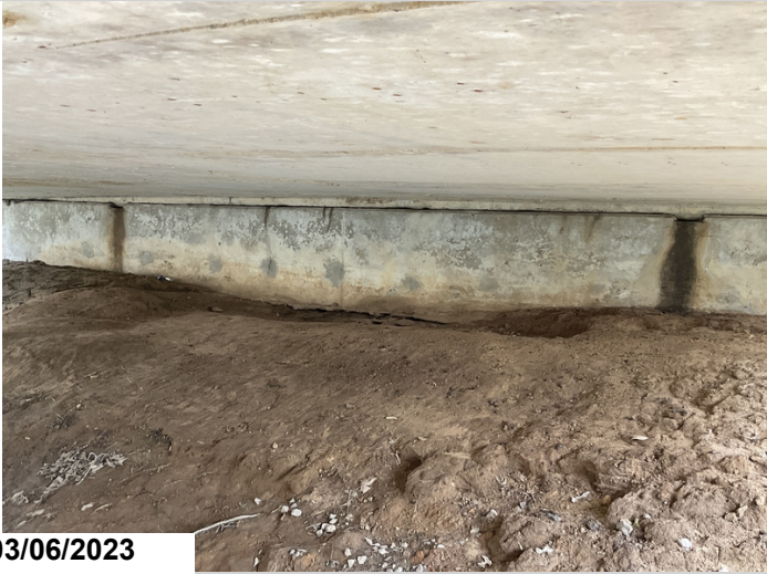
Bent 4 abutment has minor erosion.
