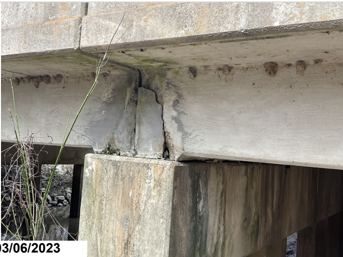
Bent 3 right has cracking delams and spalls.
