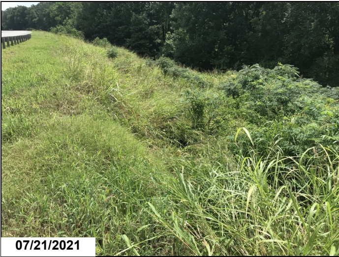
Roadway slope - Bent 9 right: Erosion/slope slumping
