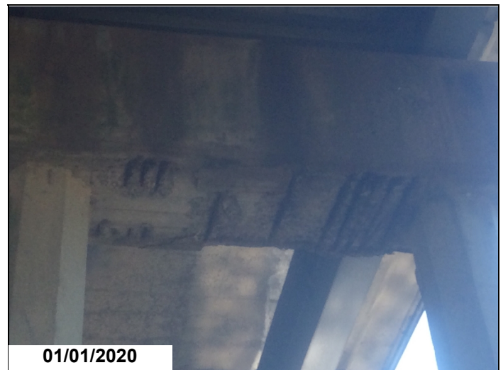
Bent 4 bottom of cap right side has spall with exposed rebar with up to 100% section loss.
