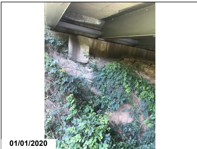
Abutment - Bent 1 right : Erosion
