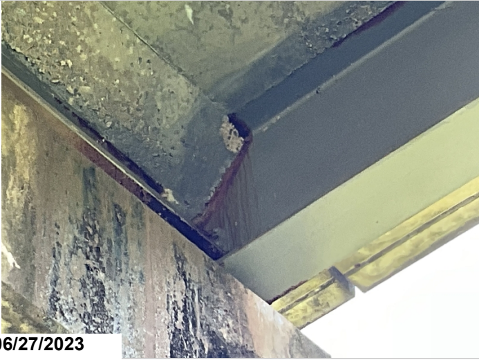
Bent 3 girder 1 rust near haunch area
