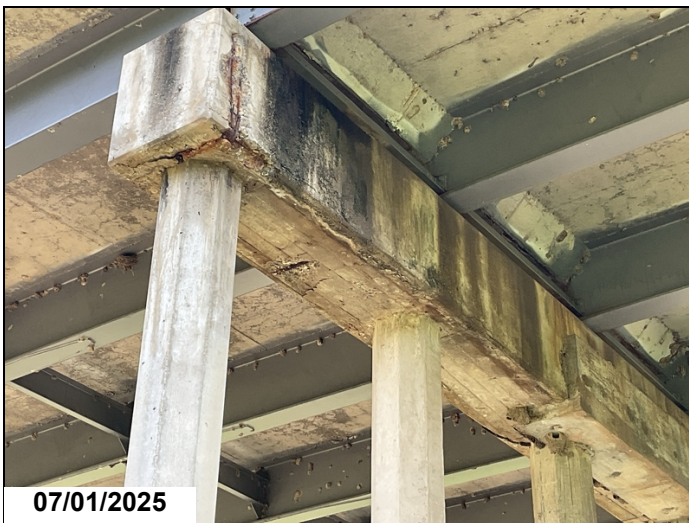
Cap - Bent 6 right: Exposed Rebar
