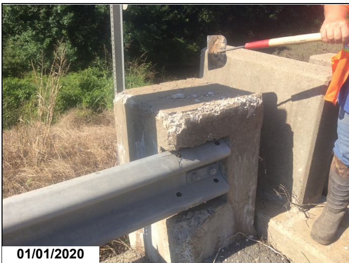
Concrete guard rail end post has efflorescence and has small spalls with delams .
