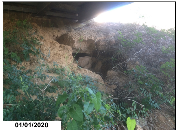
Abutment 1 end slope has moderate to heavy scour exposing bottom of cap.
