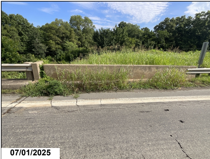
Approach railing transition - Bent 9 left: Cracking/scaling
