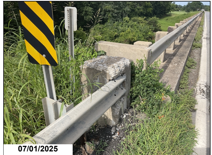
Approach railing transition - Bent 9 right: Scaling
