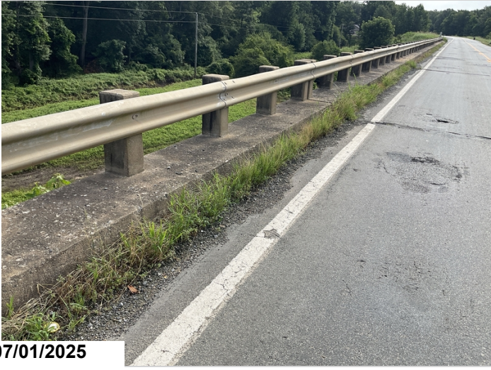
Gutterline - left side: Debris build-up
