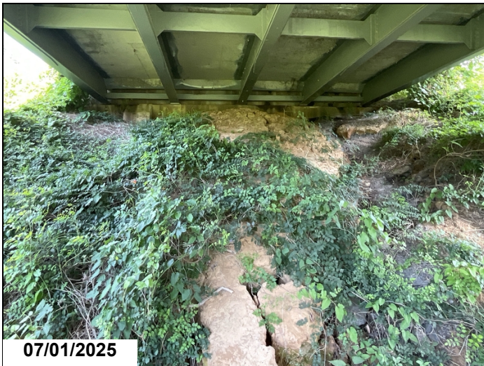
End-slope - Bent 1: Erosion
