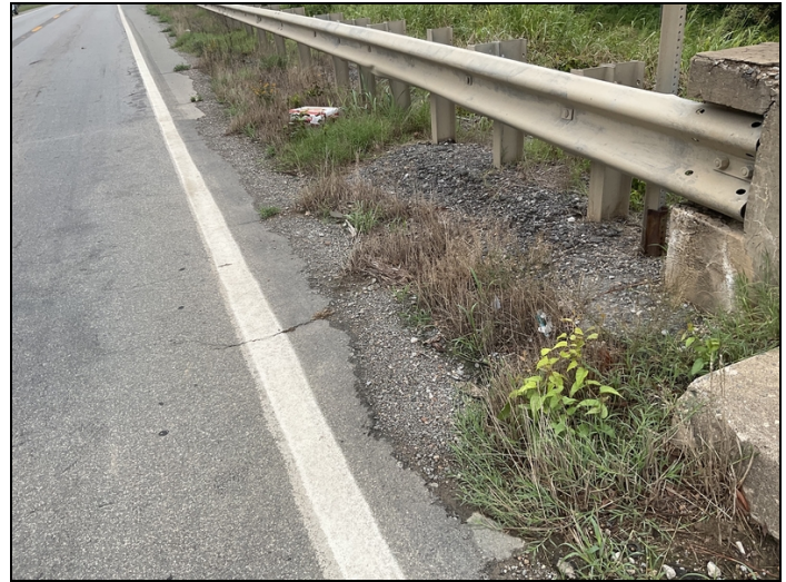
Approach gutter - left side: Debris build-up
