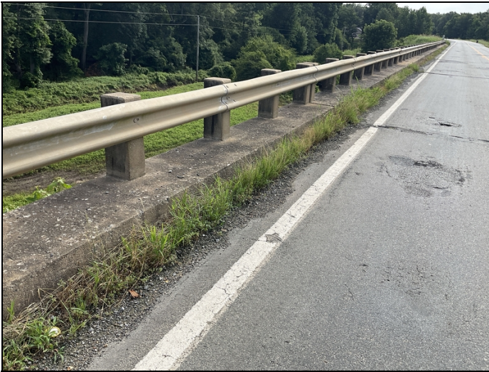
Gutterline - left side: Debris build-up
