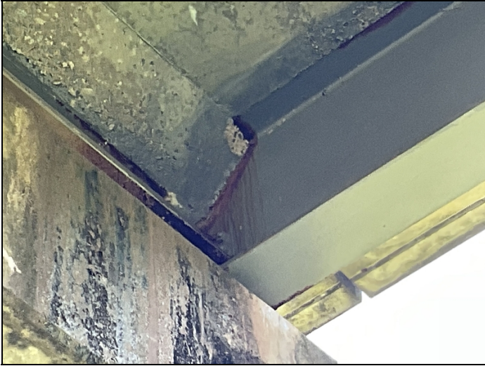
Bent 3 girder 1 rust near haunch area
