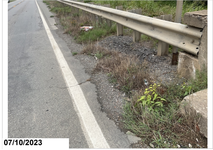
Approach gutter - left side: Debris build-up
