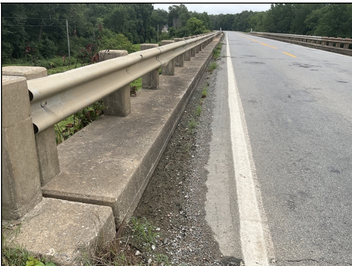
Gutter-line - left side: Filled with debris, restricting storm water runoff
