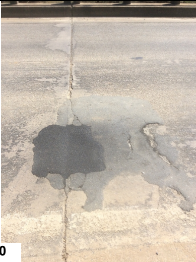
Deck @ Bent 2: Joint damage and patch
