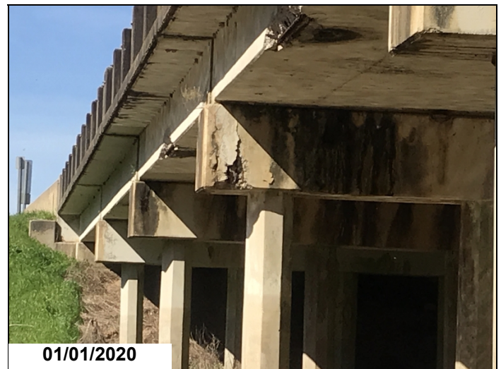
Bent 4 cap ahead right has spall with exposed rebar.
