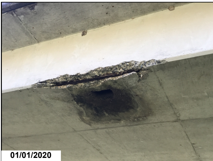
Span 2 left drain opening has spall with exposed rebar.
