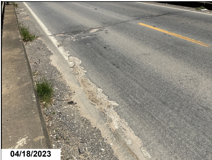
Deck - Span 1 left @ 1/2-3/4 span: Scaling
