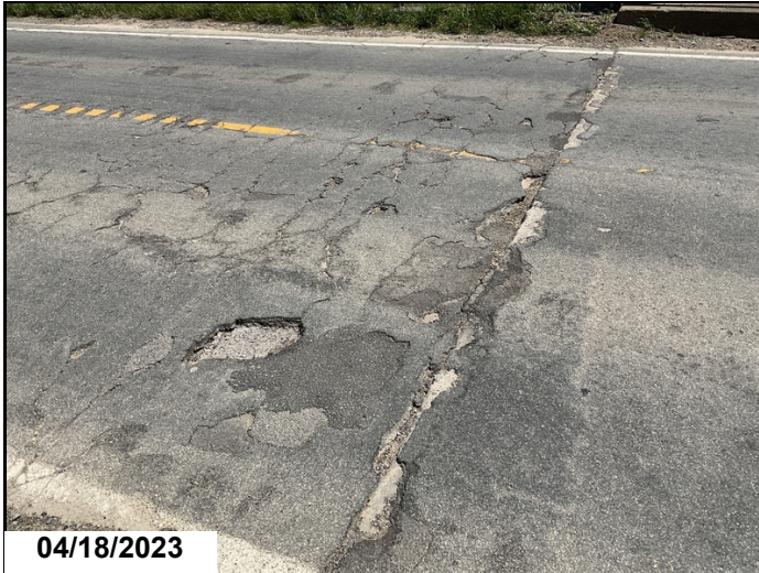
Approach roadway - Bent 8: Deterioration/cracking
