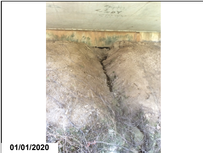
Endslope - Span 1: Minor erosion
