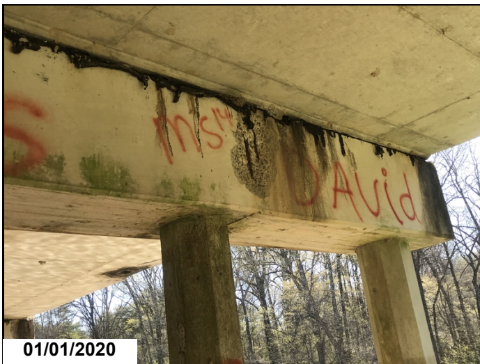
Bent 3 cap back has spall with exposed rebar.
