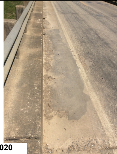
Deck - Span 5 left: Patches
