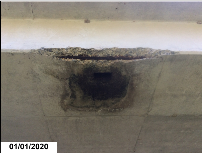
Soffit - Span 2 left: Rebar exposed
