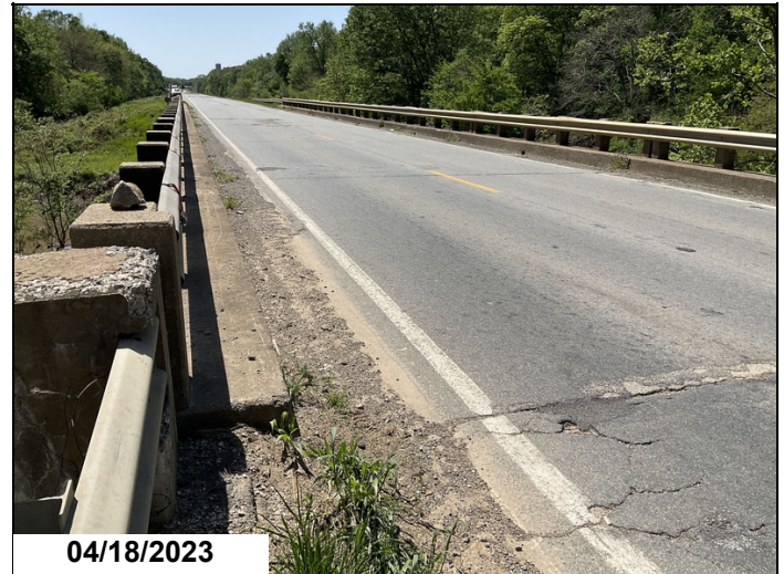
Gutter-line - right side: Debris build-up
