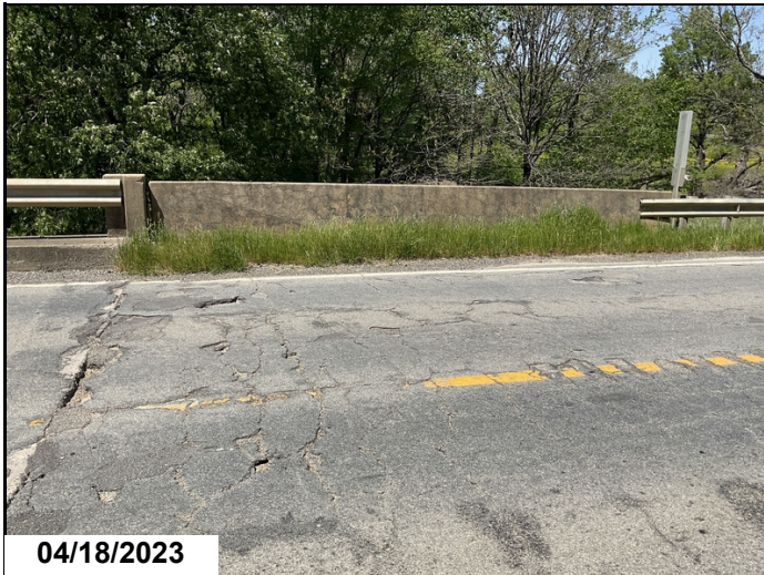
Approach gutter-line - Bent 8 left: Debris build-up
