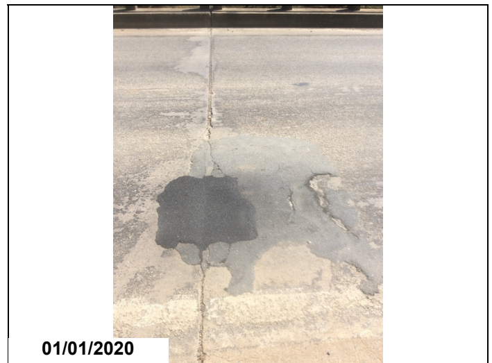
Deck @ Bent 2: Joint damage and patch
