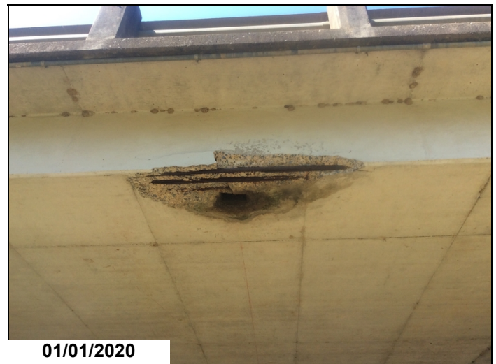
Soffit - Span 6 right: Rebar exposed
