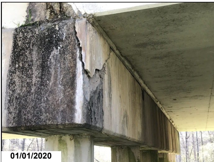
Bent 2 left side of cap has large delam. Common bent 3 left.
