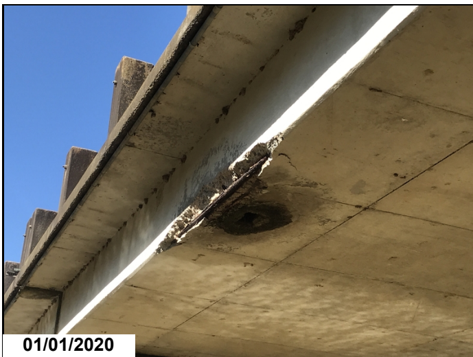
Span 5 right at drain opening has spall with exposed rebar. Common on span s 2,3,4 & 6.
