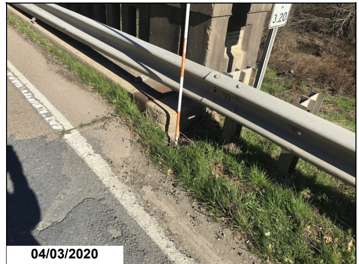
Approach roadway - Bent 1 right : Hole
