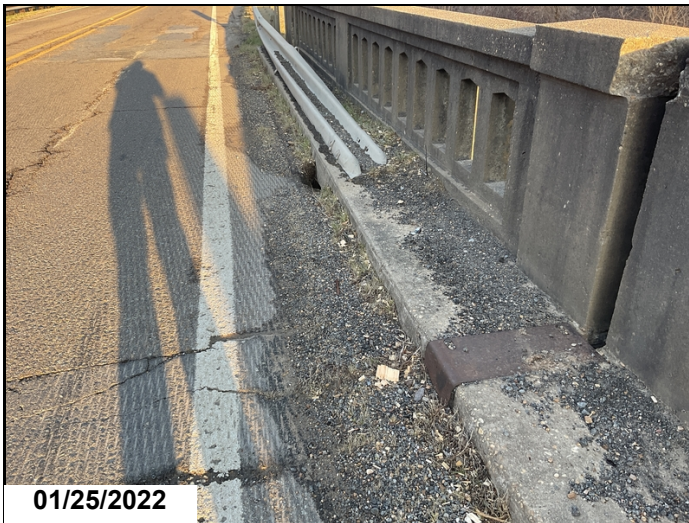
Right gutter line filled with debris.
