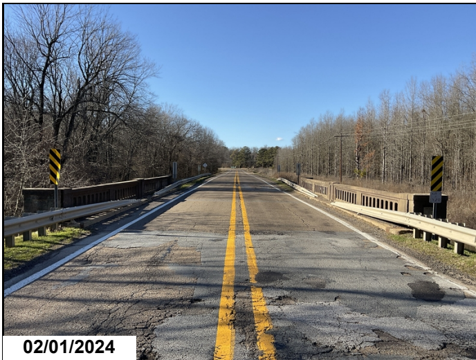
Approach roadway - Bent 1: Deterioration / "hole" - bump - going onto bridge
