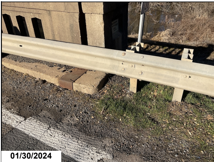
CORRECTED - Approach roadway - Bent 1 right : Hole filled
