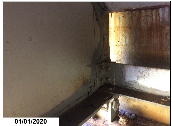
Span 3 Girder 1 right @ Bent 4: Corrosion
