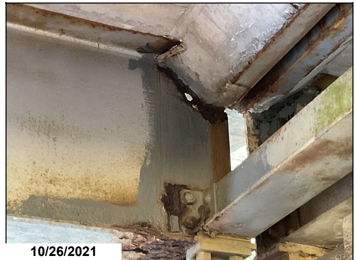
Span 2 Girder 5 @ Bent 2: Corrosion (hole)
