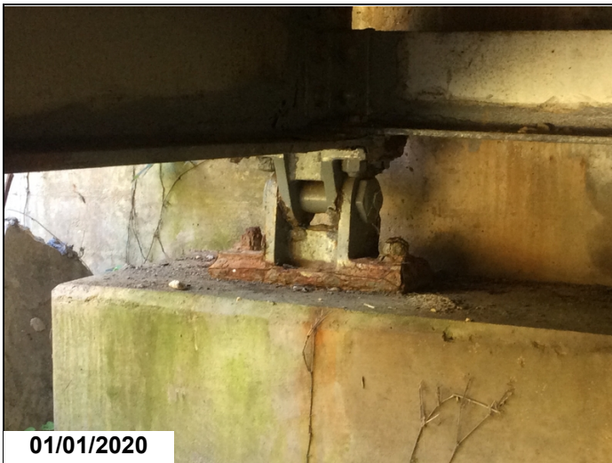
Bent 4 Bearing 1: Corrosion
