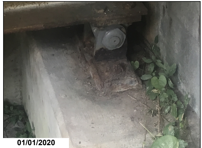
Bent 1 bearing 1 has heavy flaking rust.
