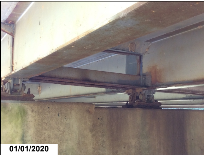
Span 1 Girders 1-2: Corrosion
