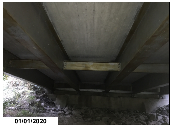
Span 1 under view of paint system.
