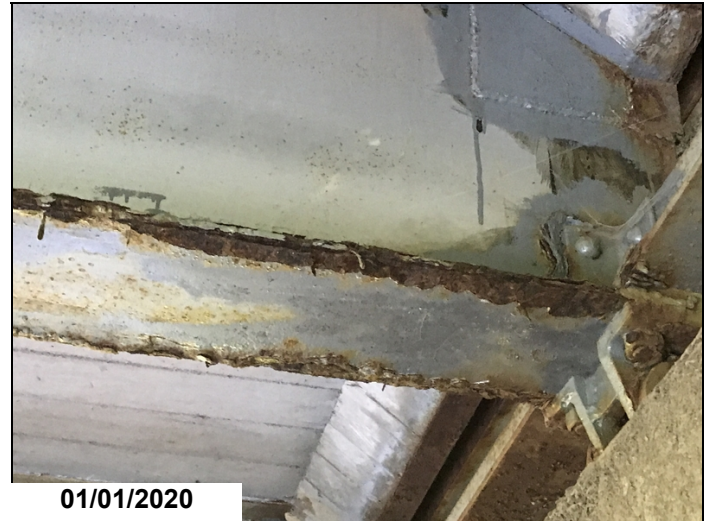
Span 2 at bent 2 girder 3 has heavy flaking rust near bearing area.
