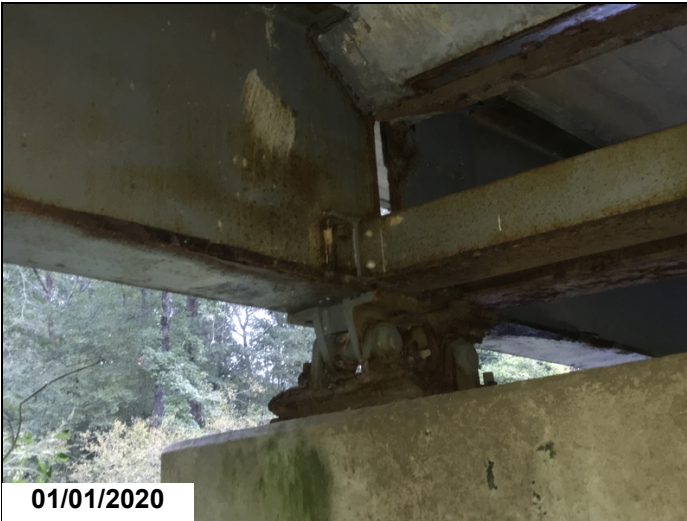
Bent 2 girder 2 beam end has heavy flaking rust.
