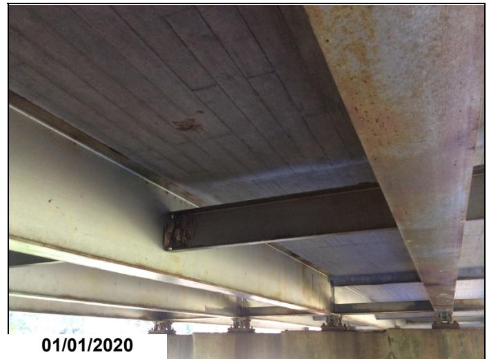
Span 3 Girders 2-3: Corrosion
