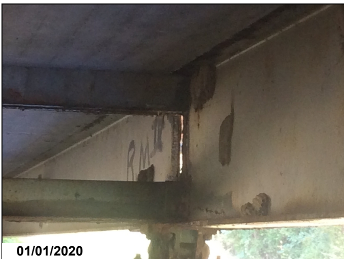
Girders 1 @ Bent 3: Corrosion
