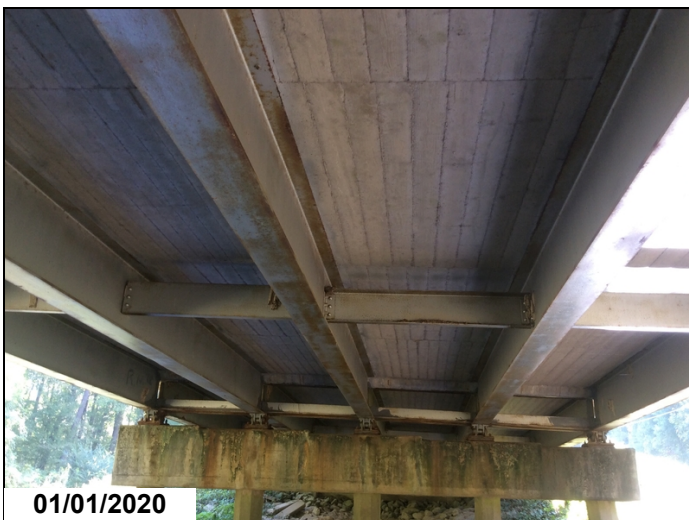
Girders - Span 2: Corrosion
