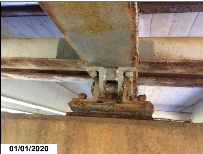
Span 1 Bearing 3 @ Bent 2: Corrosion
