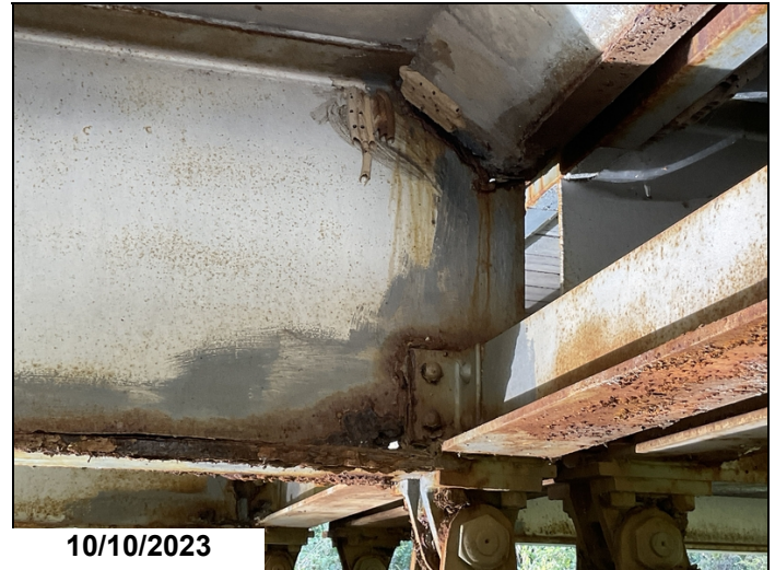
Span 2 Girder 4 @ Bent 2: Corrosion (holes)
