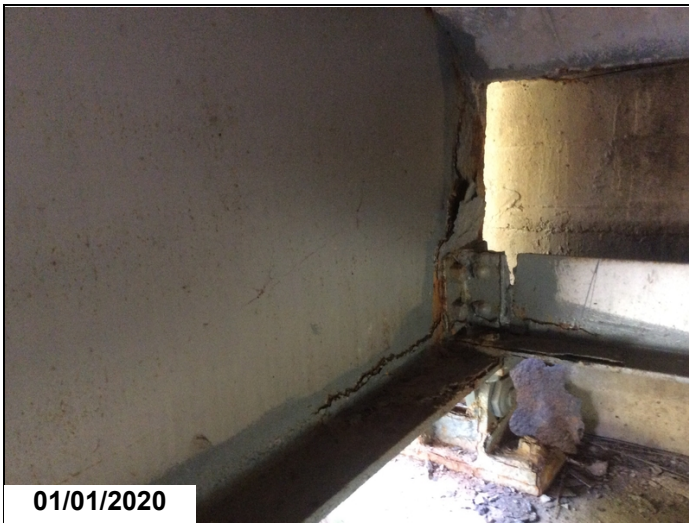
Span 1 Girder 5 left @ Bent 1: Corrosion
