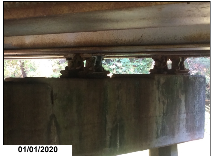
Bearings 1-2 @ Bent 3: Corrosion
