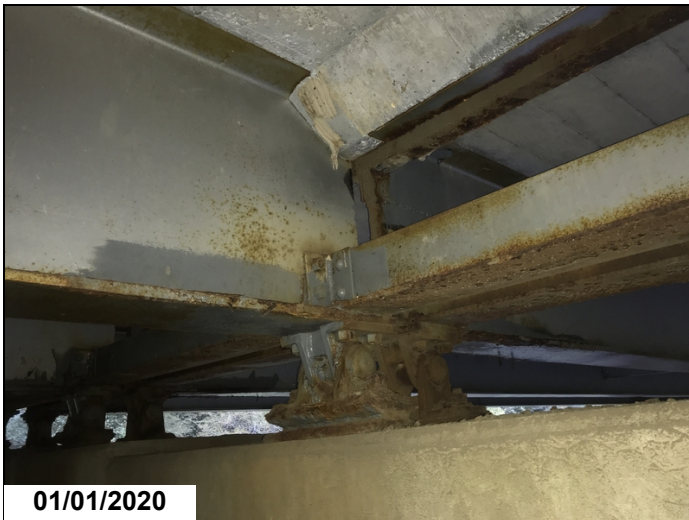
Bent 2 girder 3 beam ends have heavy flaking rust . Common on most beam ends .
