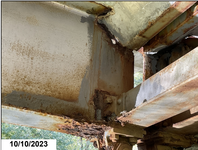
Span 2 Girder 5 @ Bent 2: Corrosion (hole)
