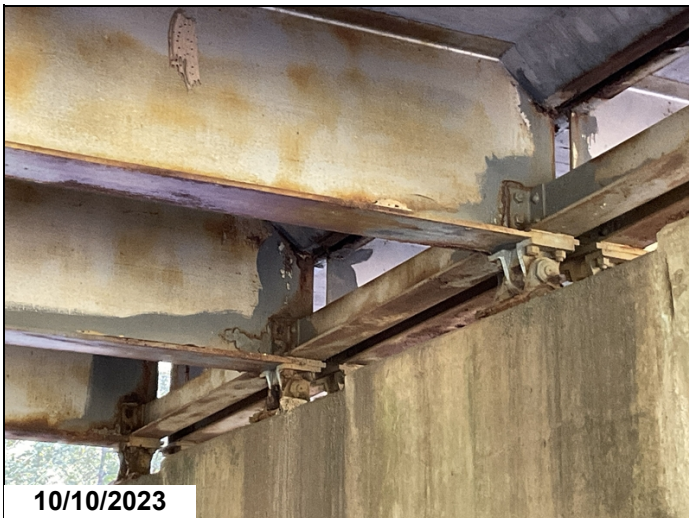
Span 3 Girders 3-5 @ Bent 3: Corrosion
