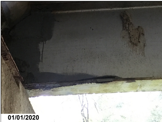
Span 2 at bent 2 girder 1 has flaking rust from end of girder ahead 4'. Common most girders this bridge.
