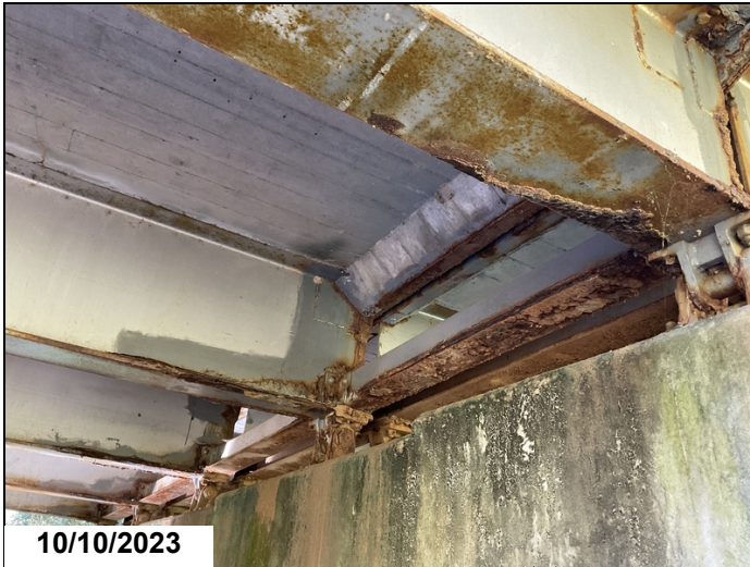
Span 2 Girders 1-3 @ Bent 2: Corrosion
