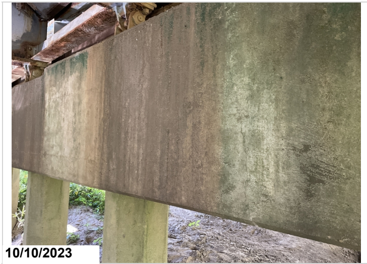
Cap - Bent 2 ahead: Cracking
