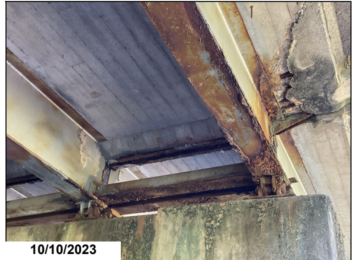
Span 3 Girders 1-2 @ Bent 3: Corrosion
