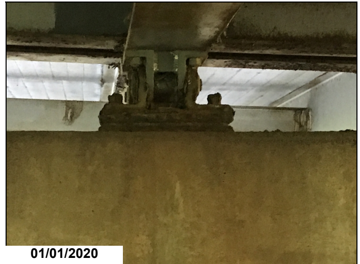
Bent 2 bearing 3 back has heavy flaking rust.
