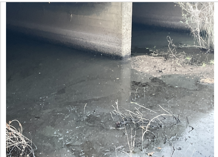
Barrel 3 wall abrasion common on all divider walls.
