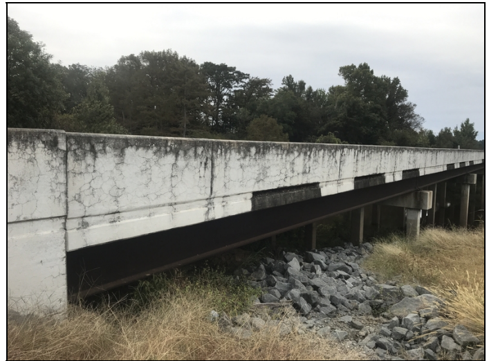
Span 6 map cracking ( common on all concrete bridge railing).
