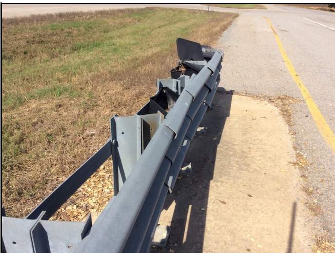
Approach railing - Bent 7 left (damage)
