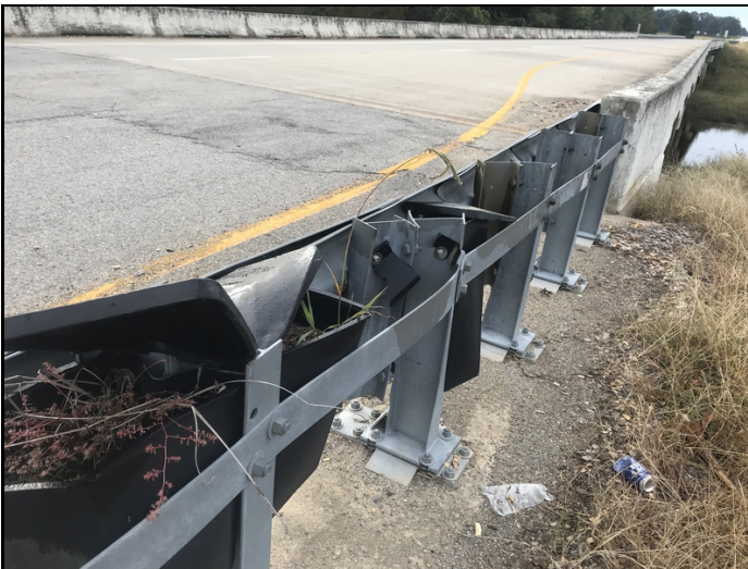
Bent 7 bridge railing and post damage.
