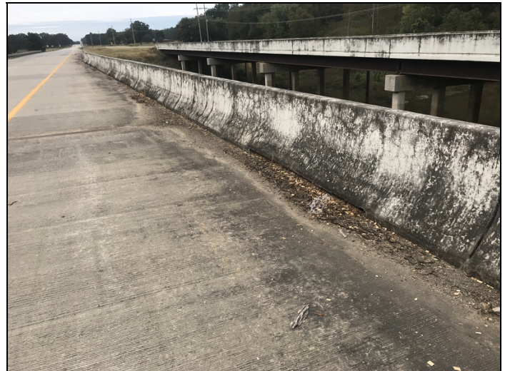
Gutter lines and drains full sediment and debris impeding drainage.
