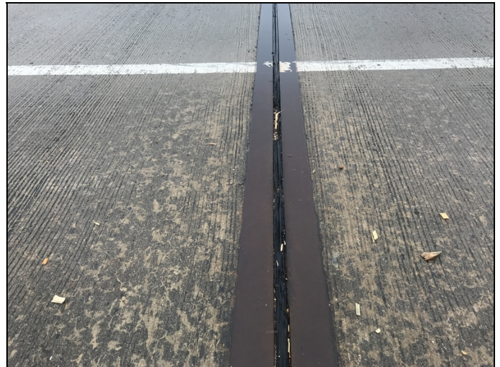
Bent 4 joint seals are torn and leaking.
