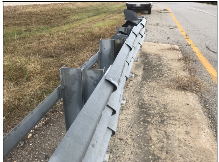
Bent 7 bridge guard rail damage.
