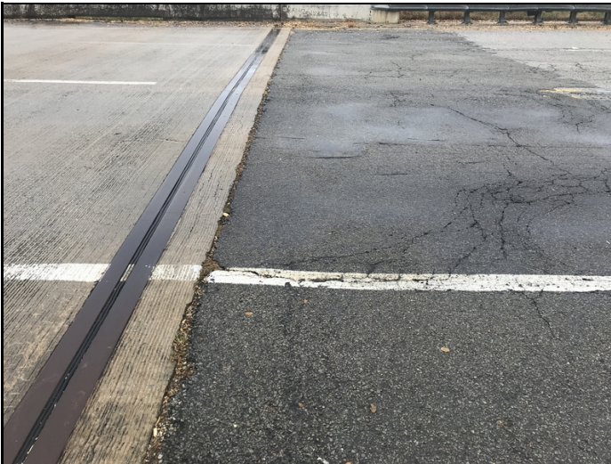
North approach has 1/2" to 1" drop leaving bridge.
