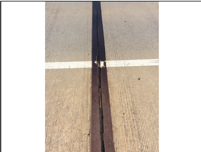
Joint - Bent 4 (damaged)
