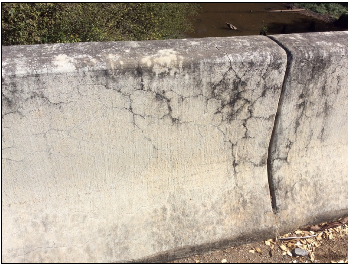
Railing - Span 7 left (typical map cracking)
