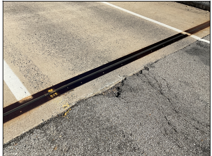
Approach roadway - Bent 1 right: Deterioration/pothole
