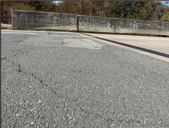
Approach roadway - Bent 1 left: Settlement
