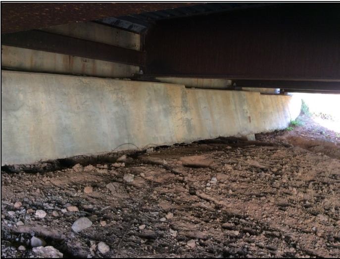
End slope - Bent 1 (settlement/scour)
