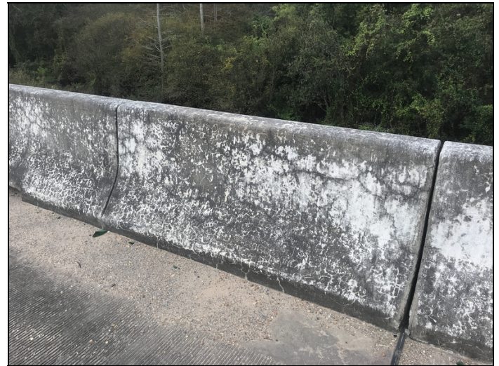
Bridge railing has moderate to heavy map cracking on all spans.
