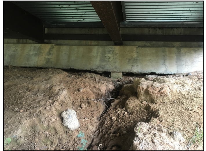
Bent 1 abutment has erosion on left side under cap.
