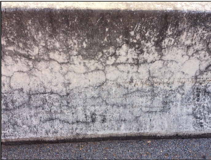
Railing - all spans (map cracking)
