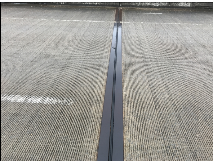
Bent 2 joint seal is torn and leaking.
