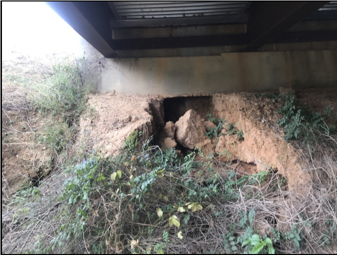
Bent 7 left side has erosion under approaching towards roadway.
