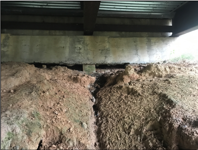
Bent 1 abutment has erosion exposing bottom of cap and pile.
