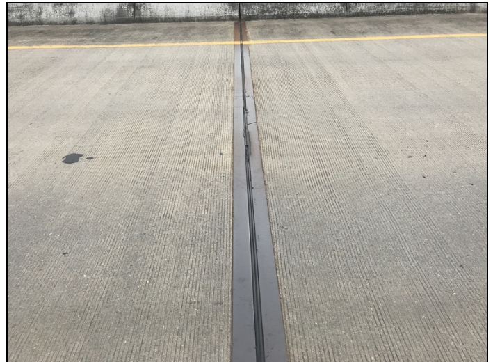
Bent 5 expansion is torn and tattered.
