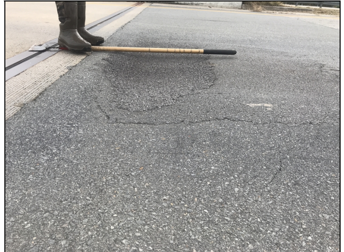
Right lane south bound, approach road way has settlement due to erosion under cap at abutment at bent 1.
