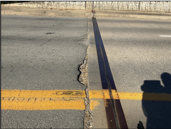
Asphalt approach on South end of bridge at Bent 1 has some potholes in both lanes.
