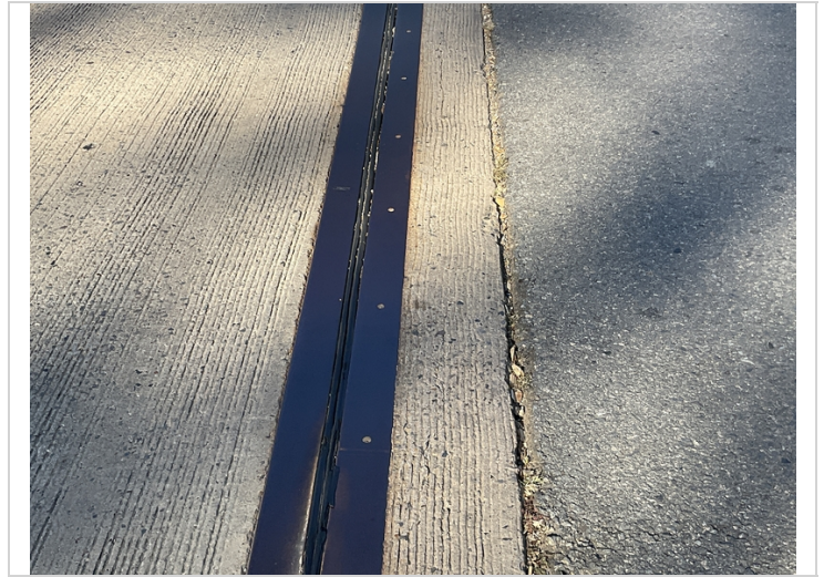
Bent 4 concrete header has cracking right lane northbound.
