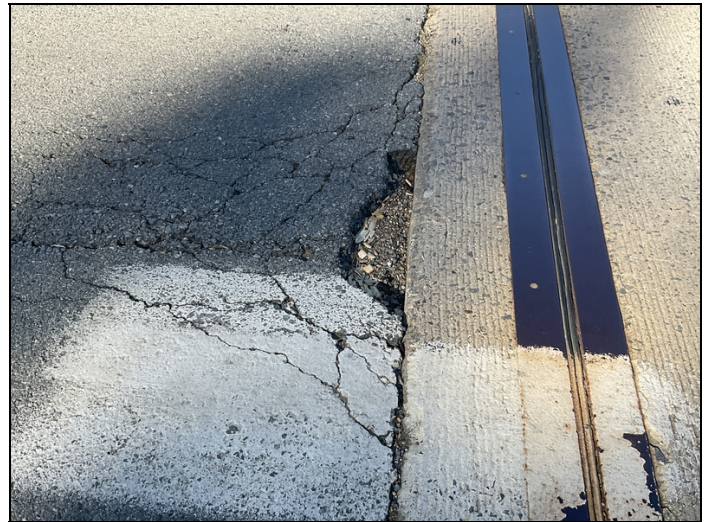
Bent 1 asphalt approach has spalling and a few potholes. (common on bent 4 right lane headed south .)
