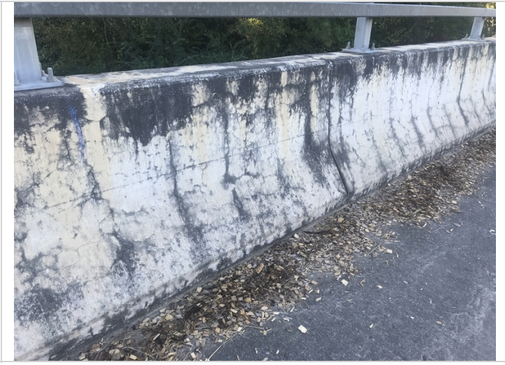
Bridge rail right side has map cracking. Common left.
