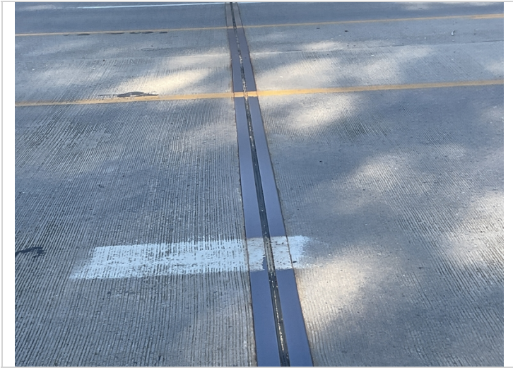
Bent 3 joint seal has some loss of adhesion.
