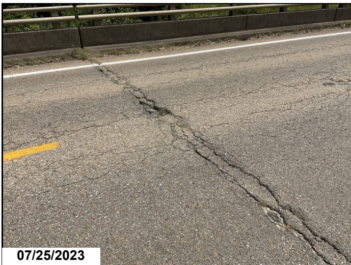
Wearing surface - Bent 3: Spalling (pothole)
