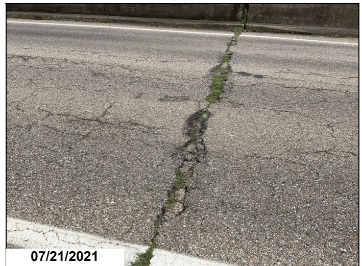
Approach asphalt as spalling.
