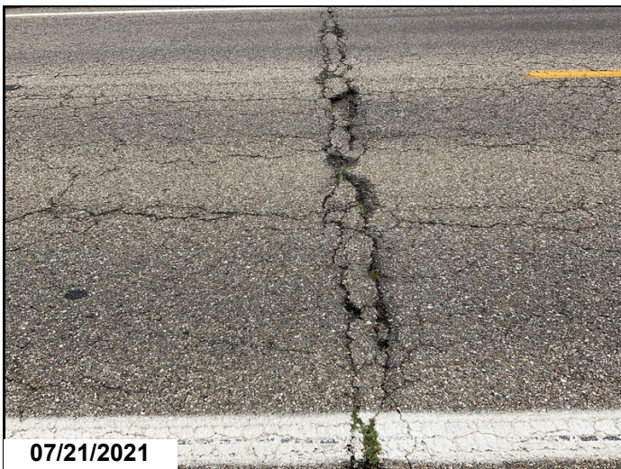
Bent 3 spalling to asphalt wearing surface.
