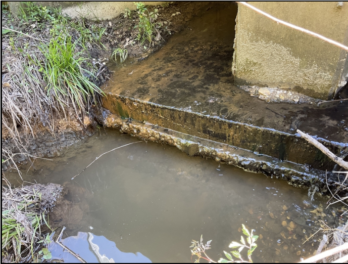
Channel - Barrels 3-4 left: Erosion
