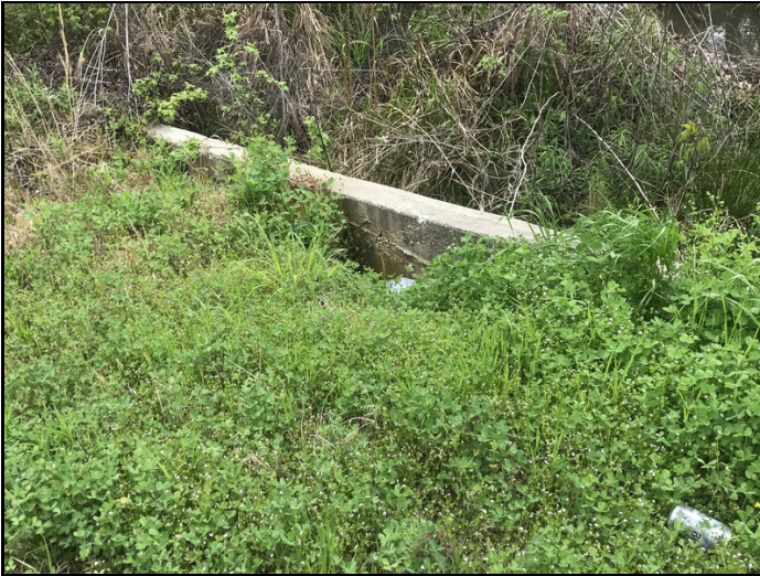
Northeast wing wall has some erosion exposing back face of wing.
