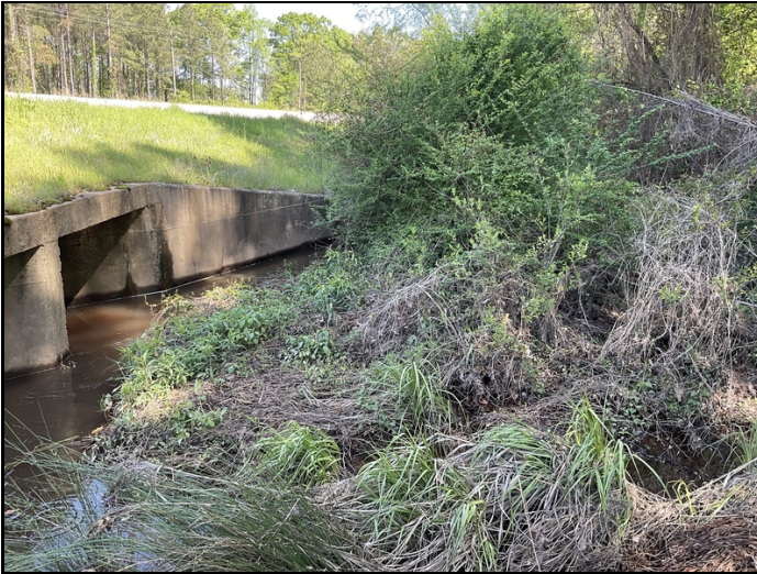
Trees, vines and vegetation on right side (inlet end) of culvert.
