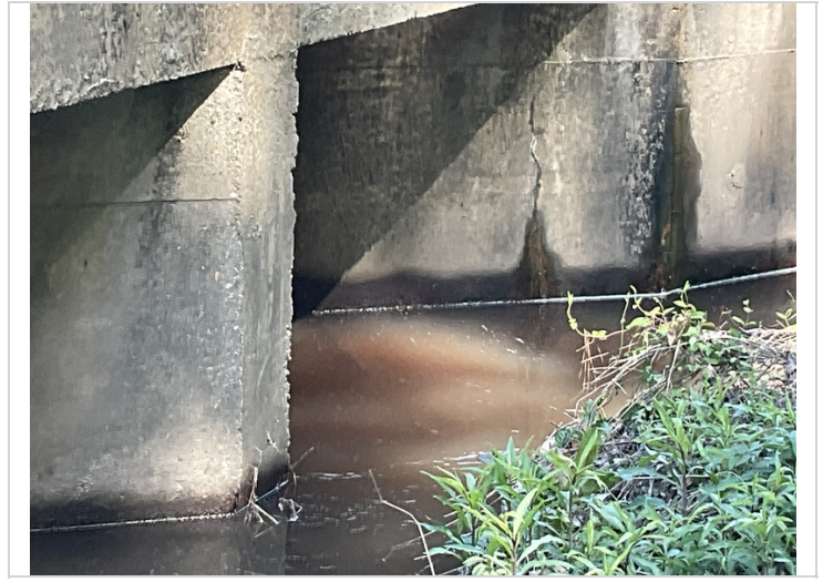
Barrel 3 right has cracking on wall and near wing wall..
