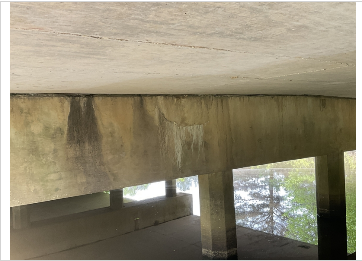
Bent 3 cap right ahead has delam at key way.
