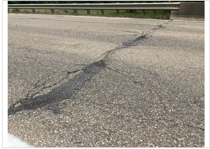
Heavy settlement and rutting on approaches.
