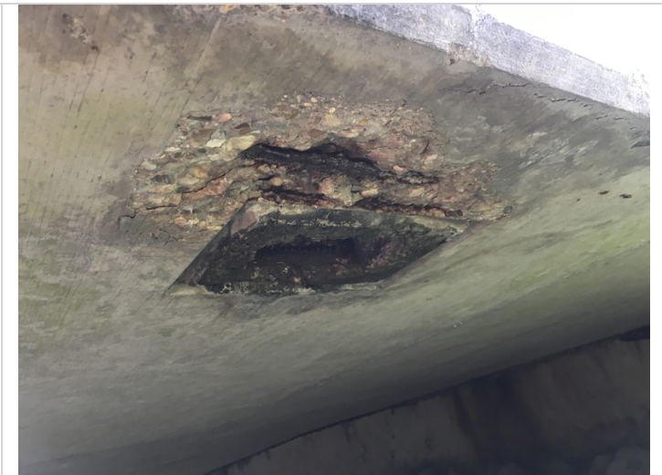
Span 1 left has small spall at drain opening.
