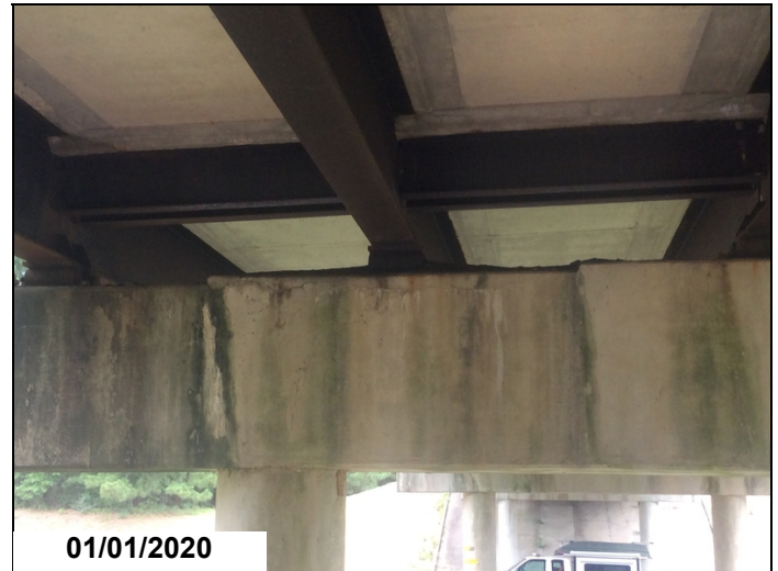
Cap - Bent 4: Delamination
