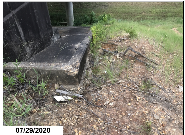
Bent 1 right enslope has erosion.
