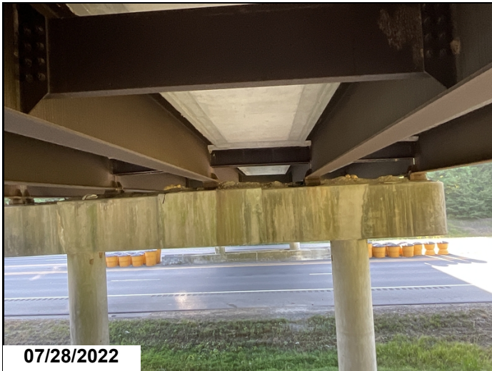
Bent 4 cap has debris on cap.
