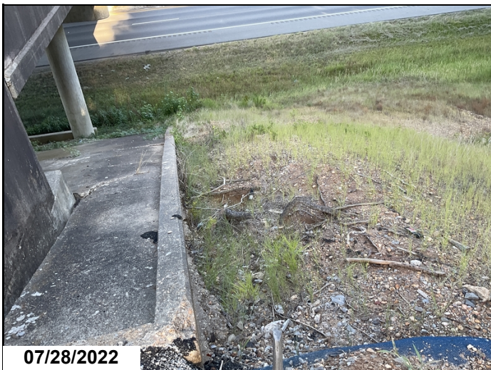
Bent 1 right has erosion at end slopes.
