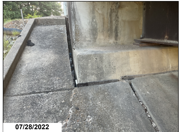
Bent 1 right slope paving separation due to erosion.
