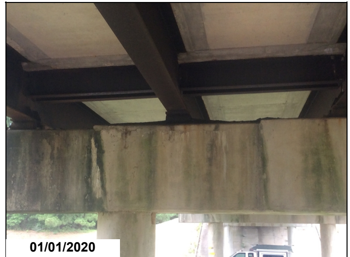
Cap - Bent 4: Delamination
