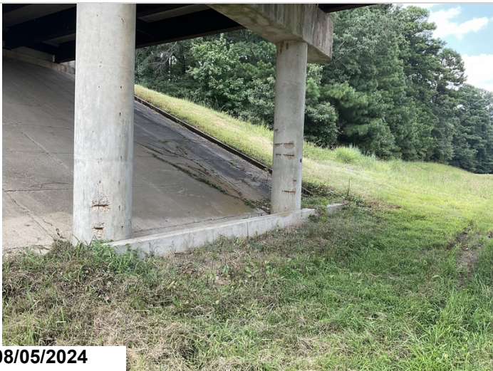
Bent 4, columns 1 & 3 - CS3 Exposed Rebar
