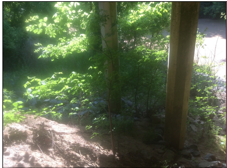
Span 1 & 2 small trees growing under bridge.
