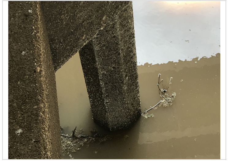
Bent 4 Pile 7: Abrasive wear
