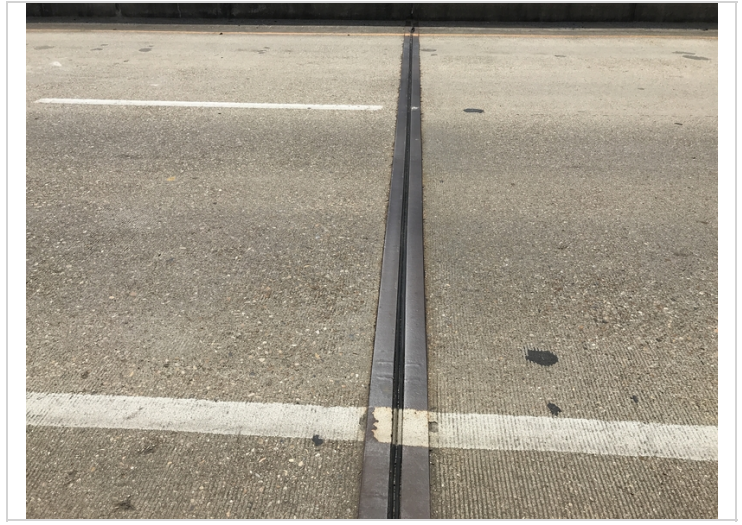
Joint - Bent 2 left: Adjacent deck spalling
