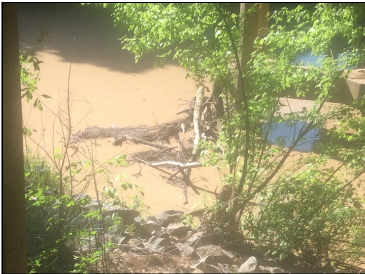
Bent 3 drift and debris against pile on upstream side.
