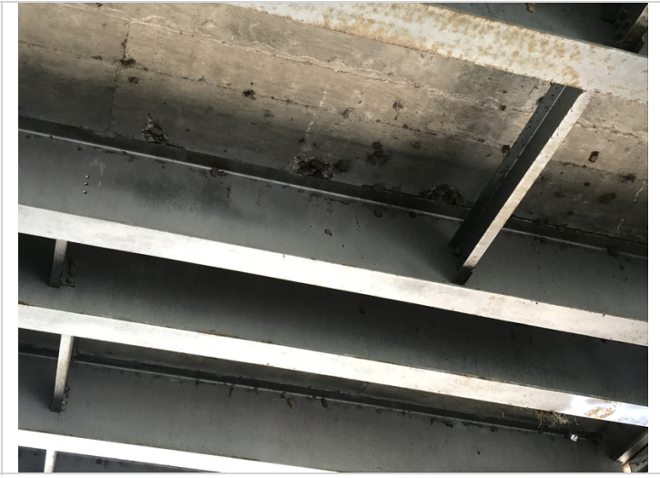
Soffit - Span 4 Bay 5: Rebar exposed
