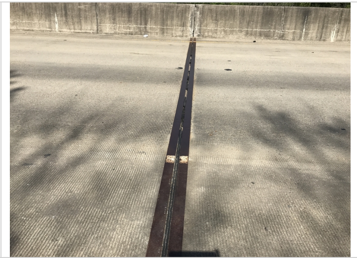
Joint - Bent 2 right: Damage
