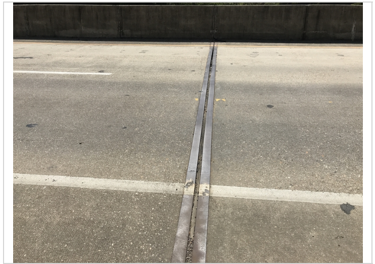
Joint - Bent 5 left: Loss of adhesion
