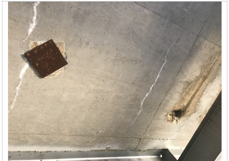
Soffit north bound lanes has spalls from screed placement. As built.
