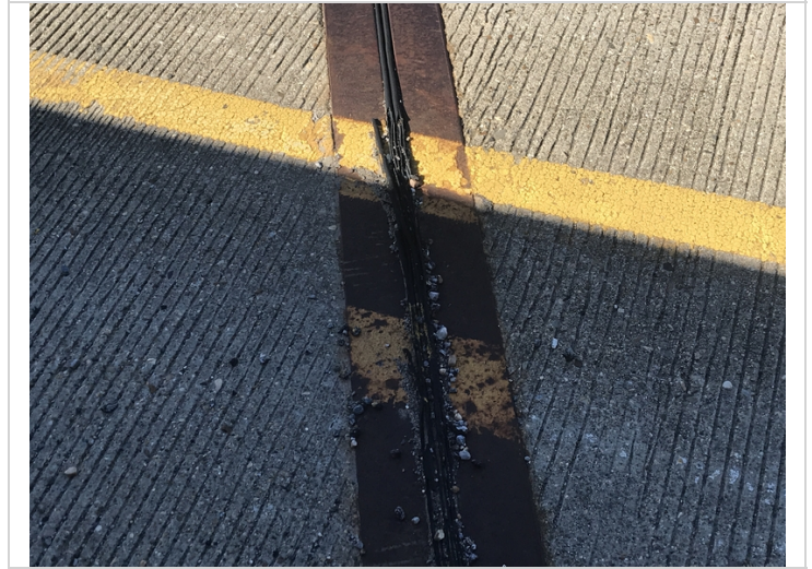
Bent 2 joint seals are torn and leaking near gutter line south bound.
