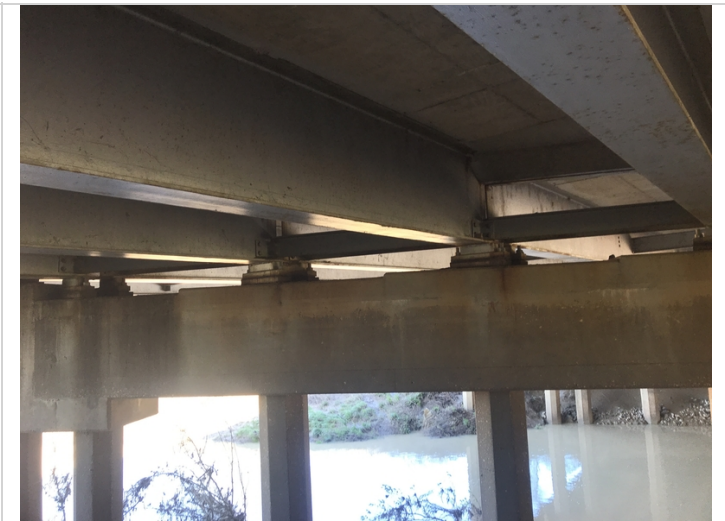
Bent 3 bearing has rust with flaking.
