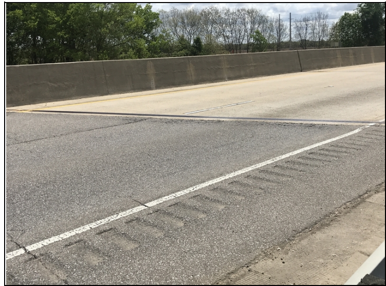
Approach roadway - Bent 1 SB: Settlement
