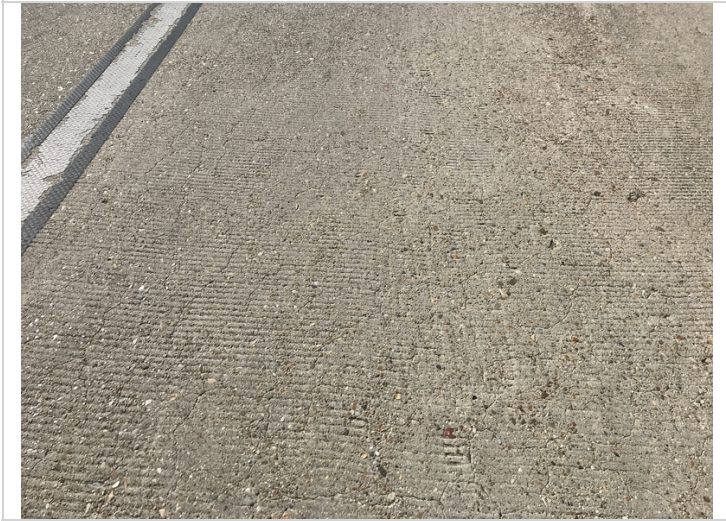
North bound span 2 map cracking in deck.
