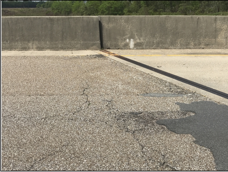
Approach roadway - Bent 4 left inside : Settlement
