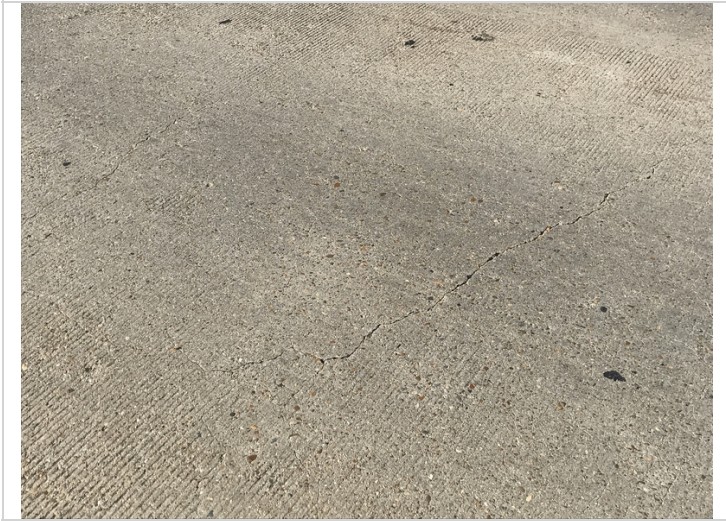
Unsealed transverse cracks.
