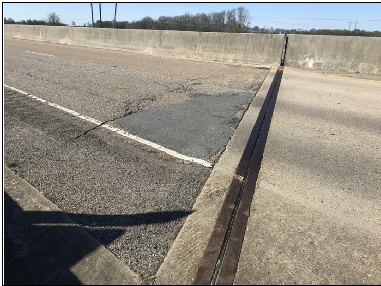
North bound approach roadway has cracking and settlement at bridge end.
