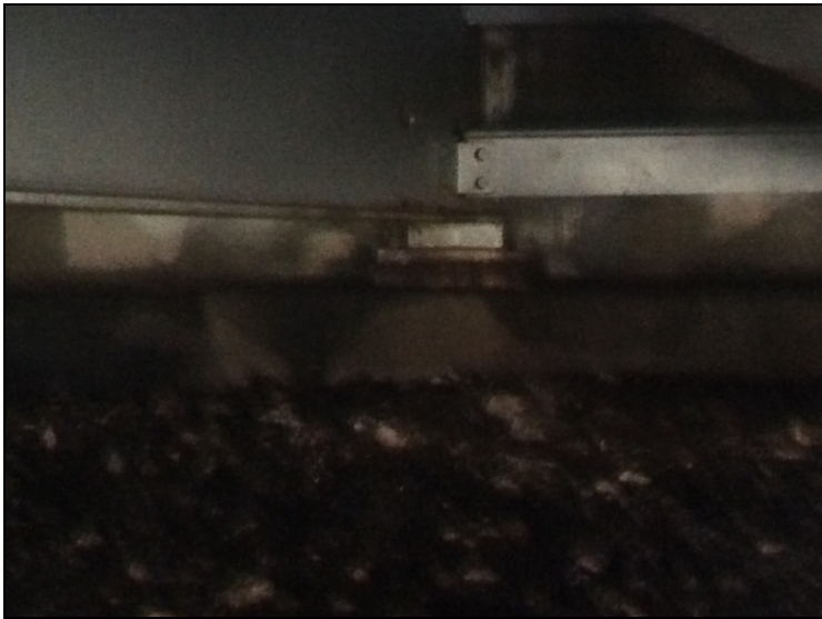
Bent 1 bearing 10 has moderate rust forming
