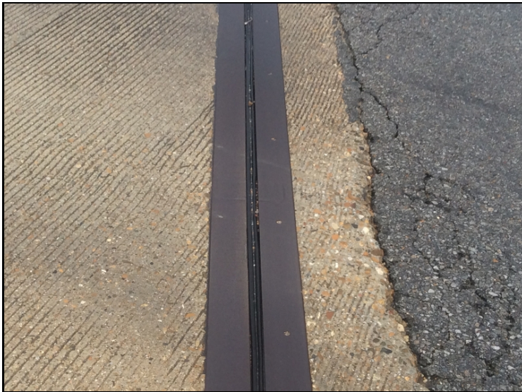
Bent 1 as logged heading south expansion joint is leaking lose of adhesion
