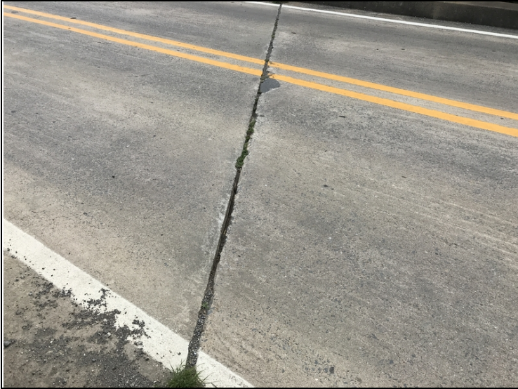
Joint - Bent 2: Material missing/debris filled
