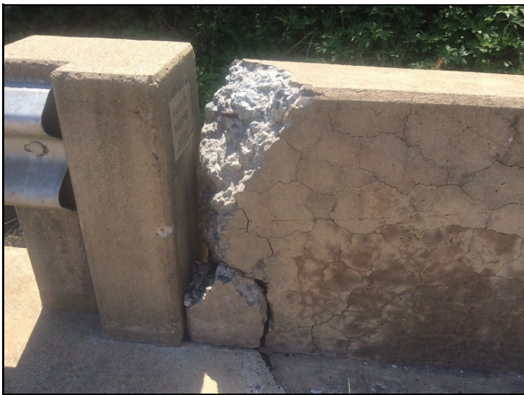
Southeast corner of bridge , guard rail end post has spalls with chloride contamination.
