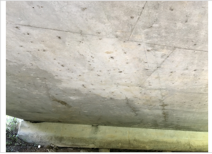
Soffit - Span 3: Cracking/rust-staining
