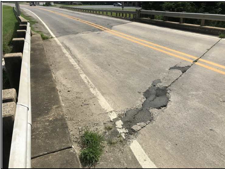
Deck @ Bents 3-4: Spalling/patches
