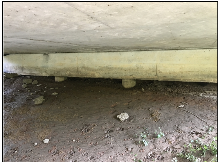
End-slope - Bent 4: Settlement/piling exposed
