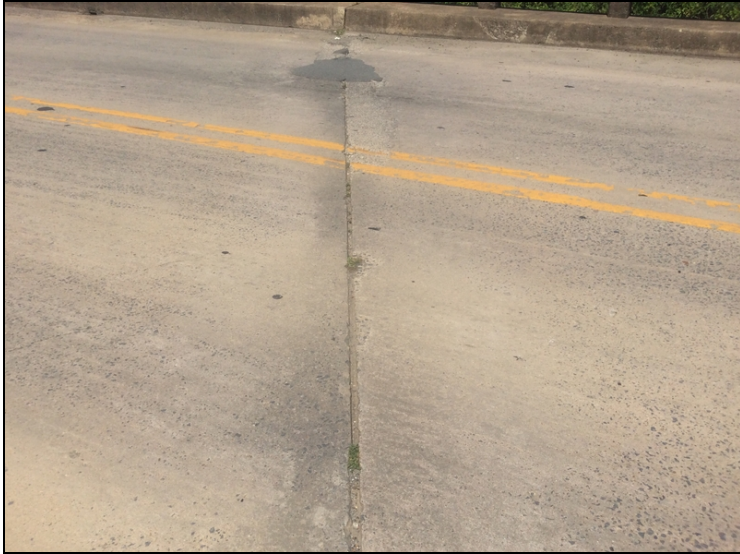
Bent 3 joint seal filled with dirt and debris. Common all bents.
