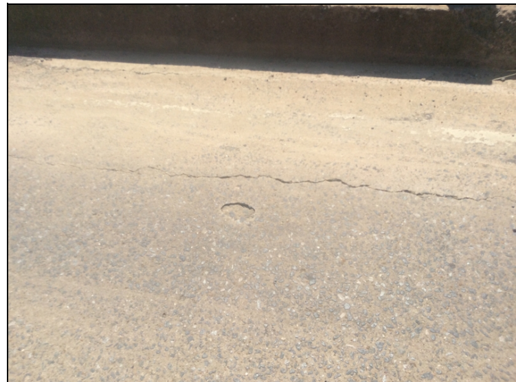
Span 1 near bent 1 right side has large unsealed longitudinal crack.
