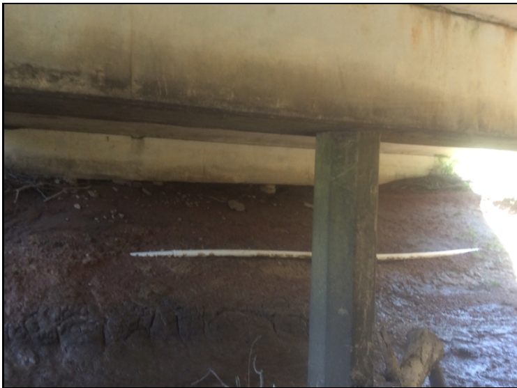
End Slope erosion area under bottom of cap on bent 4 .
