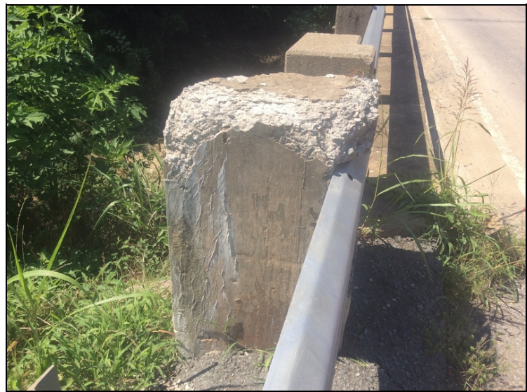
Southeast corner of bridge, guard rail end post has spalling with heavy chloride contamination..
