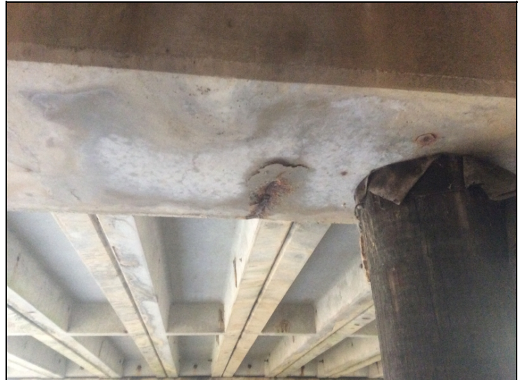
Bent 2 cap near pile 3 has spall with exposed rebar .
