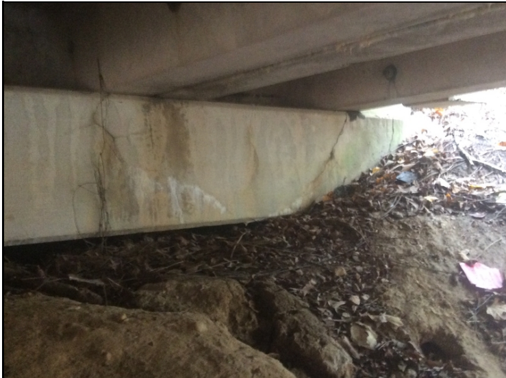
Bent 4 abutment right has cracking with efflorescence and delambs
