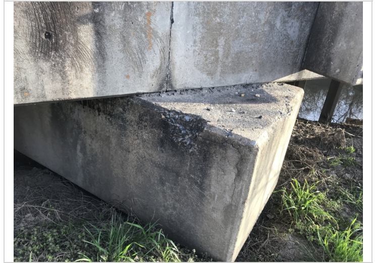
Bent 2 cap right has spall and delam.
