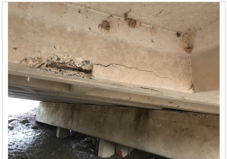
Span6 unit 7 has spall with exposed rebar.
