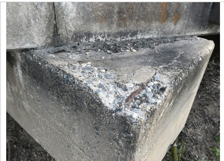
Cap at bent 6 has spall with exposed rebar.
