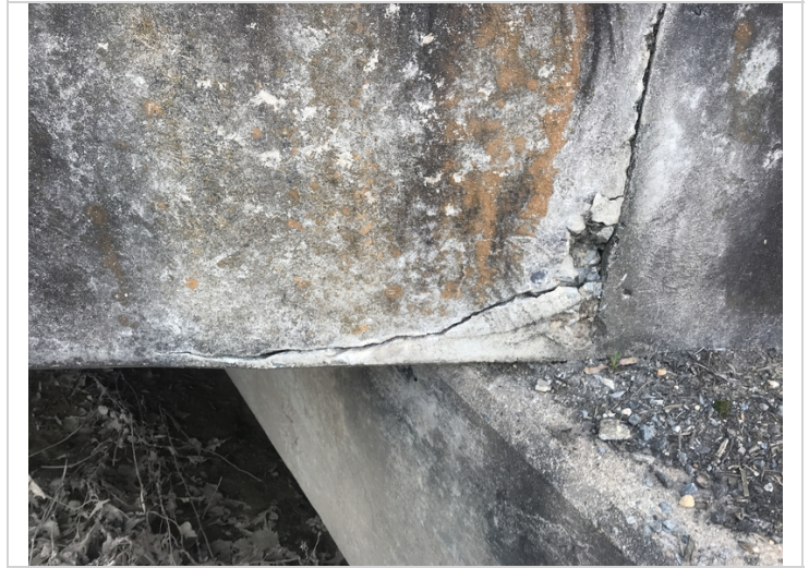
Span 6 near bent 7 girder 7 has cracking and delams.
