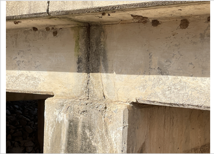
Deck - side of slab - Span 3 right @ Bent 3: Cracking
