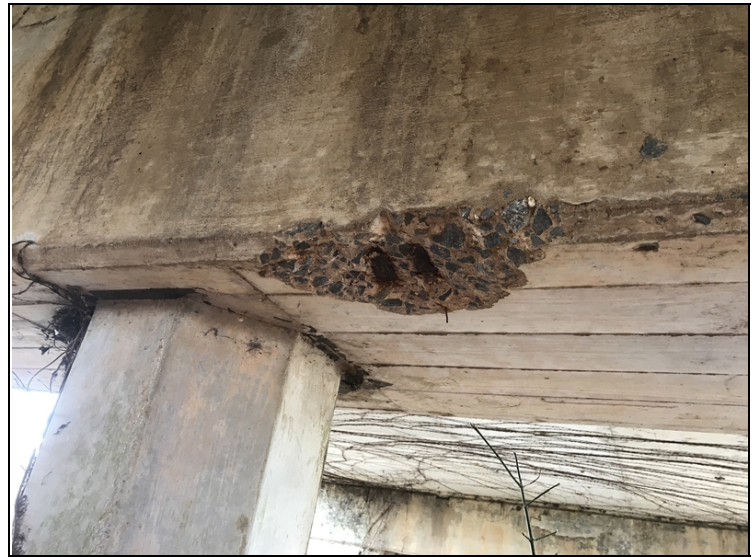
Spall with exposed rebar at bent 2 under cap near pile 2.
