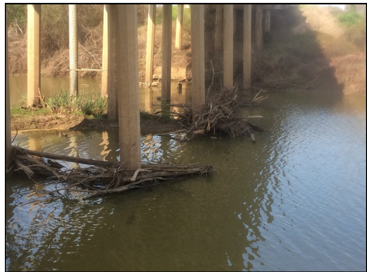
Channel - Bents 5-7: Debris build-up
