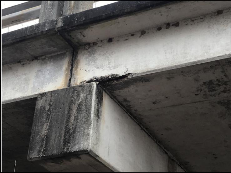
Span 9 at Bent 10 left behind under side of deck near cap has delam and spall with exposed rebar.
