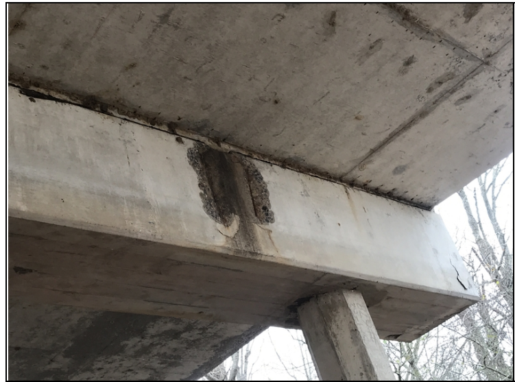
Bent 10 cap right has spall with exposed rebar.
