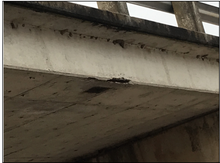
Span 7 left has spall with exposed rebar near drain opening on under side of deck.
