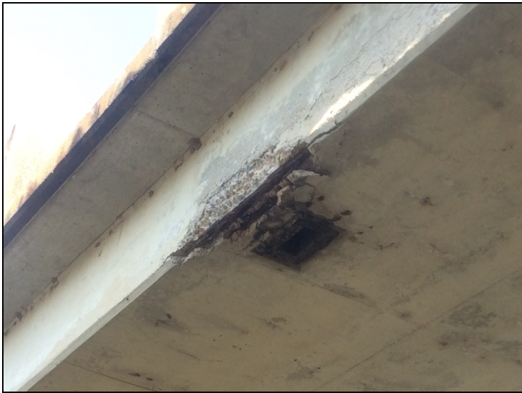
Soffit - Span 8 right: Rebar exposed
