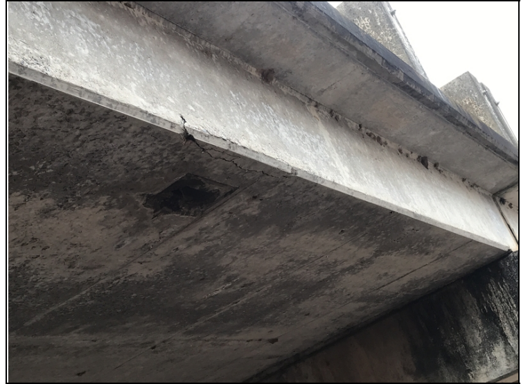
Span 10 under side of deck at soffit area at drain opening has cracking with delams.
