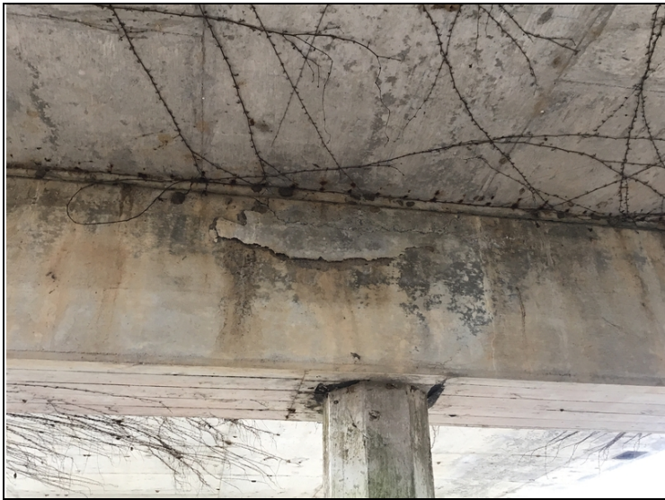
Bent 3 cap back has delams.
