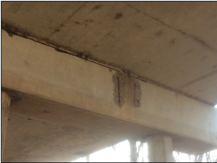
Caps - Bent 10 back: Rebar exposed
