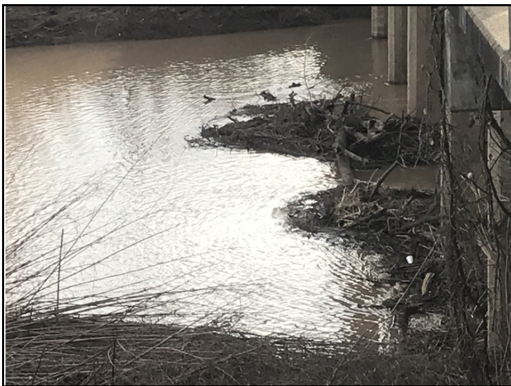
Drift and debris at bent 4-6 impeding waters flow.
