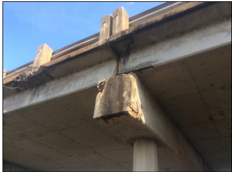
Cap - Bent 9 right end: Rebar exposed
