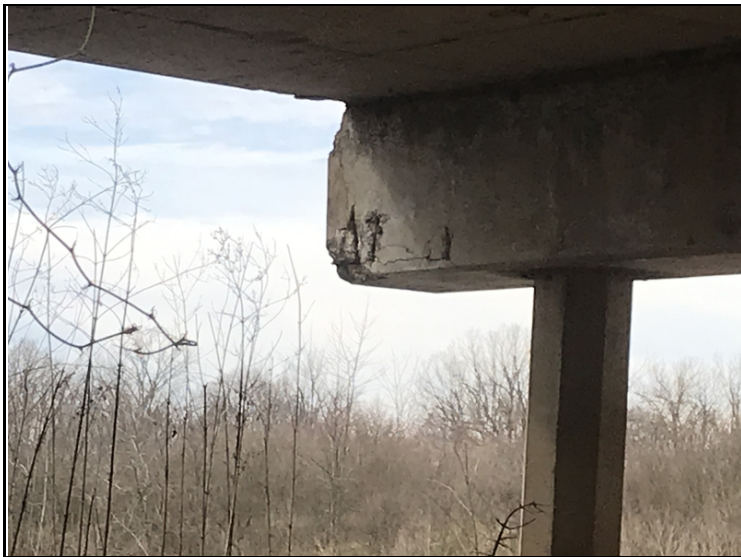
Bent 9 cap right ahead has spalls with exposed rebar.
