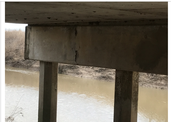
Bent 2 cap left behind cracking with delams.
