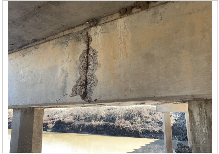
Bent 2 back has spall with exposed rebar and cracking.
