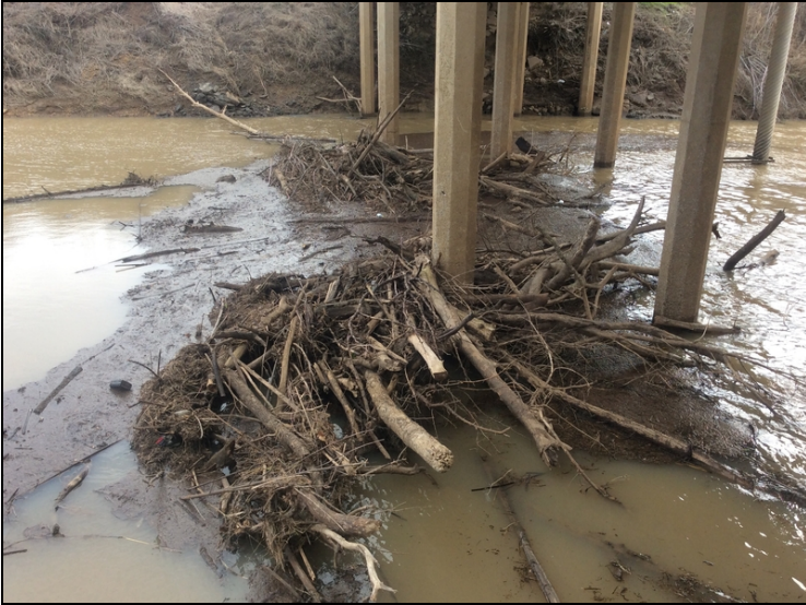
Channel - Bents 3-4 left (debris build-up)
