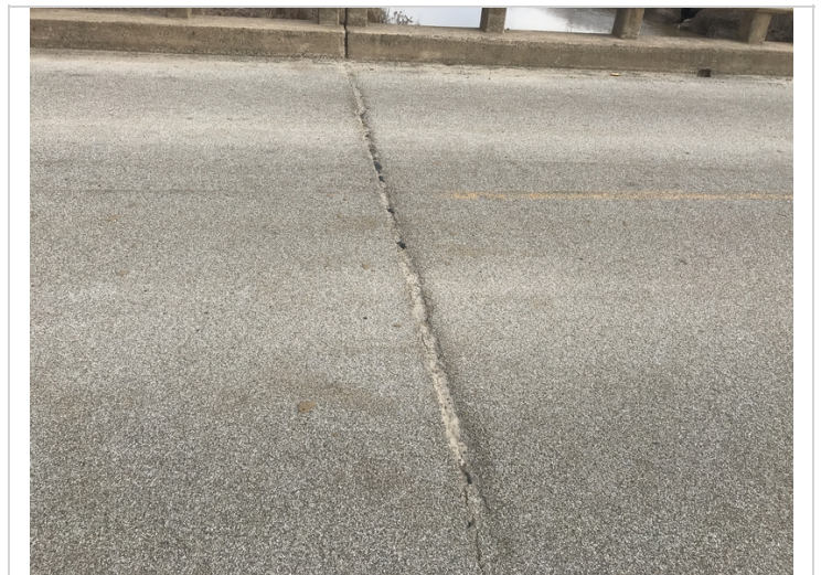
Bent 2 joint seal has debris impactation due to epoxy overlay.
