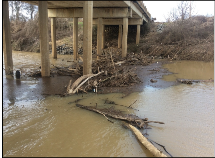
Channel - Bents 3-4 left (debris build-up)
