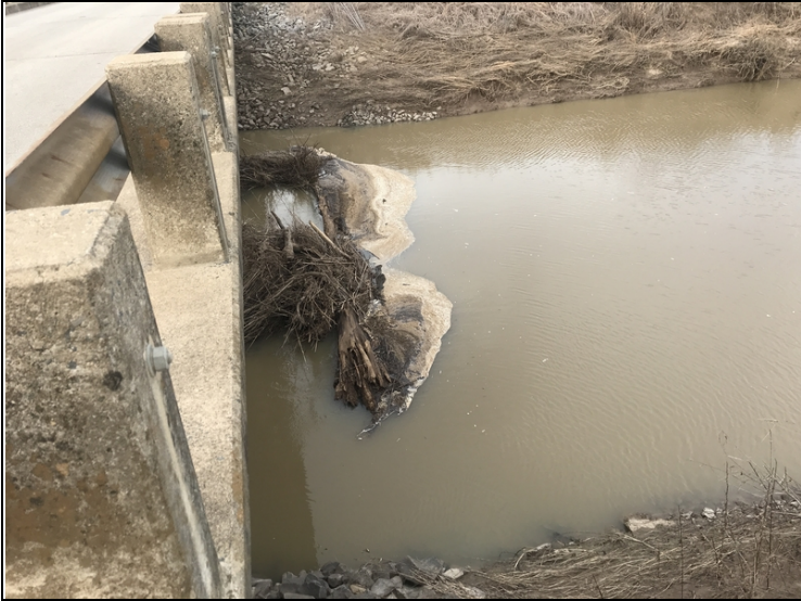
Drift and debris restricting water flow at bents 3&4.
