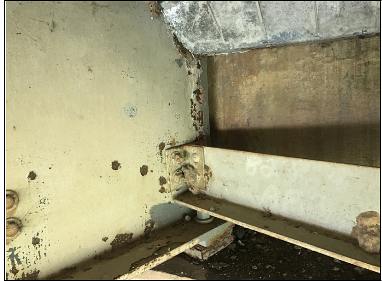
Span 1 Girder 2 left @ Bent 1: Corrosion
