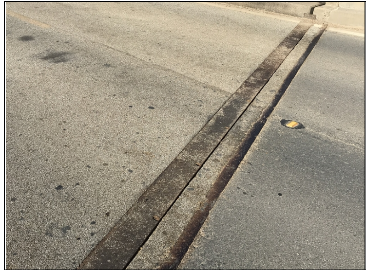
Joint - Bent 5: Sliding plate loose
