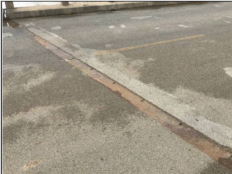
CORRECTED - Joint - Bent 4: Deck repaired/polymer sealed
