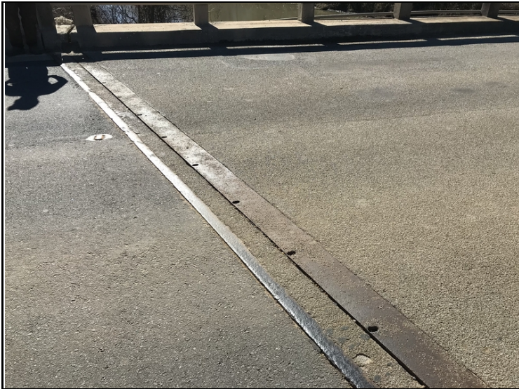
Joint - Bent 5: Sliding plate loose
