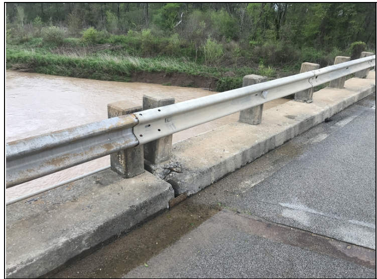
Railing - Bent 4 right: Post damaged
