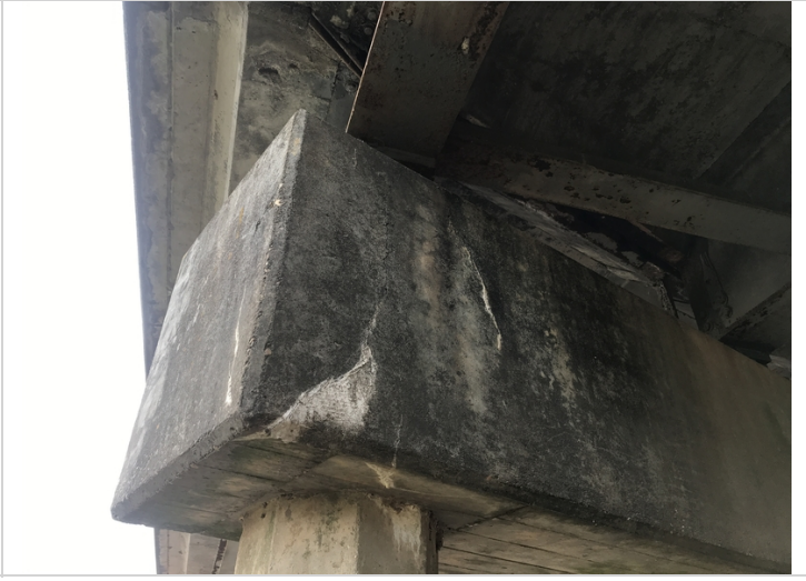
Cap - Bent 2 back left: Cracking with efflorescence
