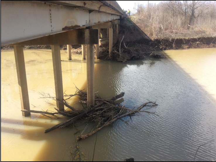
Channel - Bents 3-4 left (debris build-up)
