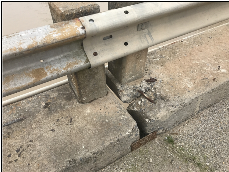
Span 3 near bent 4 has some rail post damage right side.
