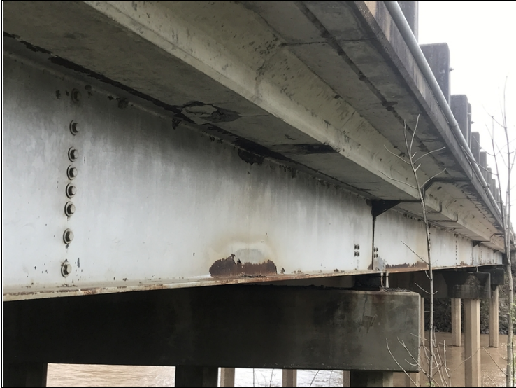
Spans 1-2 Girder 5 right: Corrosion
