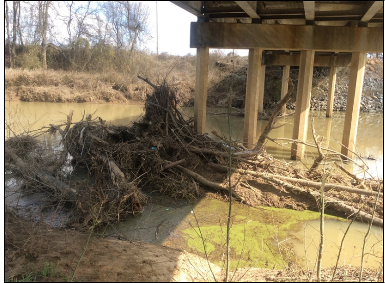
Channel - Bents 3-4 left (debris build-up)
