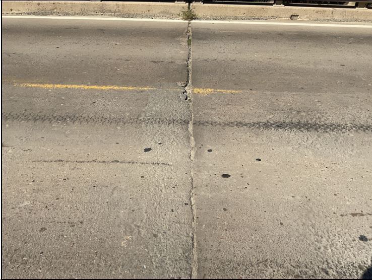
Joint - Bent 2: Spalling of adjacent deck
