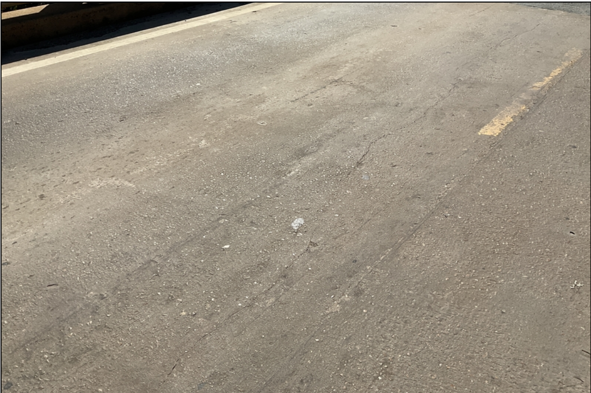
Deck - Span 6 left: Longitudinal crack
