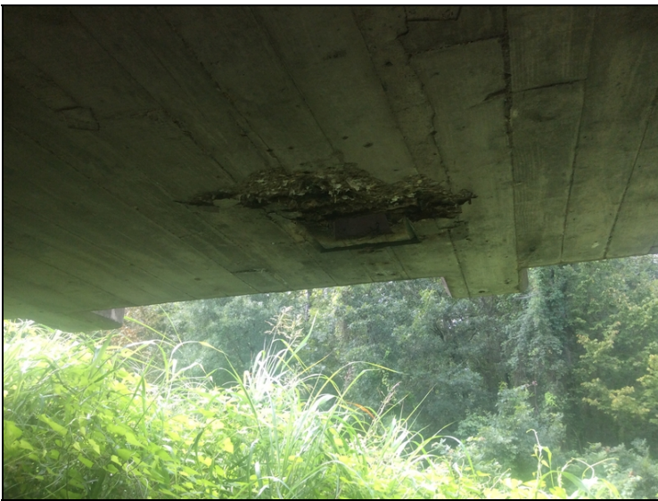
Spall with exposed rebar at soffit drain opening span 1 left side .
