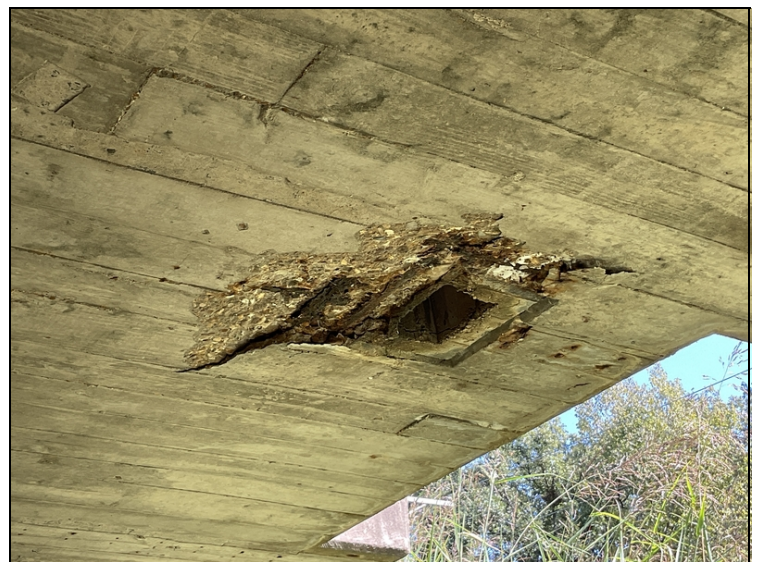
Soffit - Span 1 left: Rebar exposed
