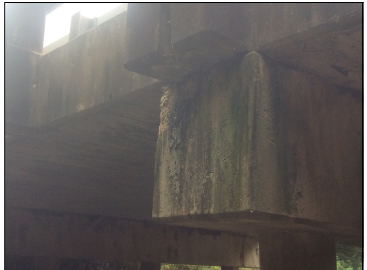
Bent 3 cap right end has small spall .
