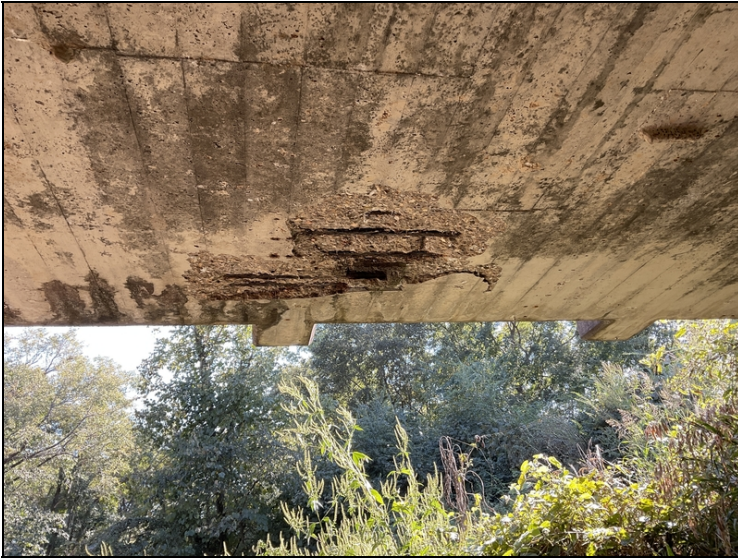
Soffit - Span 3 left: Rebar exposed at drain
