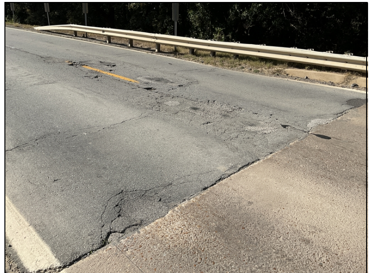
Approach roadway - Bent 4: Deterioration of asphalt wearing surface
