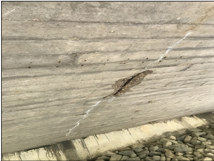
Soffit - Span 1 : Efflorescence and Exposed Rebar
