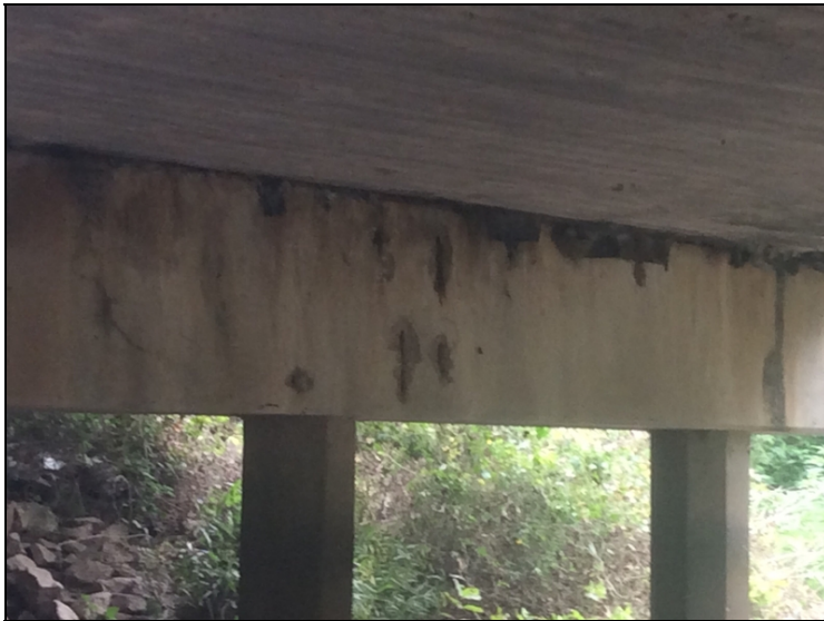
Spalls with exposed rebar on bent 2 cap ahead near mid span .
