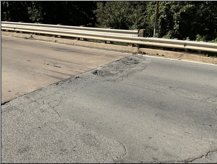
Approach roadway - Bent 1: Deterioration of asphalt wearing surface
