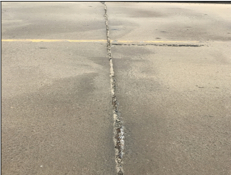
Joint - Bent 2 : Impacted
